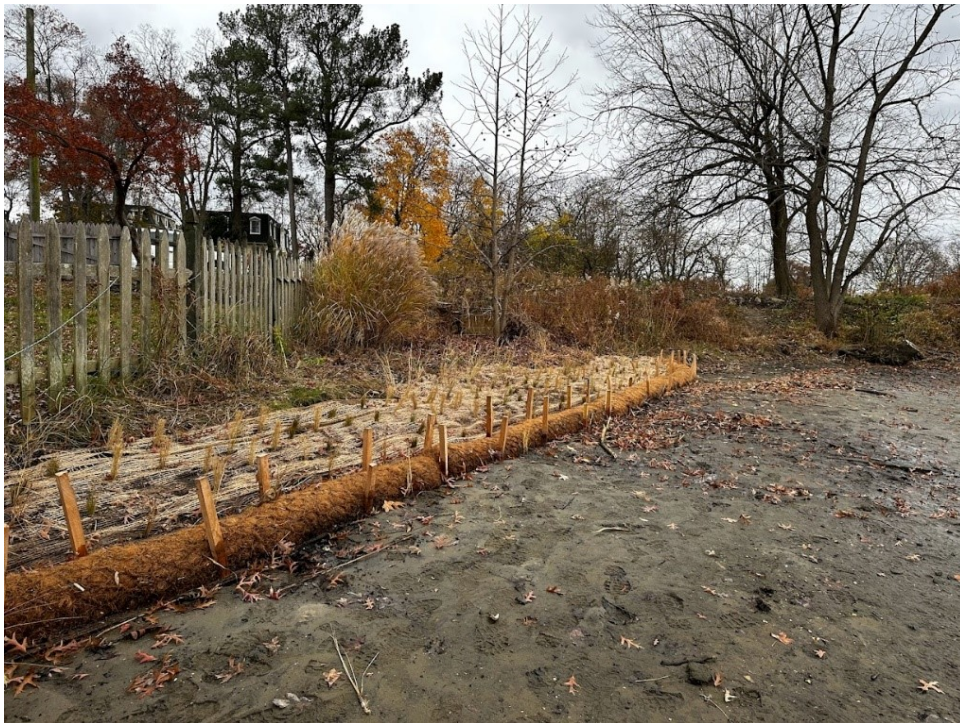
Native planting and coir log installation in Oceanport, NJ
