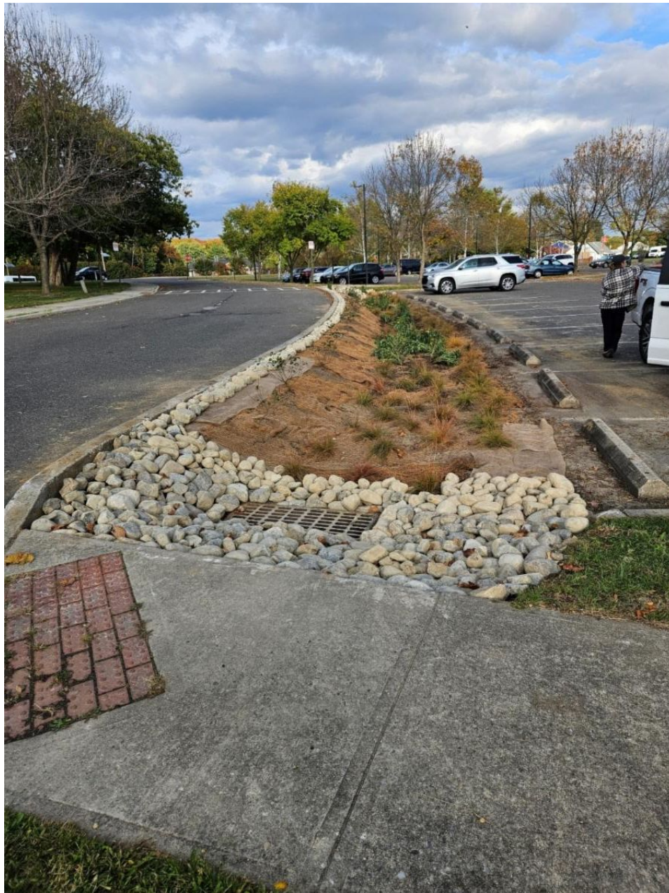
Bioswale planted with native plants at John F. Kennedy Community Center in Willingboro, NJ
