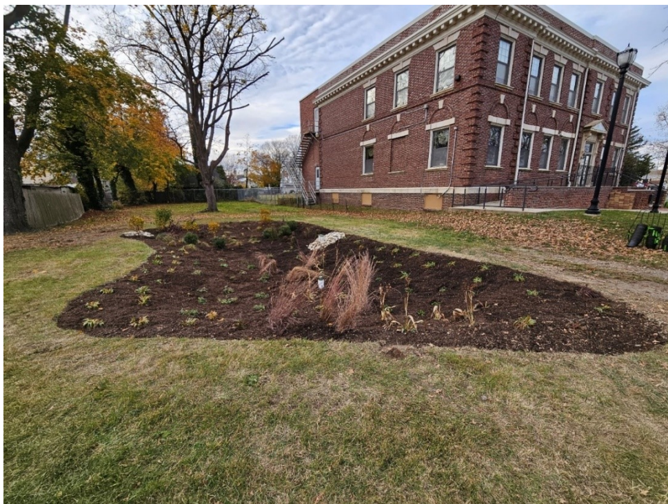
Rain garden installed at Vineland Historical Society in Vineland, NJ
