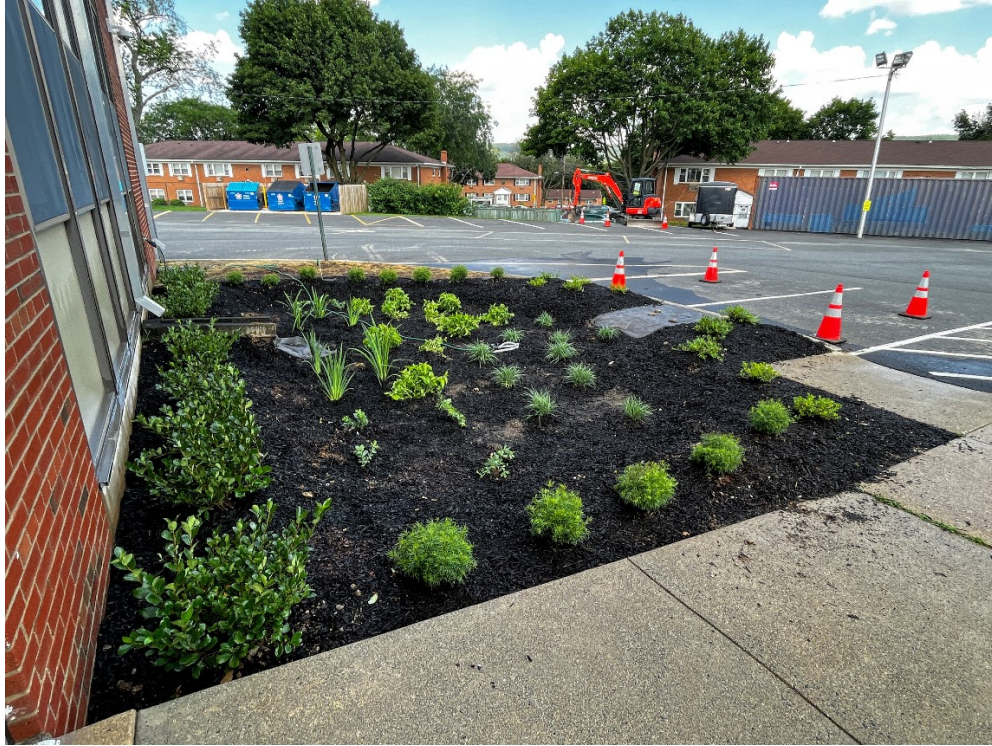
Rain garden installed at Hackettstown High School in Hackettstown, NJ
