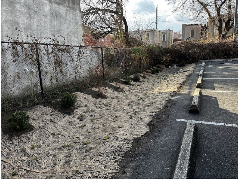
Completed bioswale at Heart of Camden in Camden, NJ
