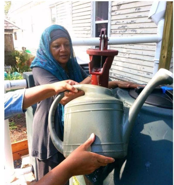
Community Garden Rainwater Harvesting System at 45 Lyons Avenue
