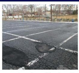
Sections of parking spaces can be replaced with porous asphalt. The porous asphalt will manage stormwater runoff from the parking lot. A preliminary soil assessment suggests that more soil testing would be required before determining the soil's suitability for green infrastructure.
