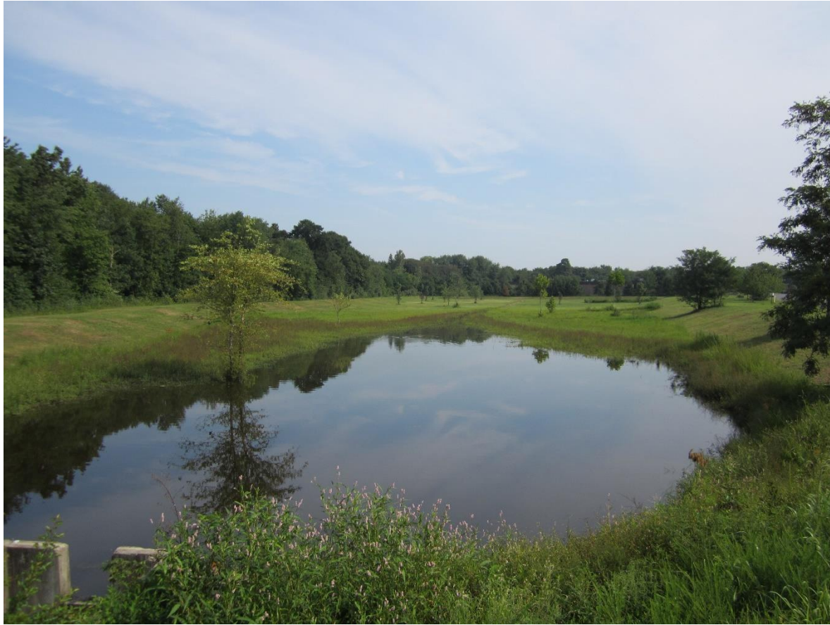
Standing water in detention basin
