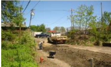
The berm is the low earthen wall of the swale that is planted with upland plants. The berm defines the edge of the swale and helps maintain the flow of the runoff within the channel of the swale. Photo credit, Pat Rector
