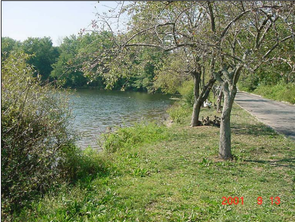
Photo 3 Eroding shoreline along Bee Meadow Pond (Phase II)
