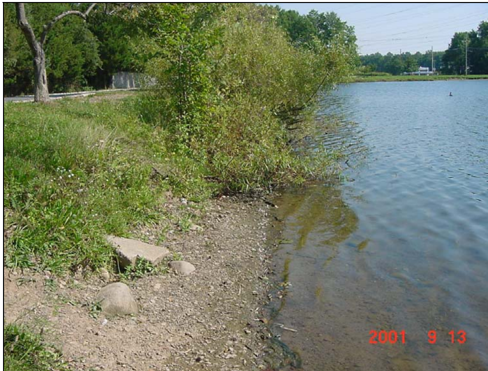
Photo 2 Eroding shoreline along Bee Meadow Pond (Phase II)
