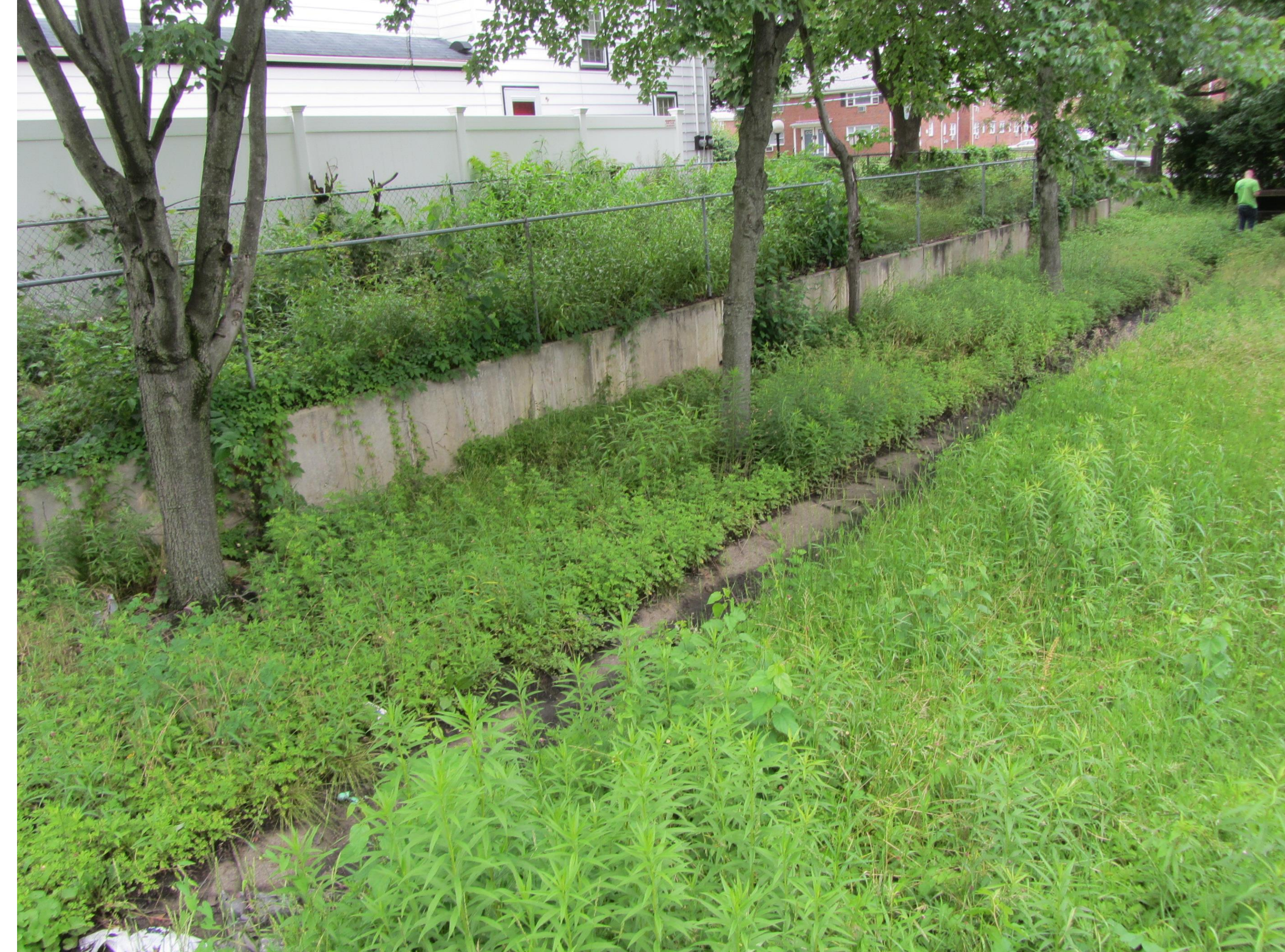
Basin bottom looking north
