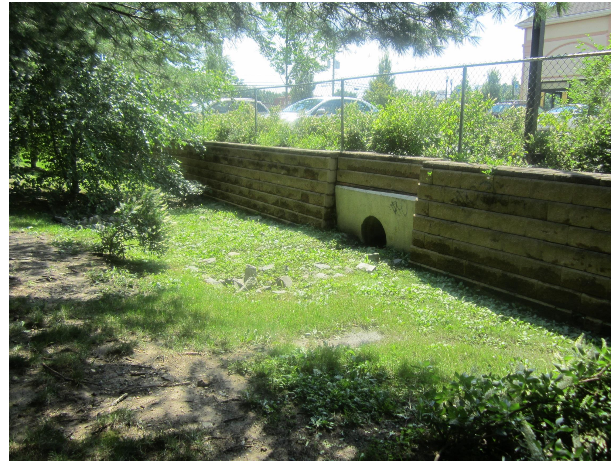
Basin bottom looking southwest
