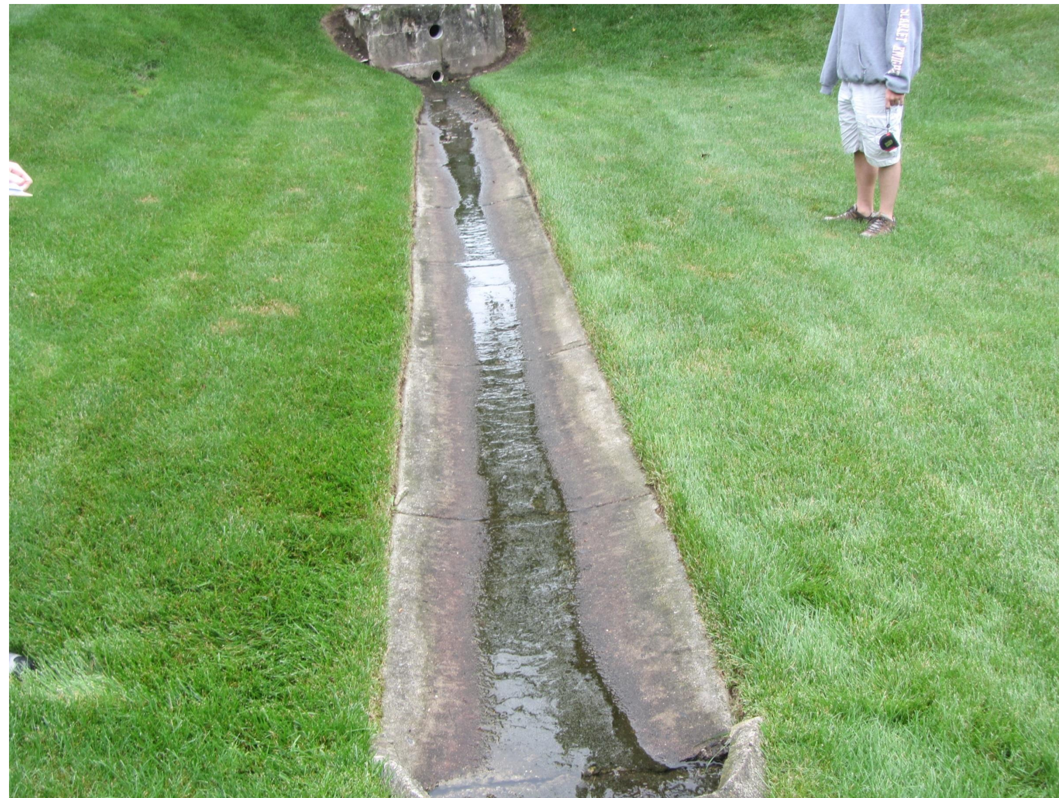
Basin bottom looking west
