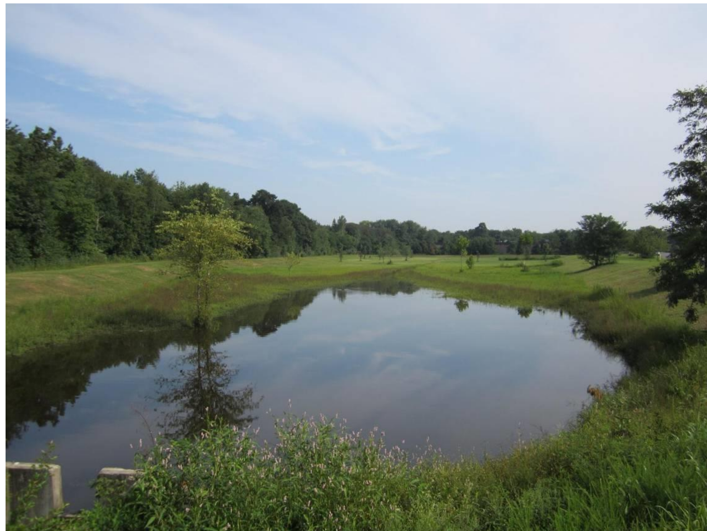
Ponding in front of outlet
