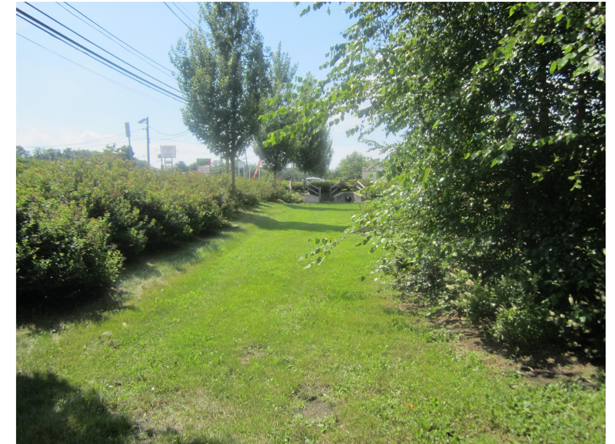
Basin bottom looking west
