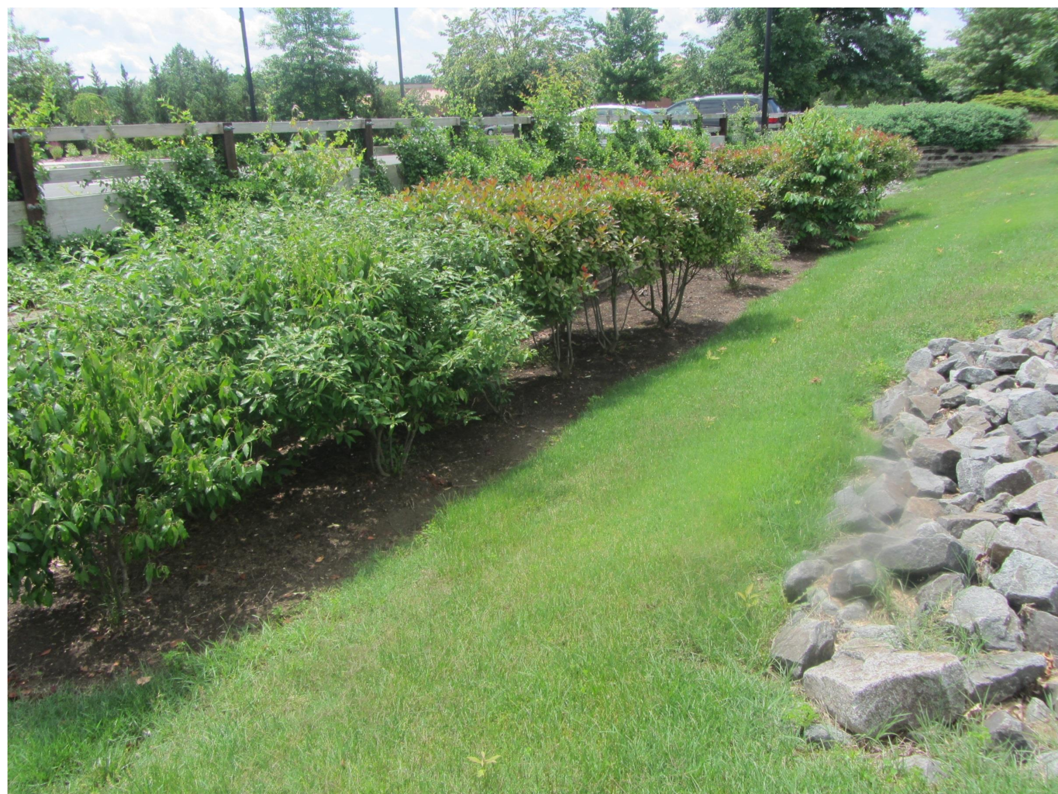
Basin bottom looking west
