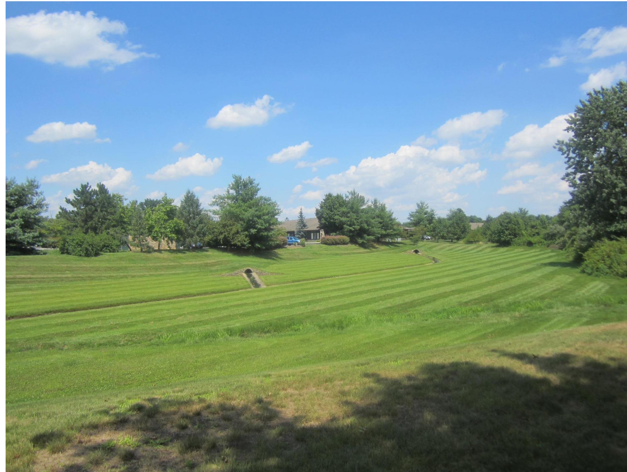
Basin bottom looking northeast
