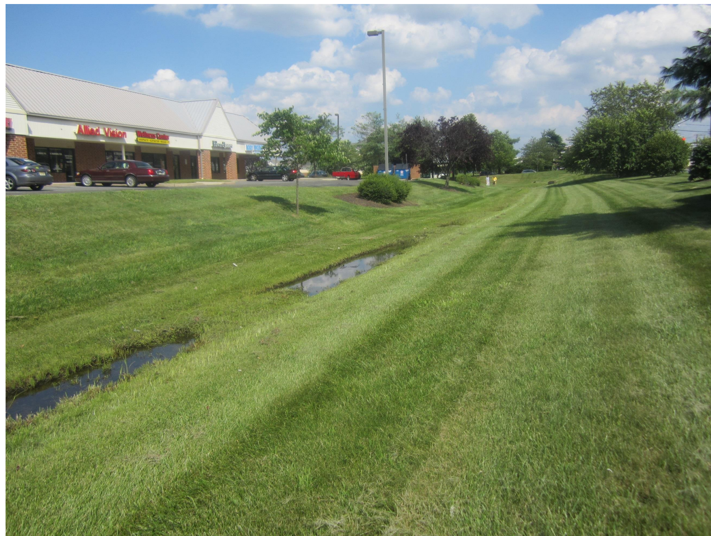
Basin bottom looking east
