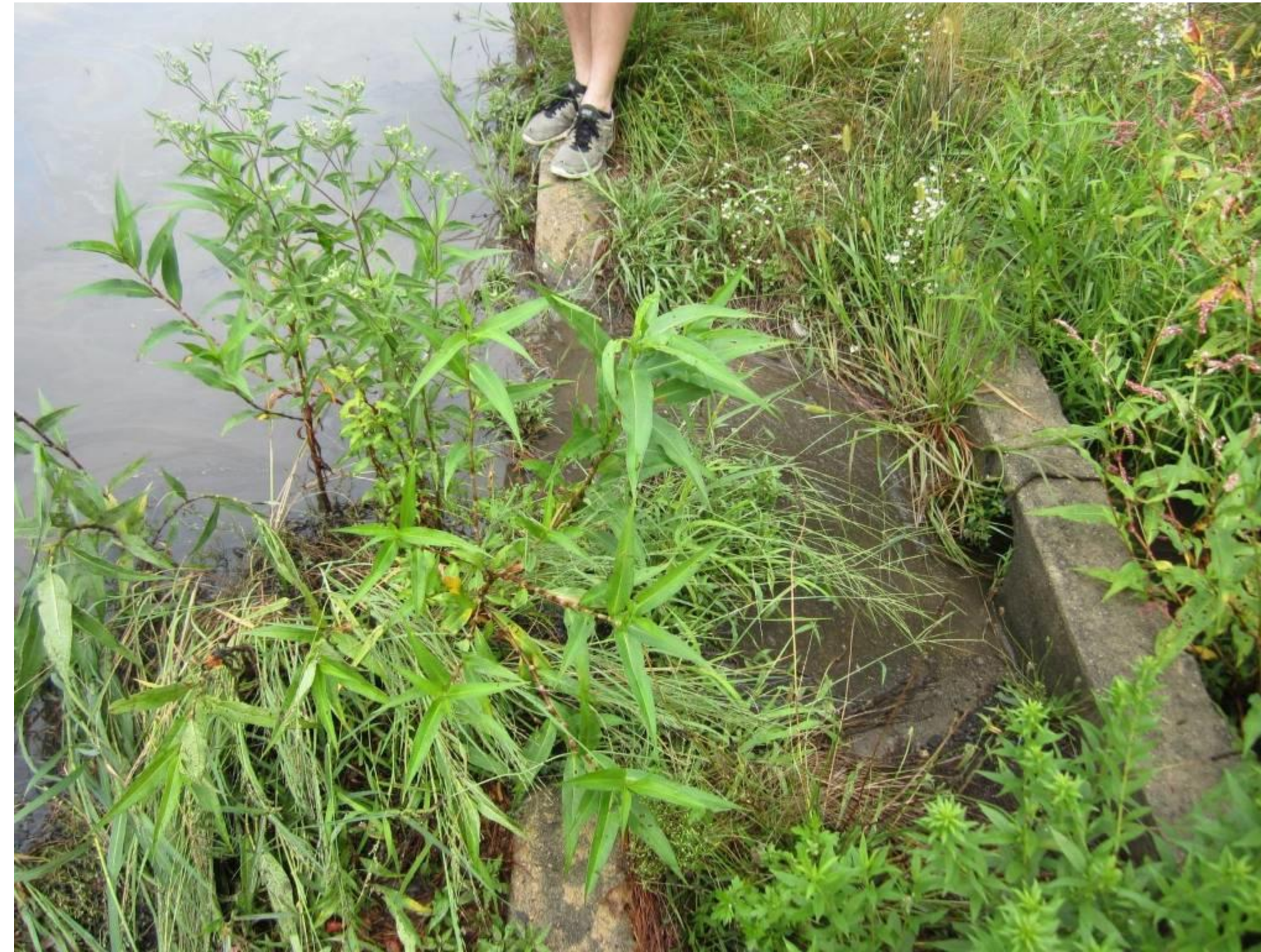
Inlet – curb cut
