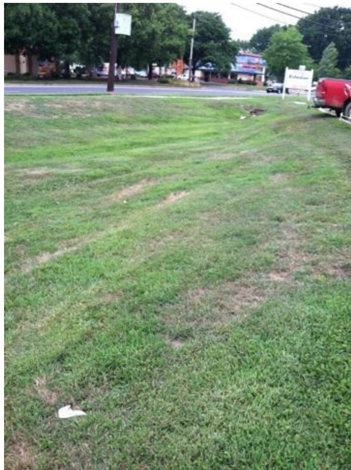
Basin bottom looking north
