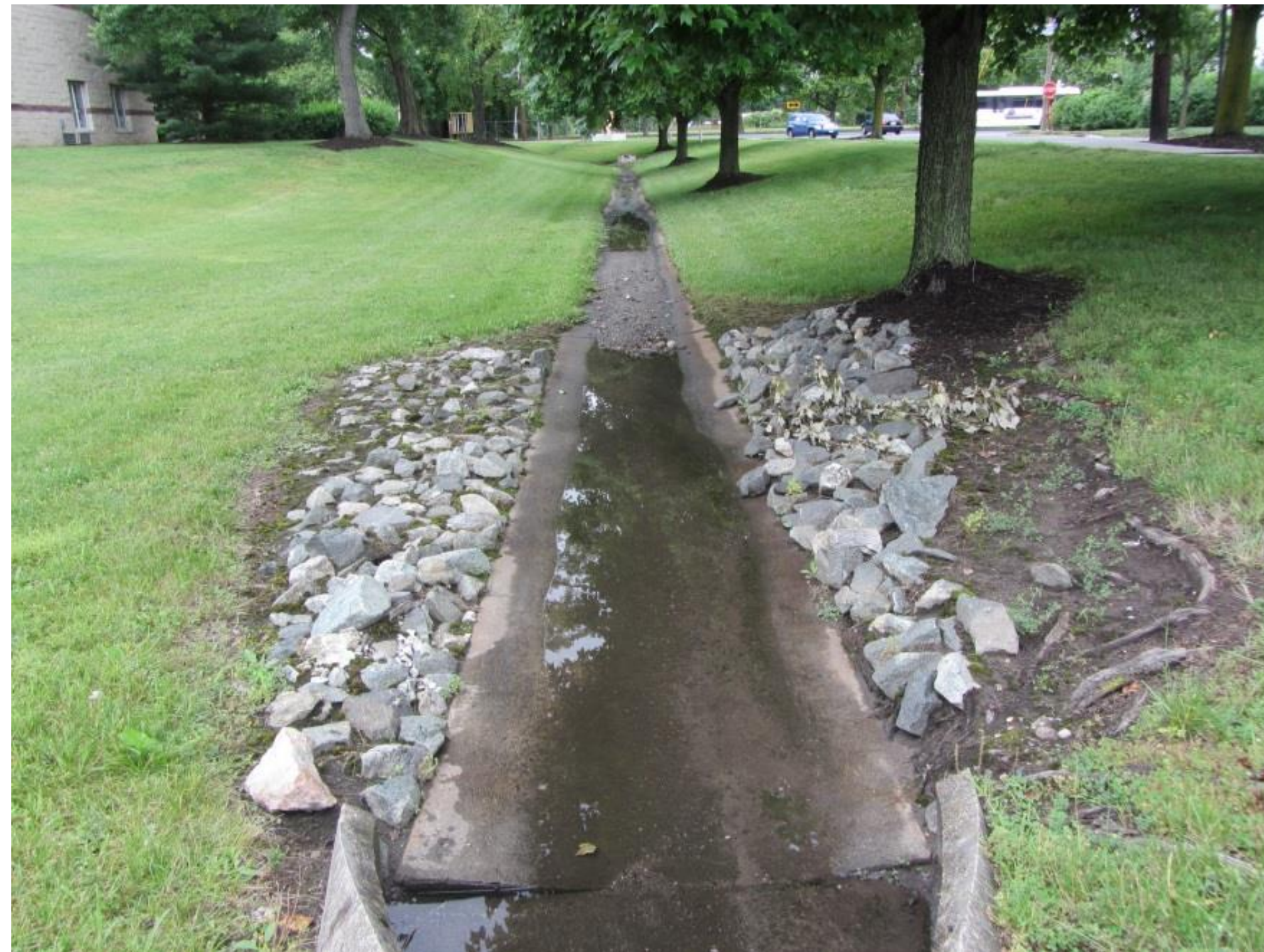
Basin bottom looking northwest
