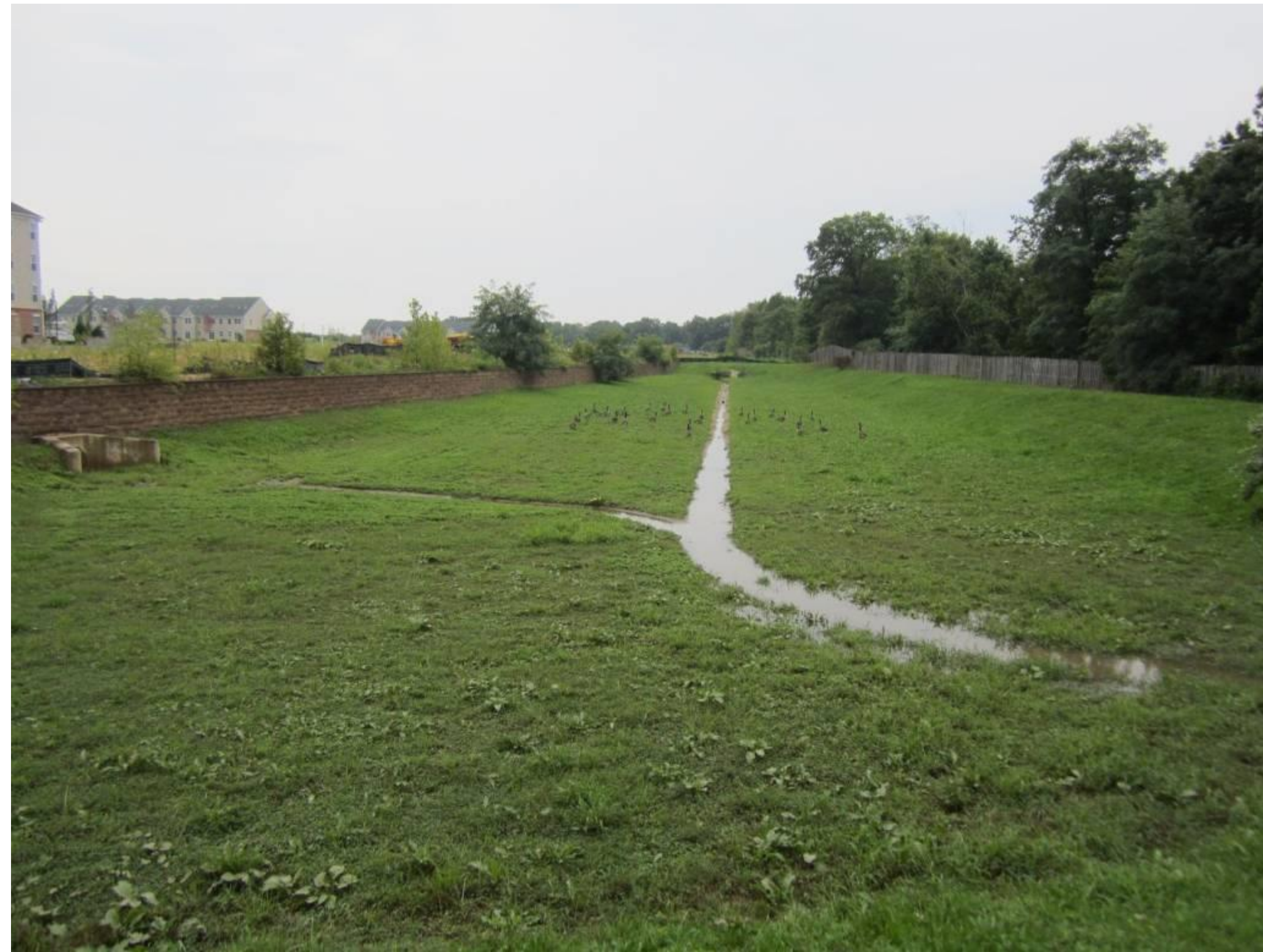
Basin bottom looking southwest
