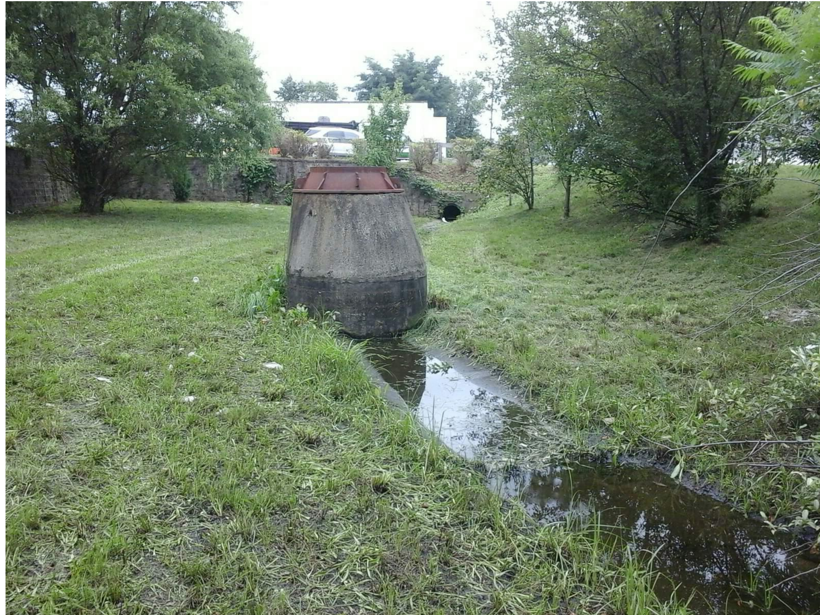
Overview of basin
