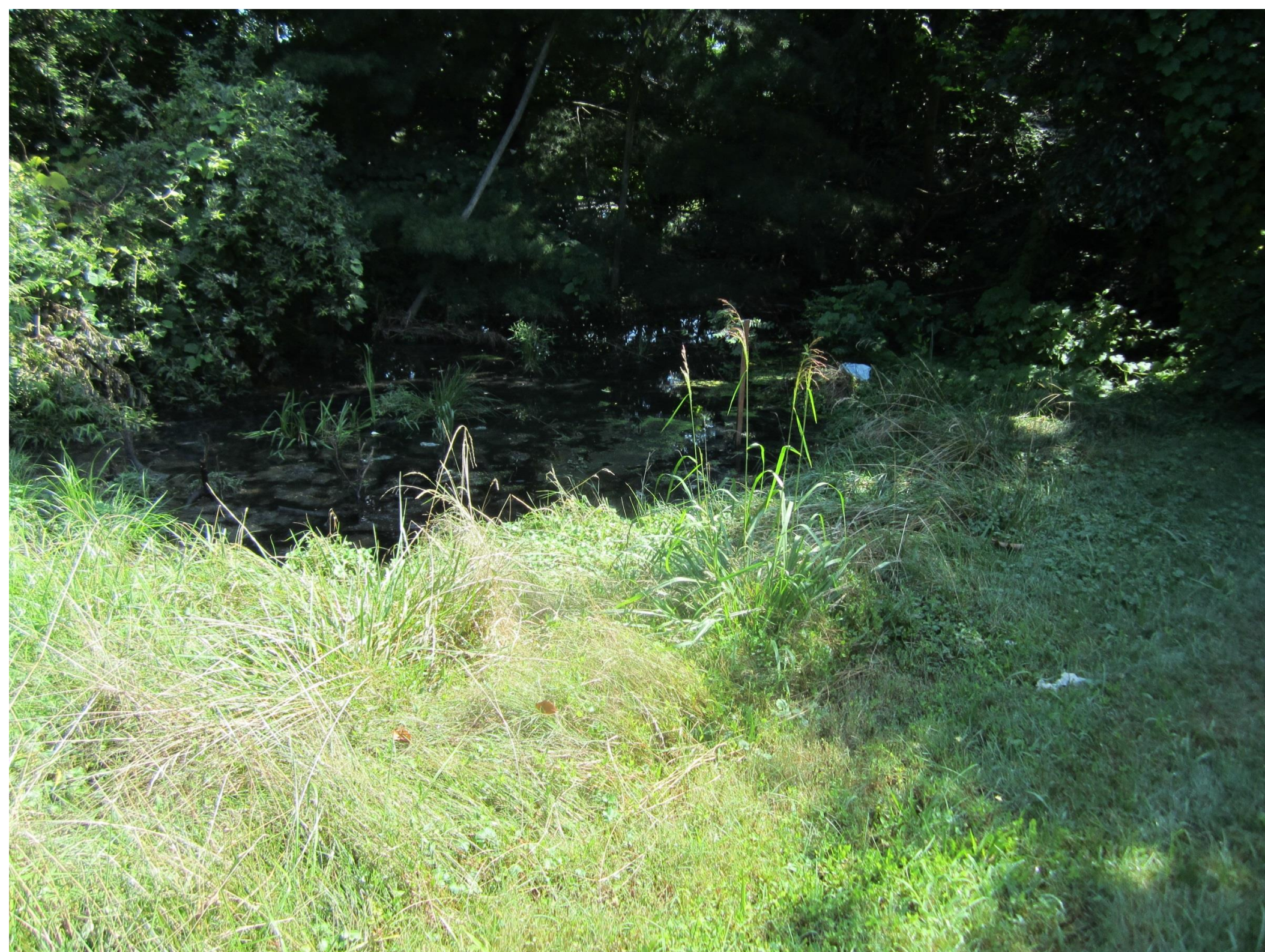
Ponding with algae growth
