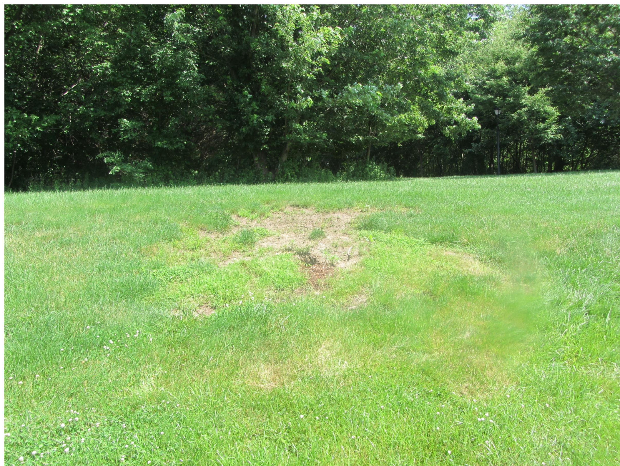
Bare spot on eastern embankment
