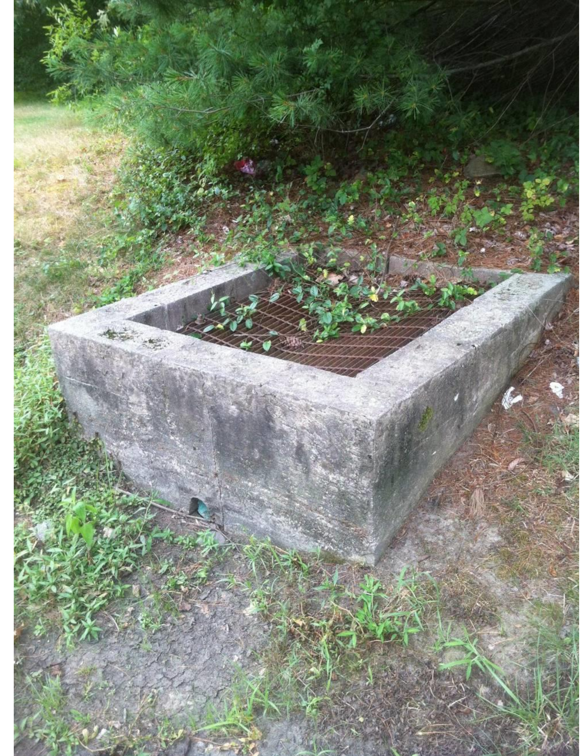
Damaged outlet
