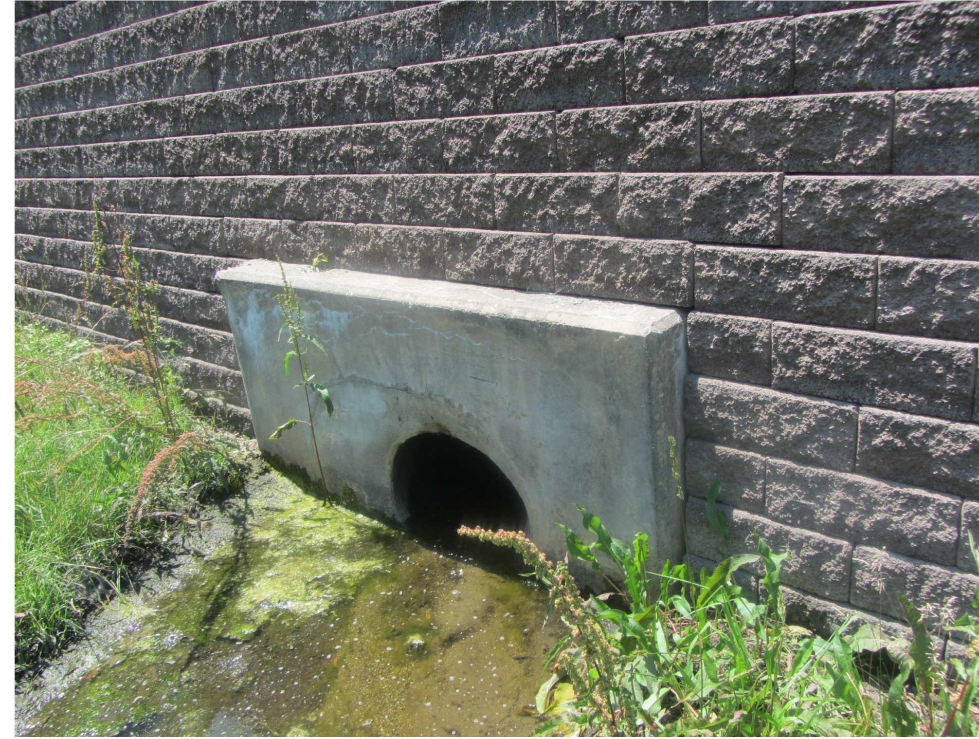
Southern inlet structure
