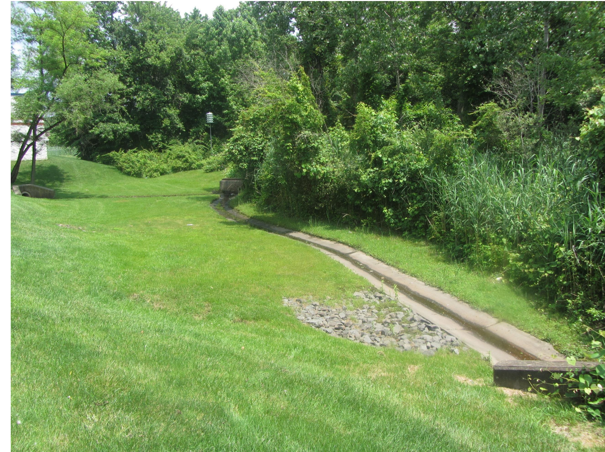
Basin bottom looking northeast
