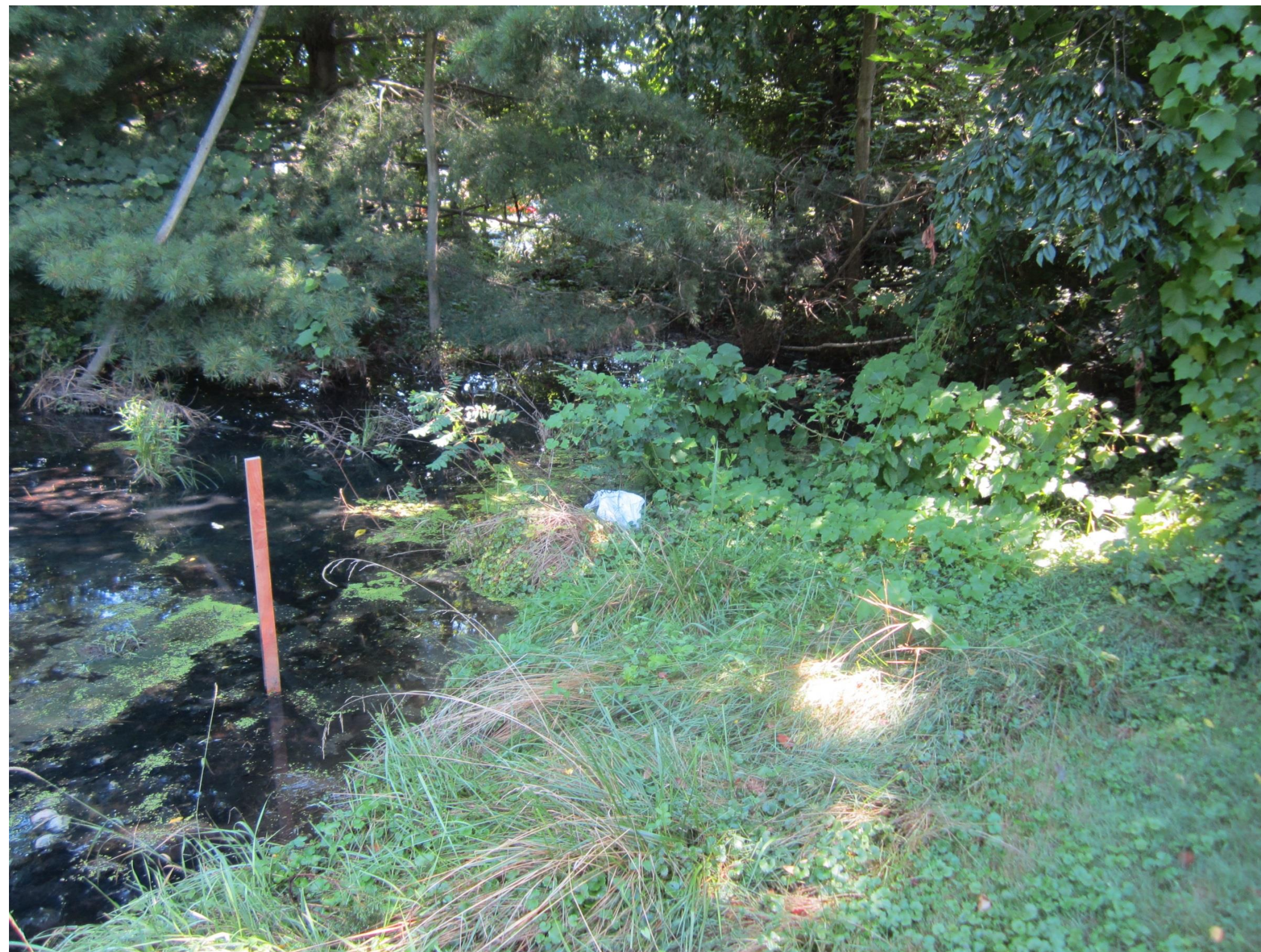
Area where basin discharges to woods
