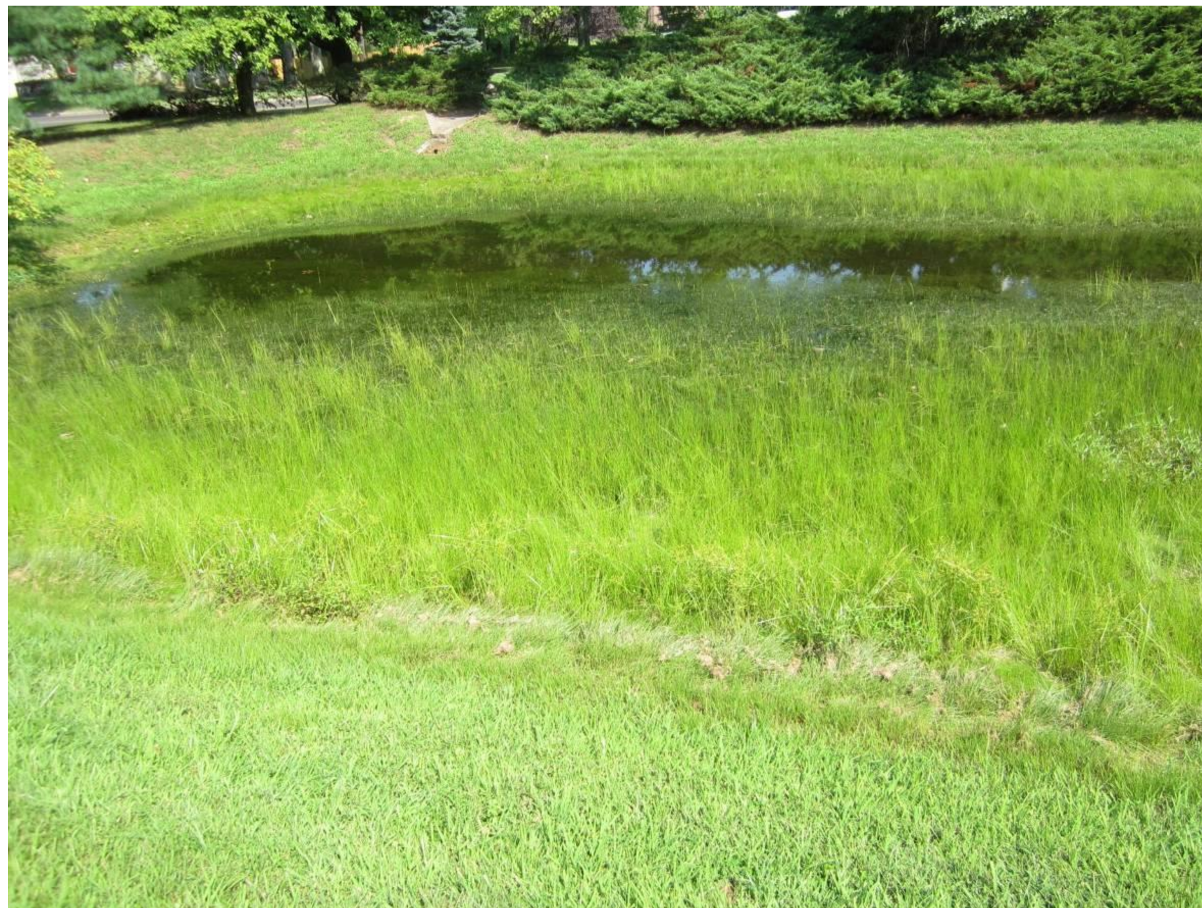
Ponding in basin bottom
