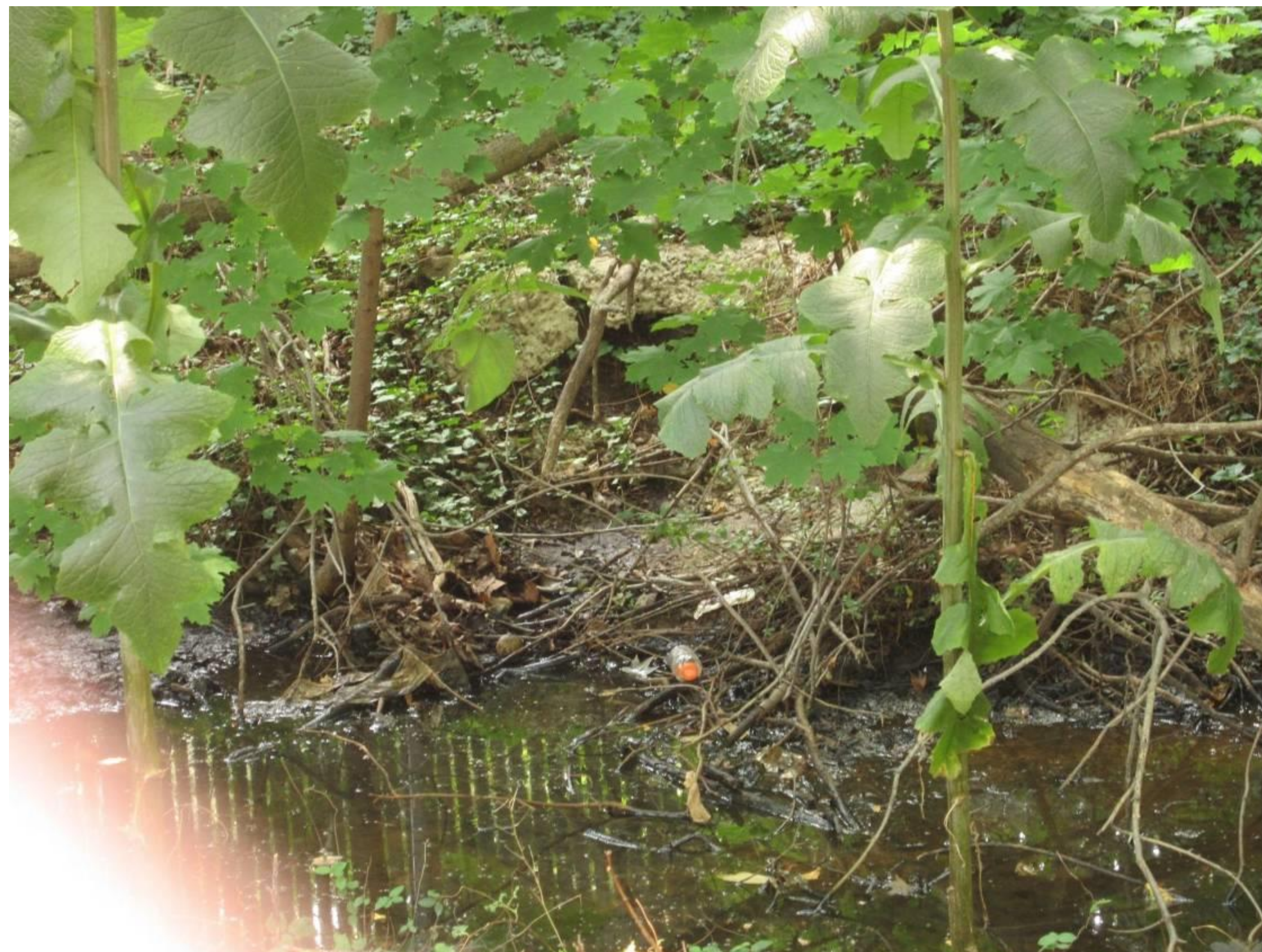
Ponding in basin bottom
