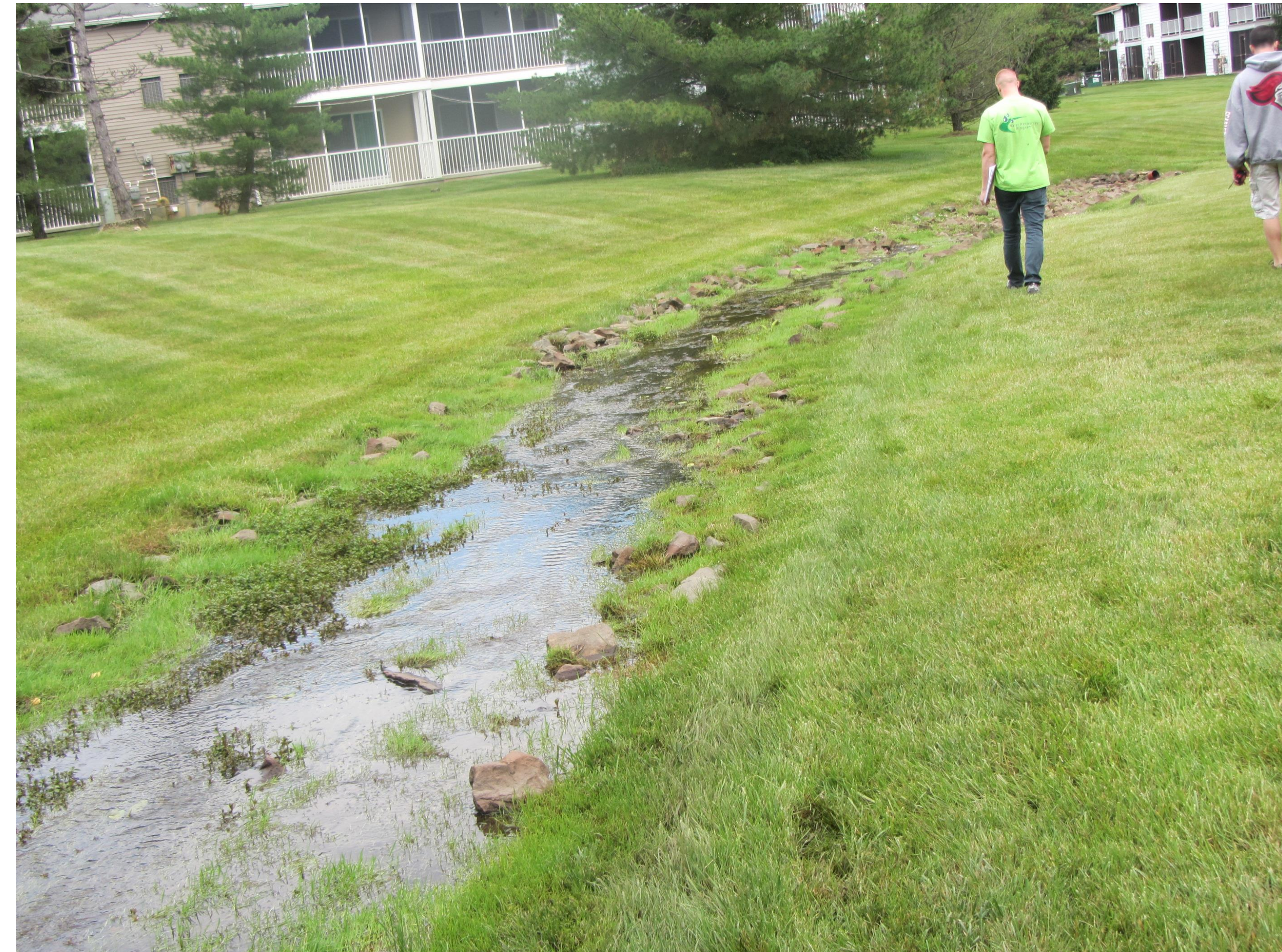
Basin bottom looking north
