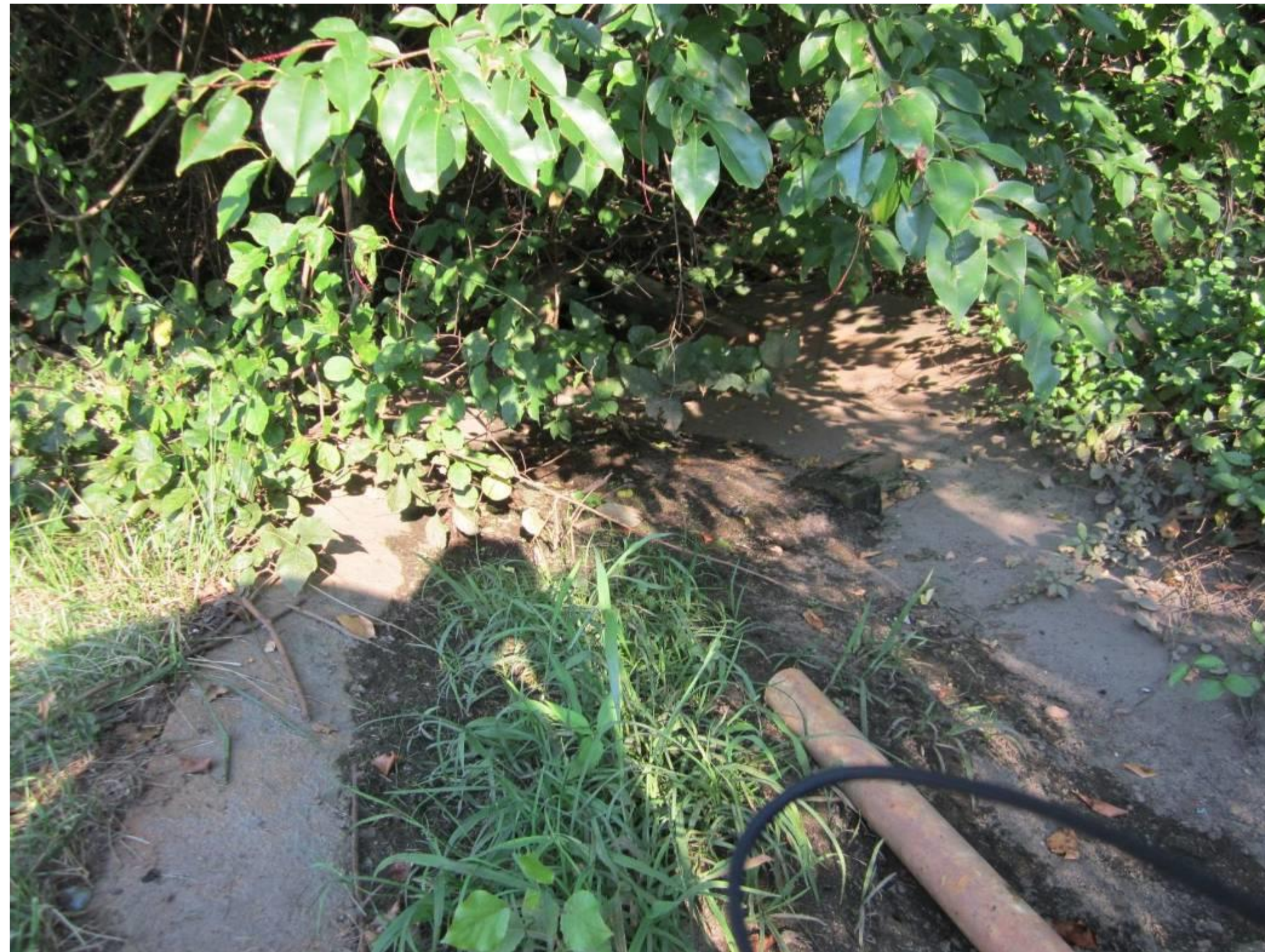
Inlet covered by plant growth
