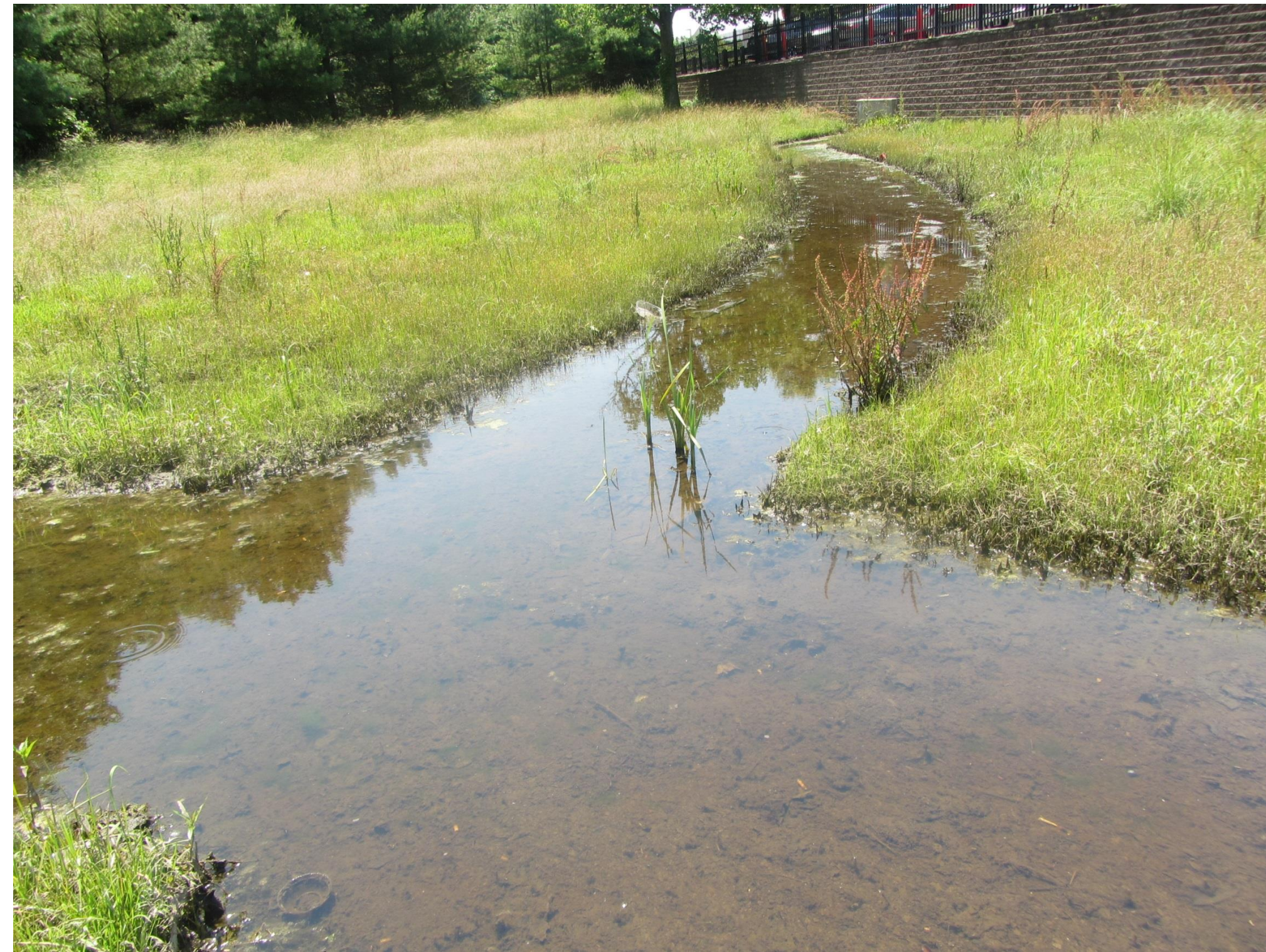
Standing water in low flow channels
