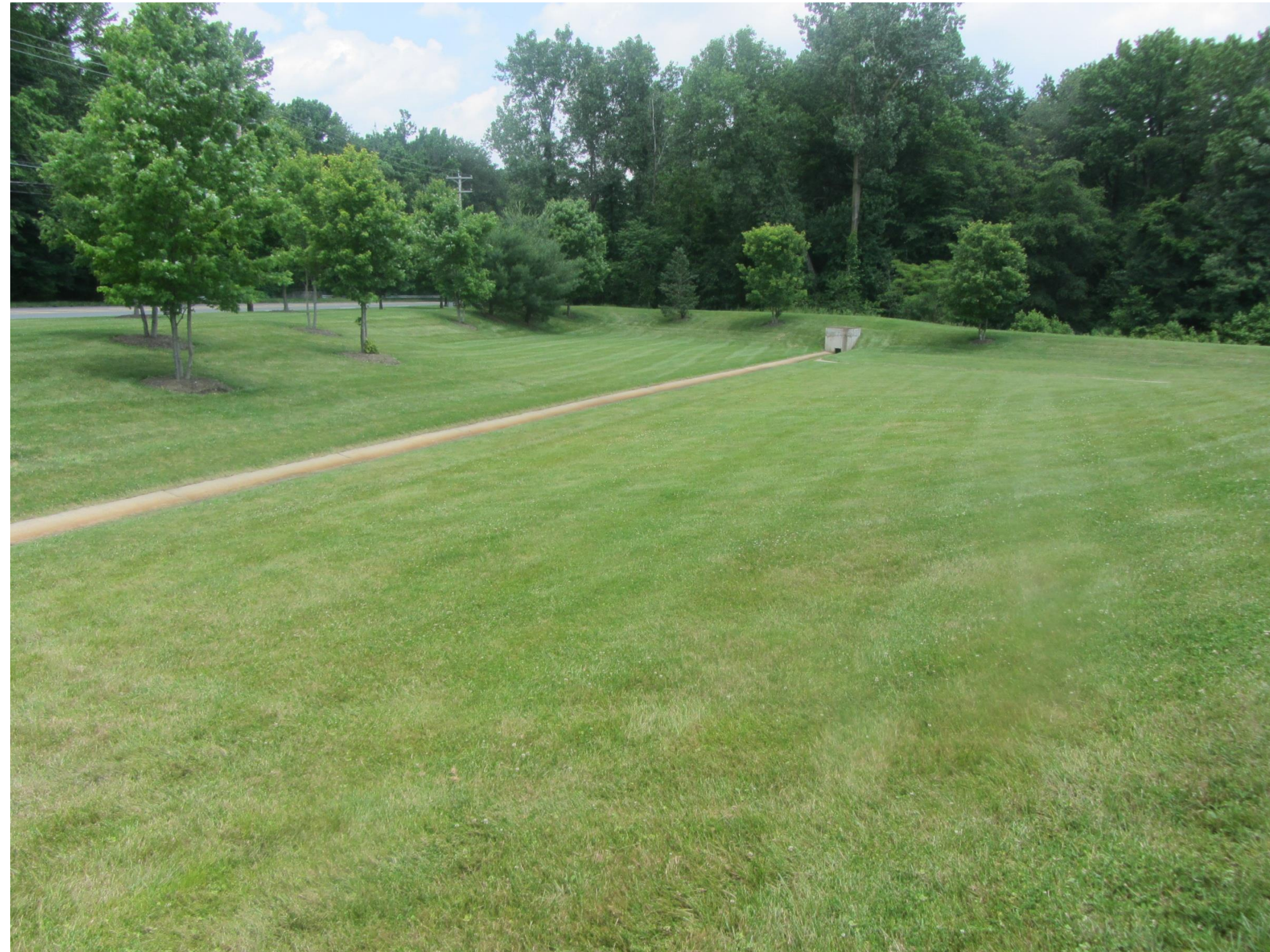
Basin bottom looking north
