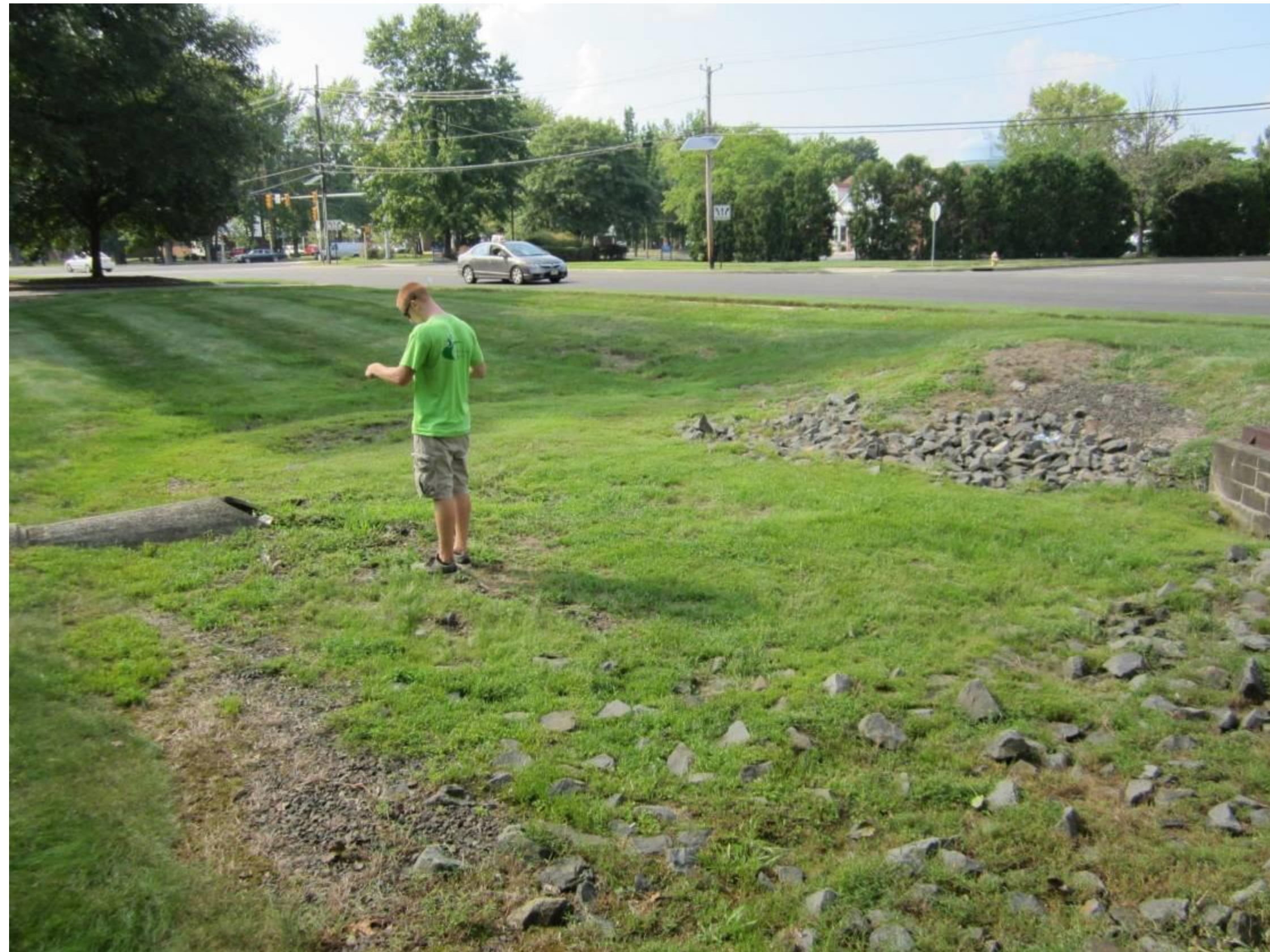
Basin bottom looking west
