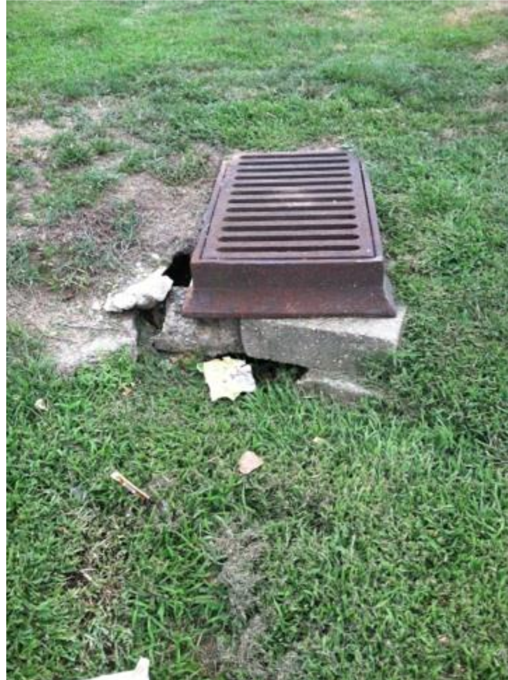
Damaged outlet
