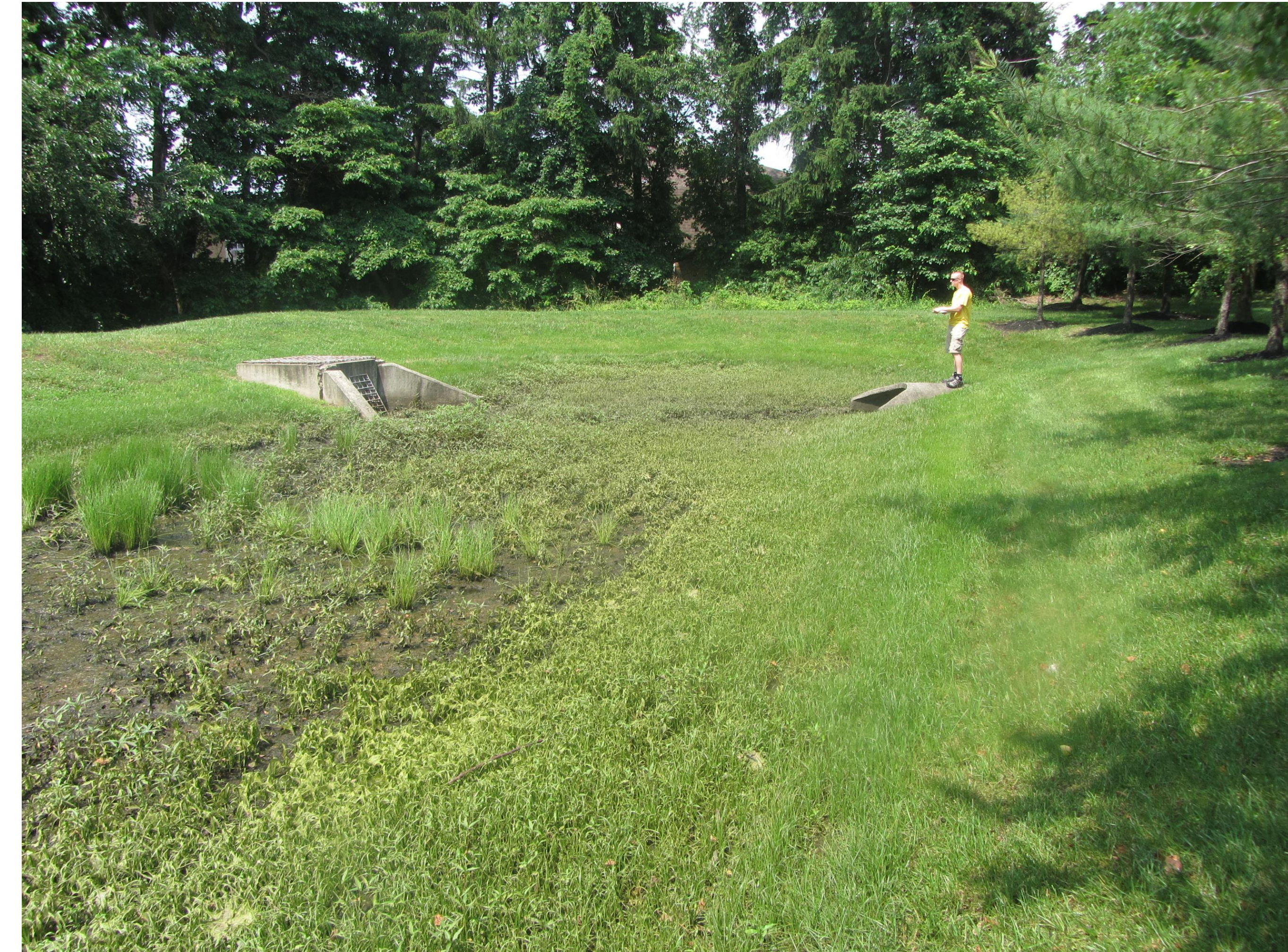
Basin bottom looking northeast
