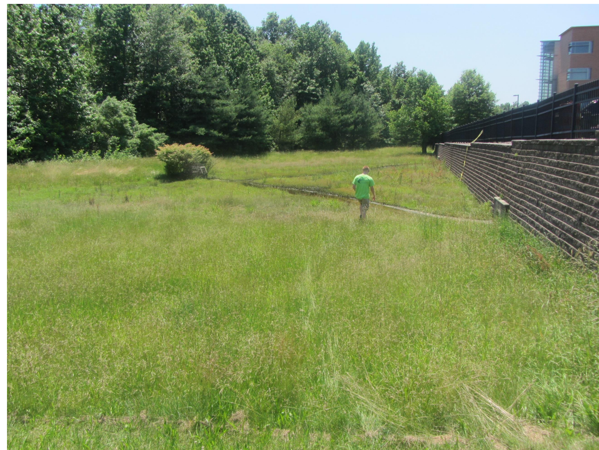
Basin bottom looking southwest
