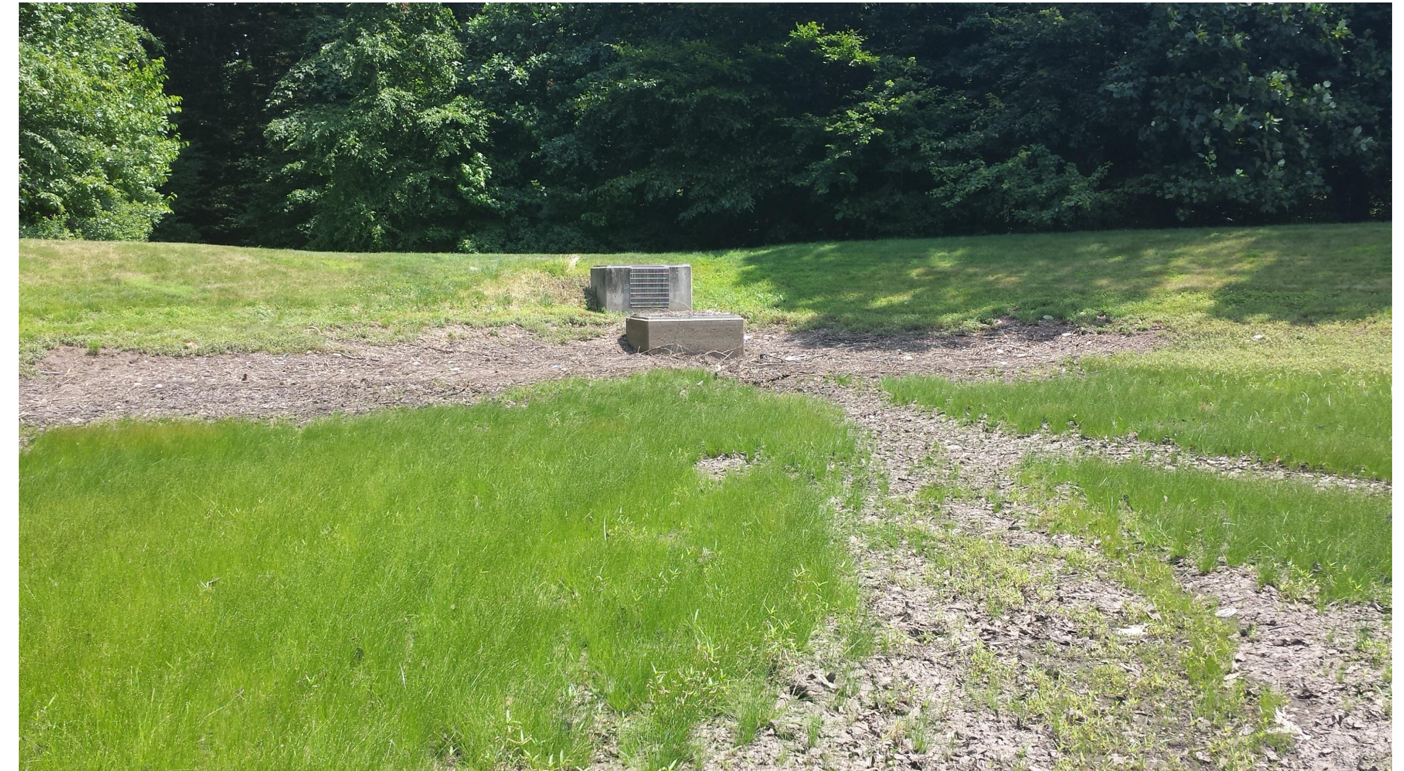
Front view of outlet
