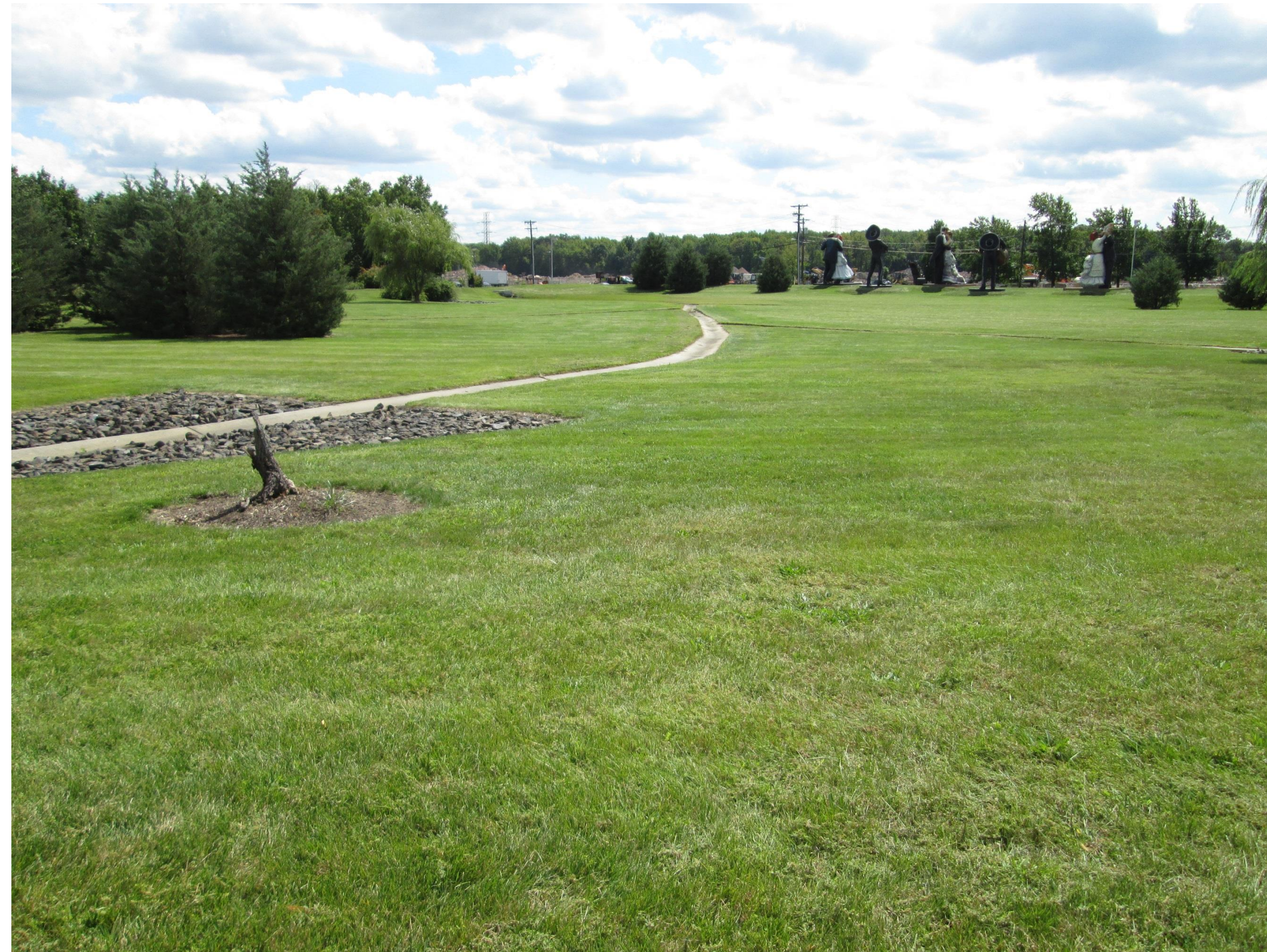
Overview of basin
