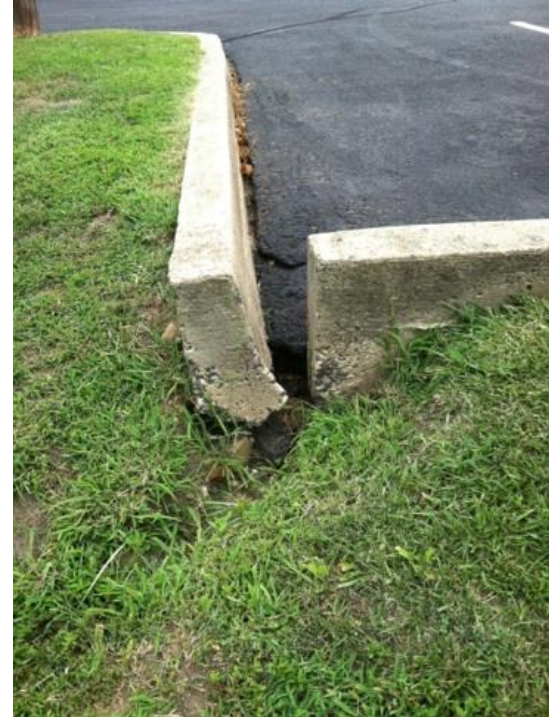
Damaged inlet
