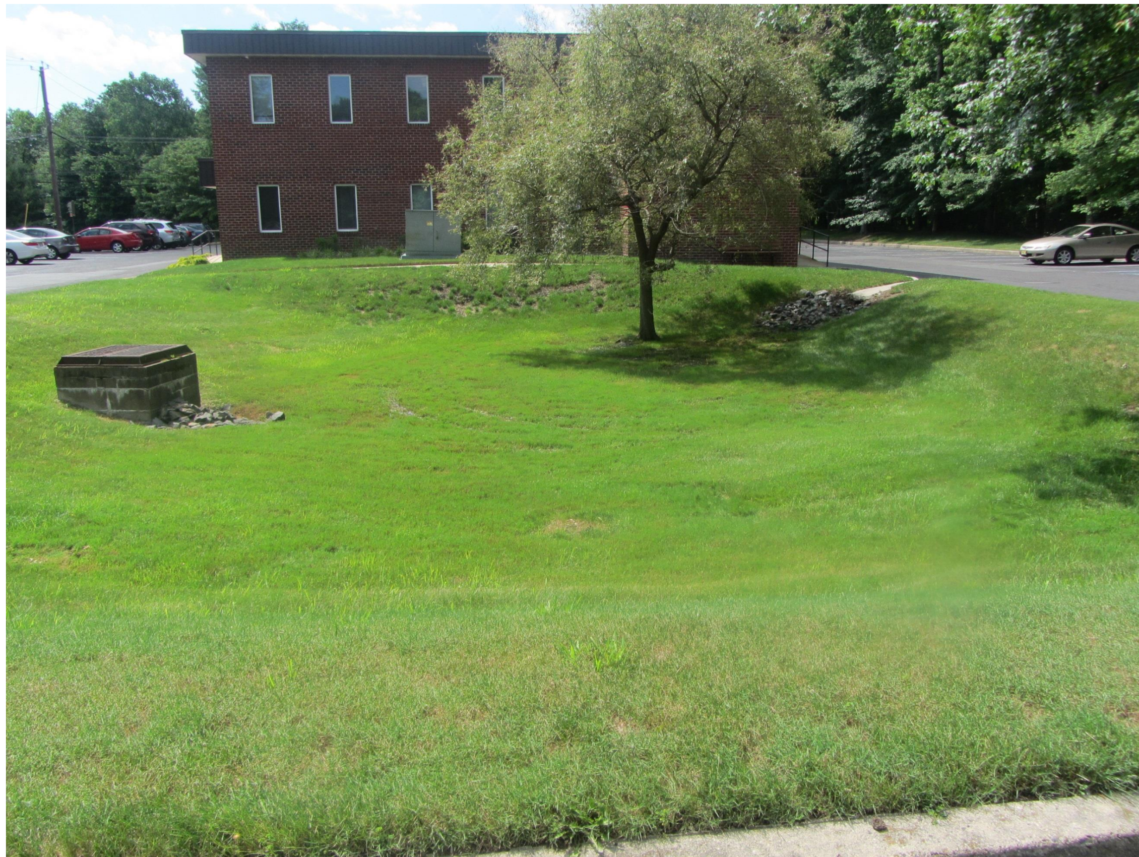
Basin bottom looking northeast
