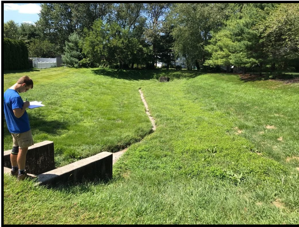
Student interns inspecting Tar Heel Road East detention basin
