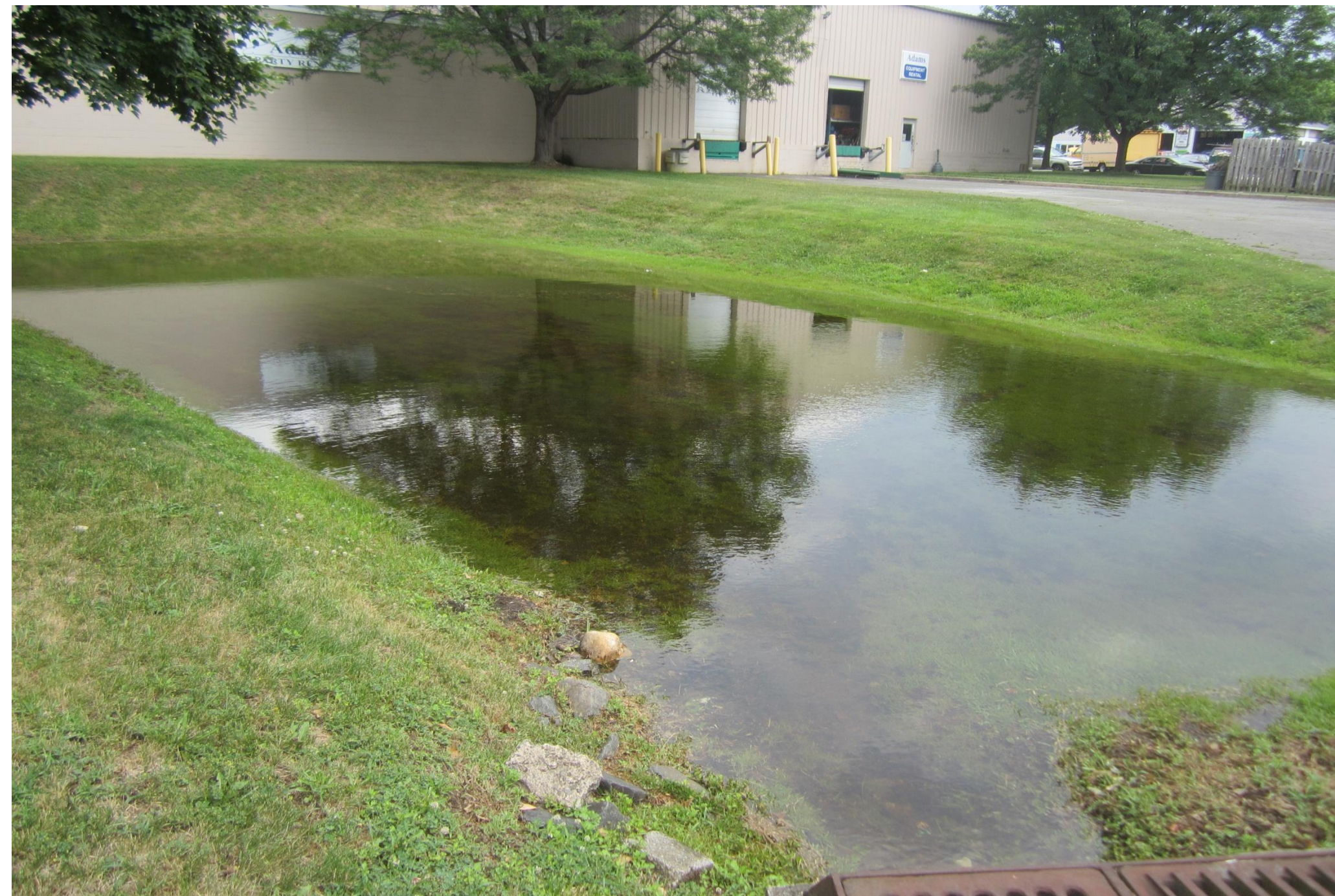
Severe ponding in basin
