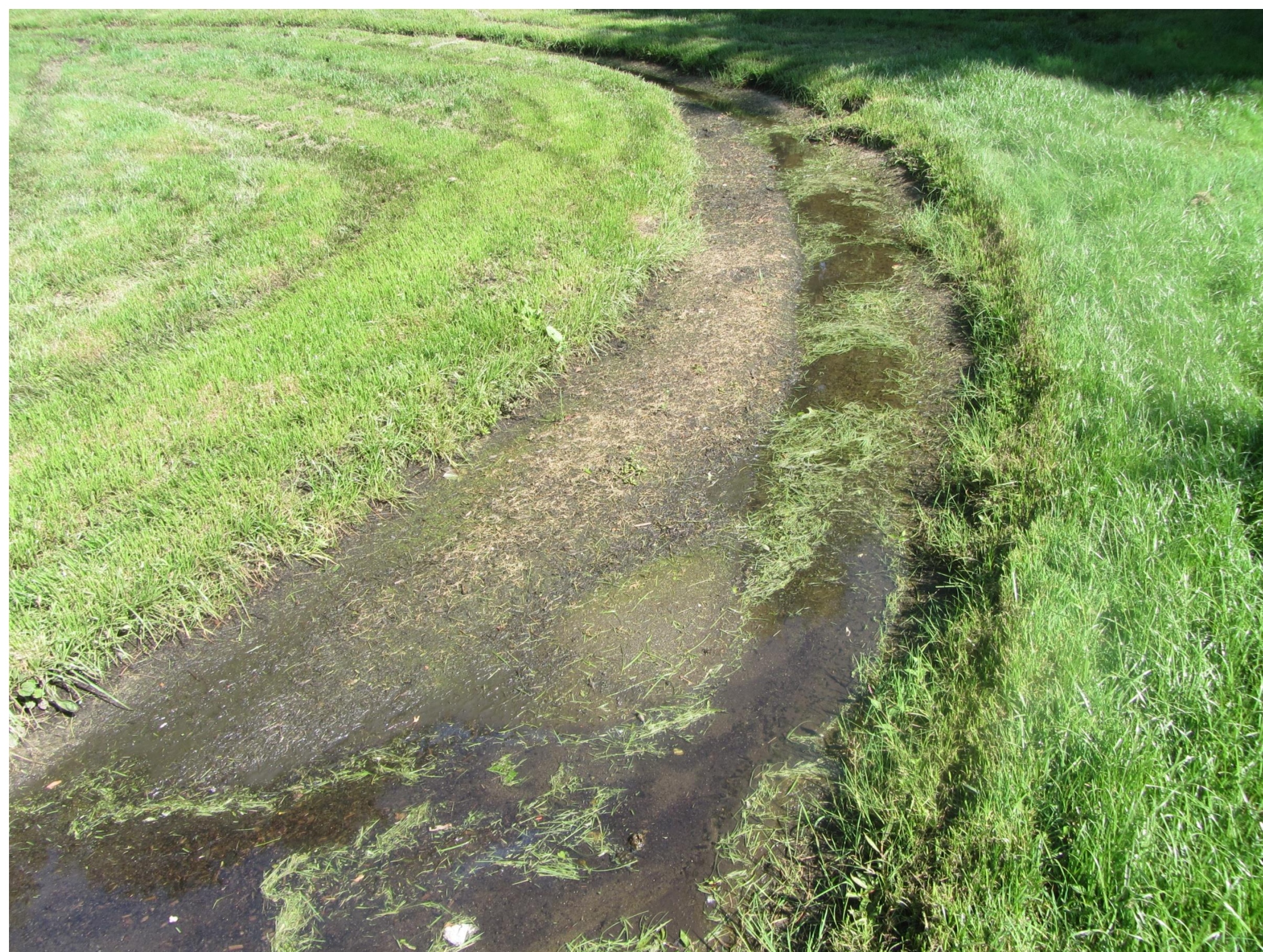
Excess sediment in low flow channel
