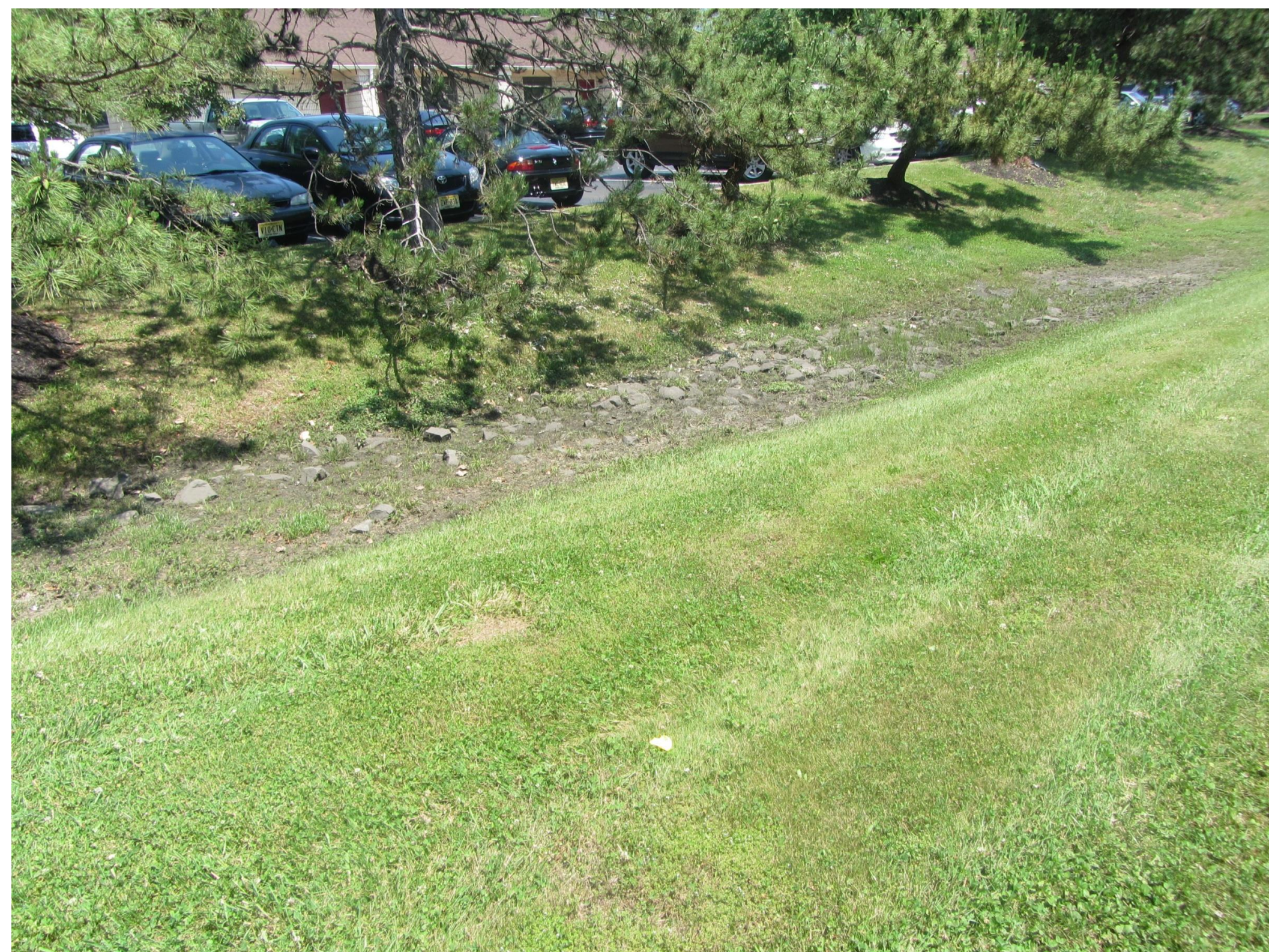
Basin bottom looking north
