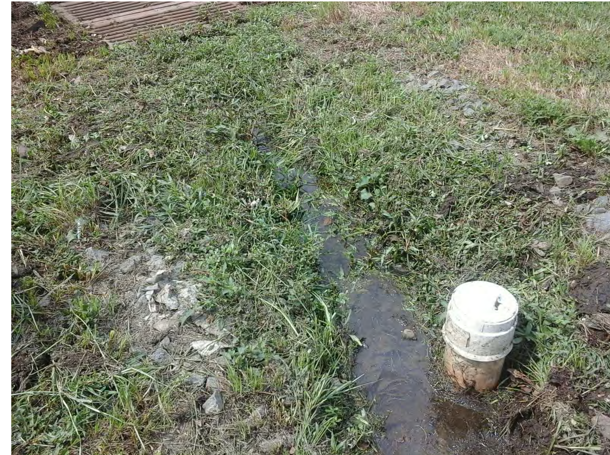
Clean out in low flow channel
