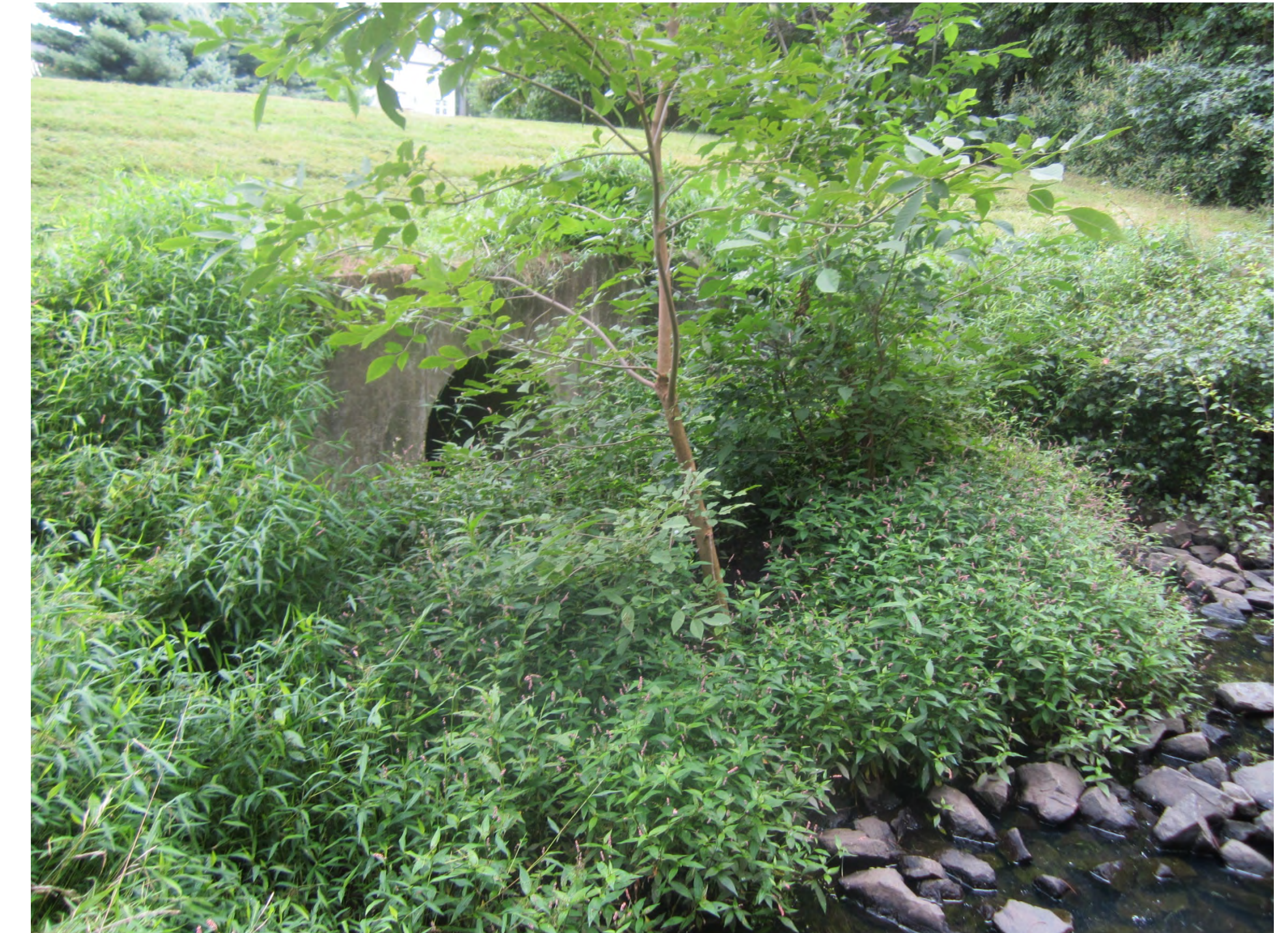
Basin discharge area
