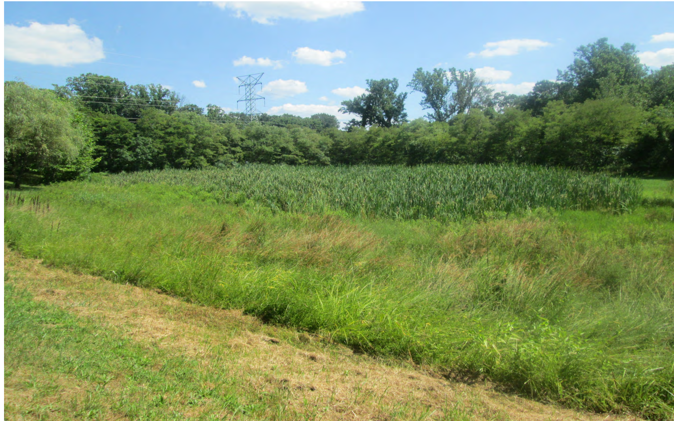
Overview of basin
