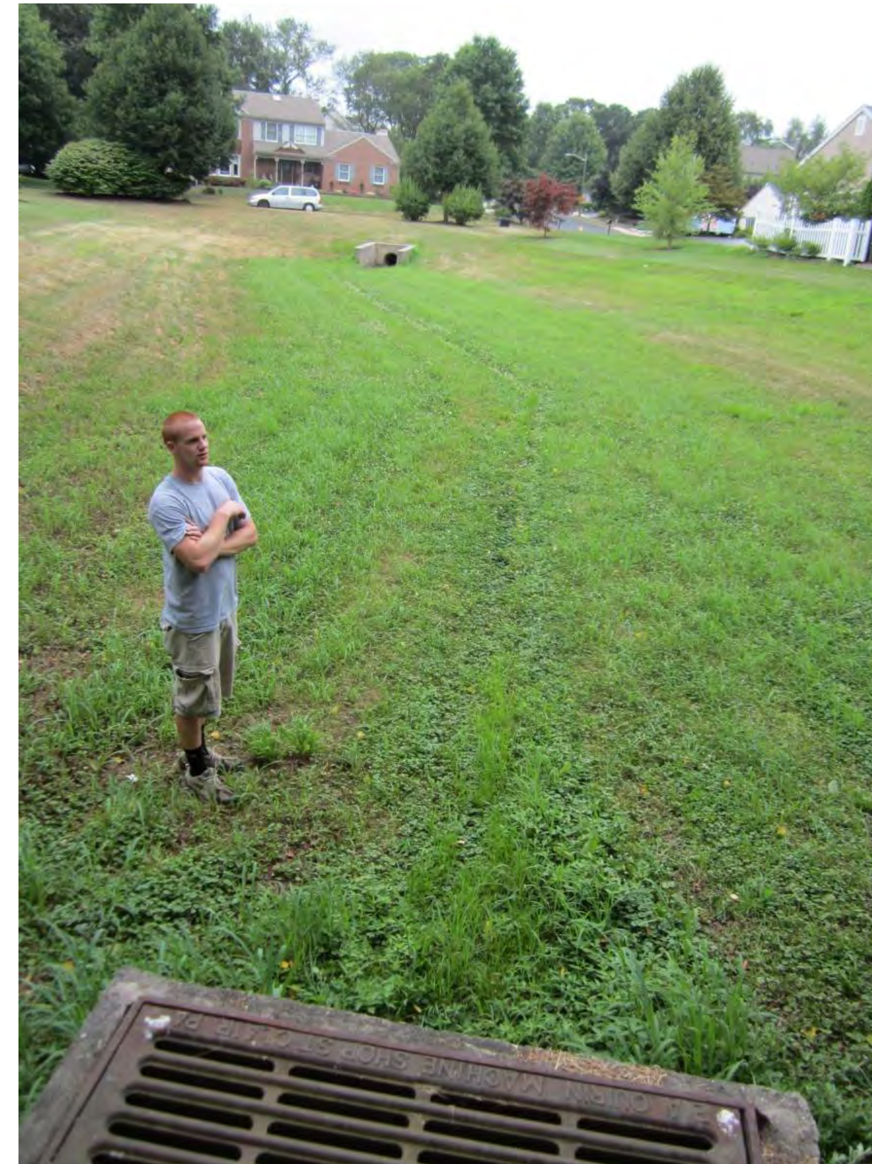
Basin bottom looking east
