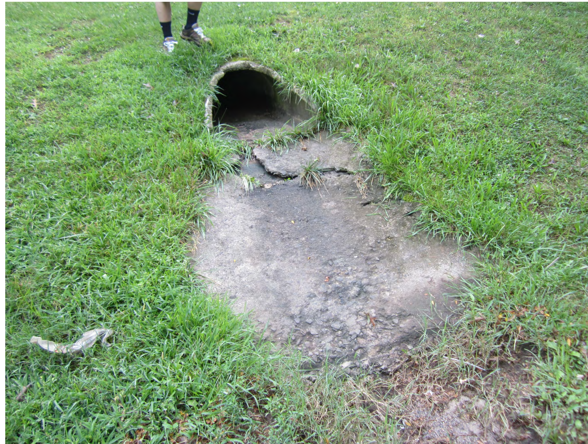
Northeastern inlet structure
