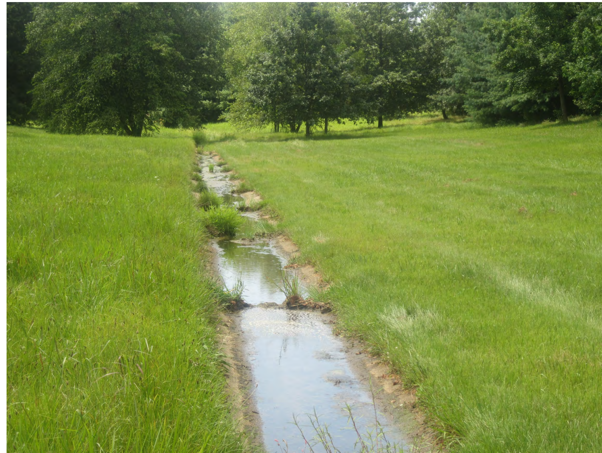
Basin bottom looking northwest
