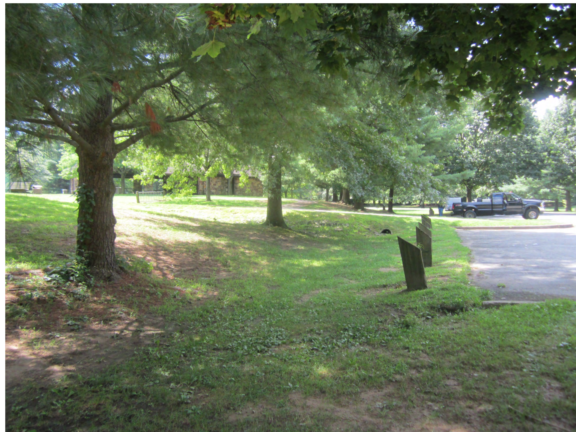
Swale that conveys two inlets to basin
