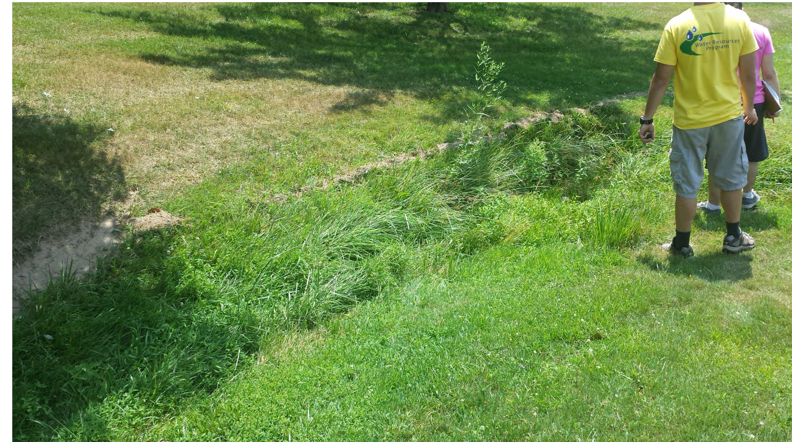
Swale feature lading to basin
