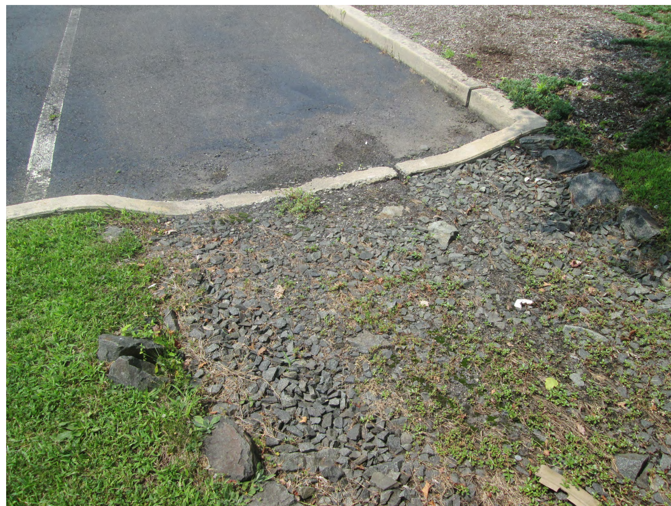
Curb-cut leading to basin
