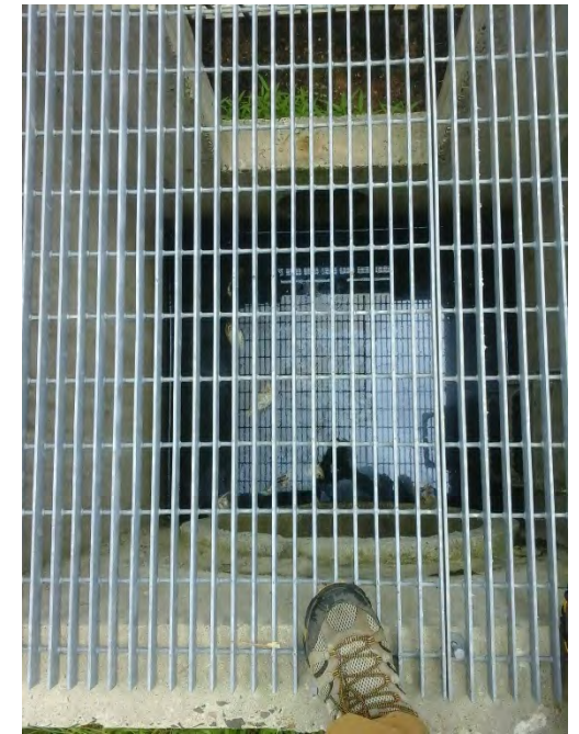
Fish in outlet structure
