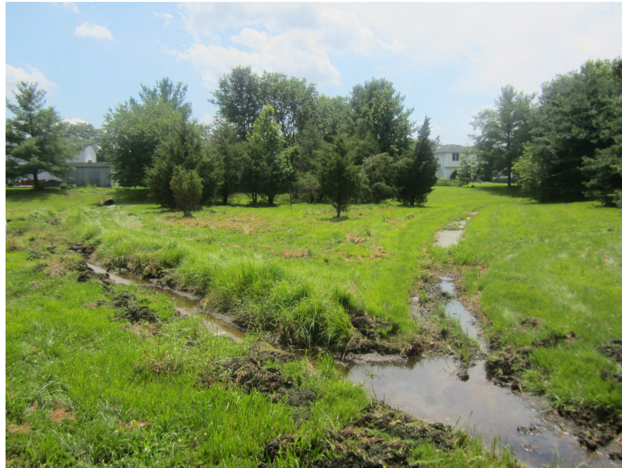
Basin bottom looking east
