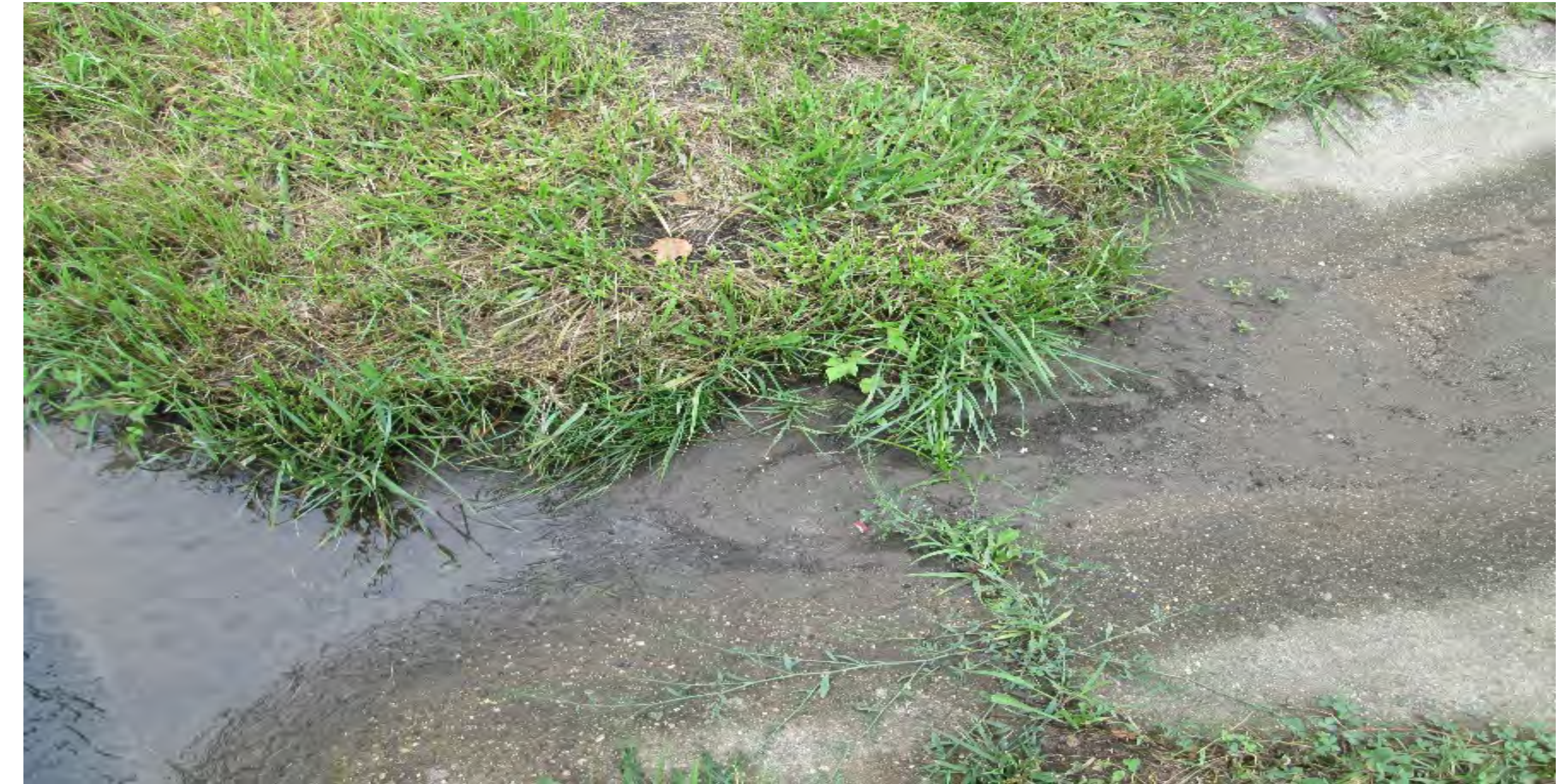
Low flow channel
