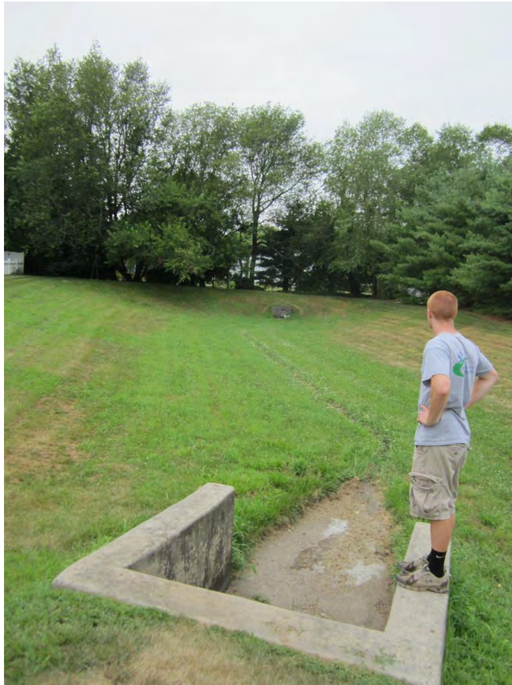
Basin bottom looking west
