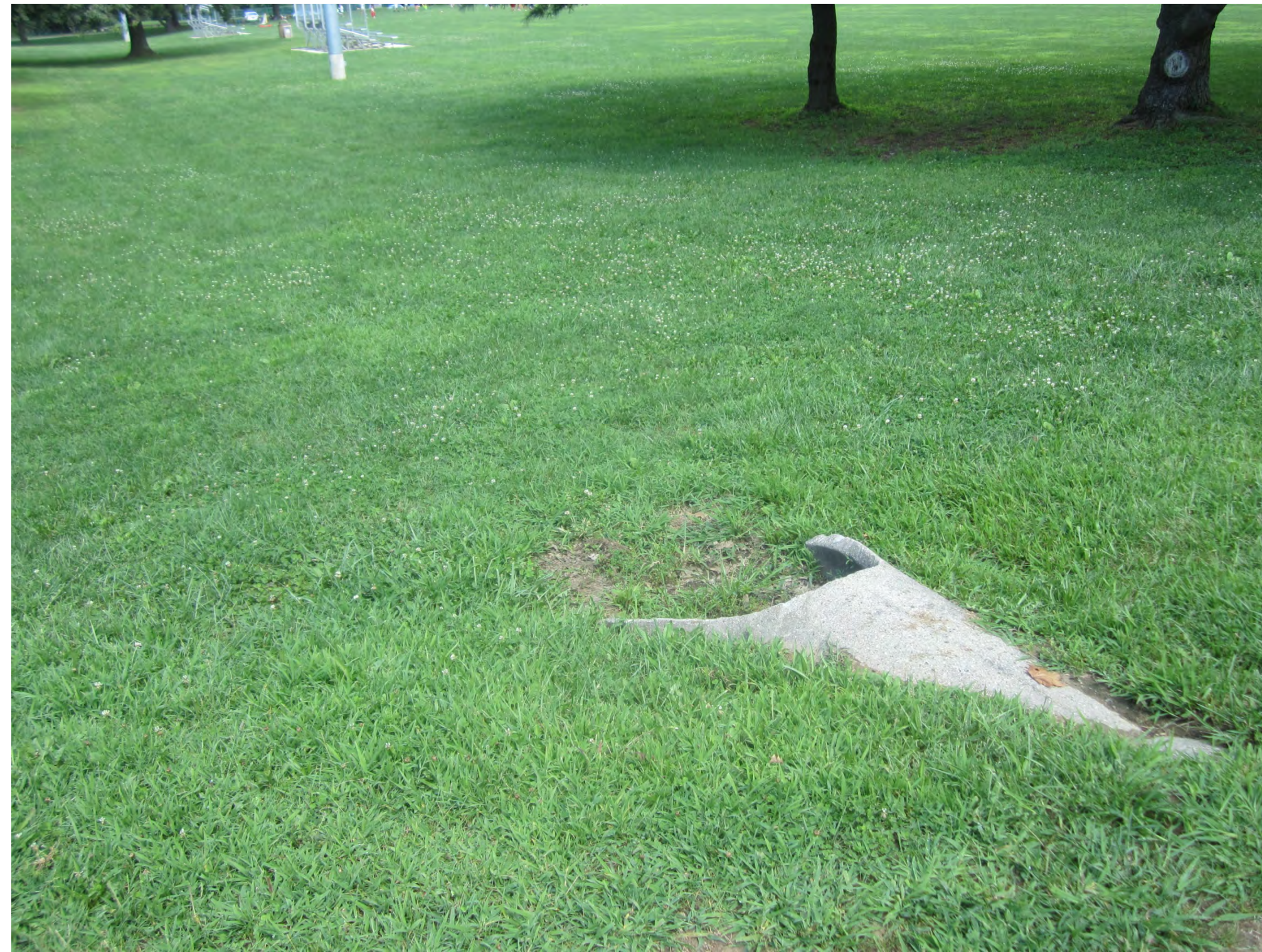
Basin #159 bottom looking west
