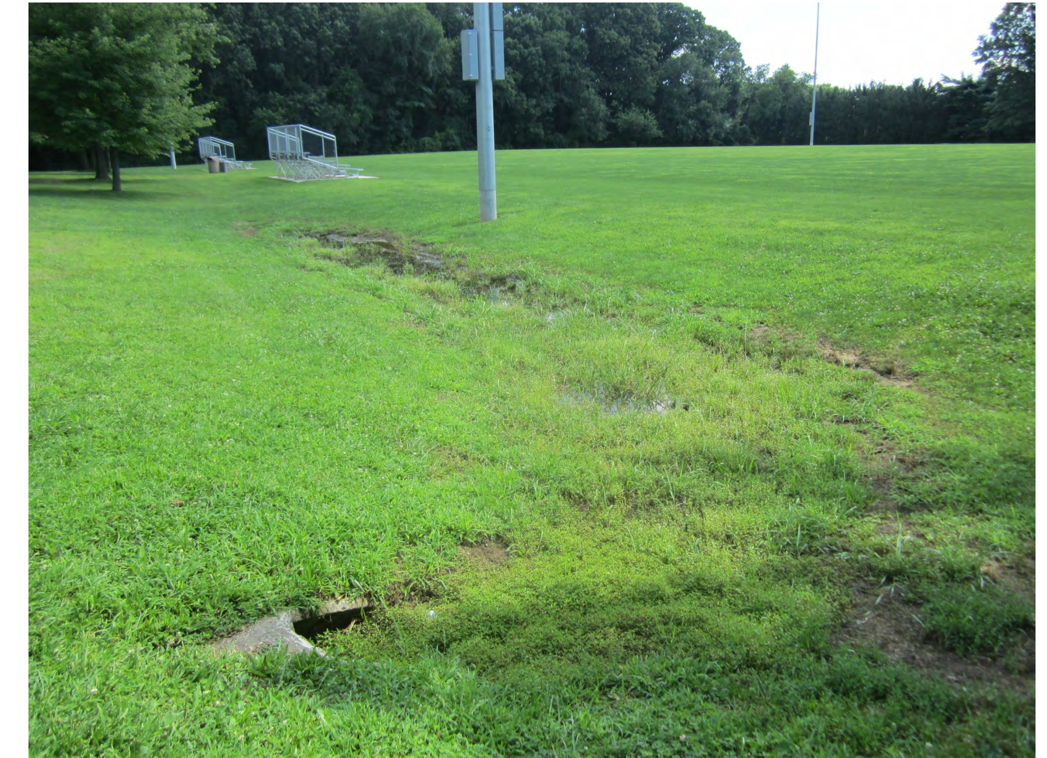
Basin #160 bottom looking north
