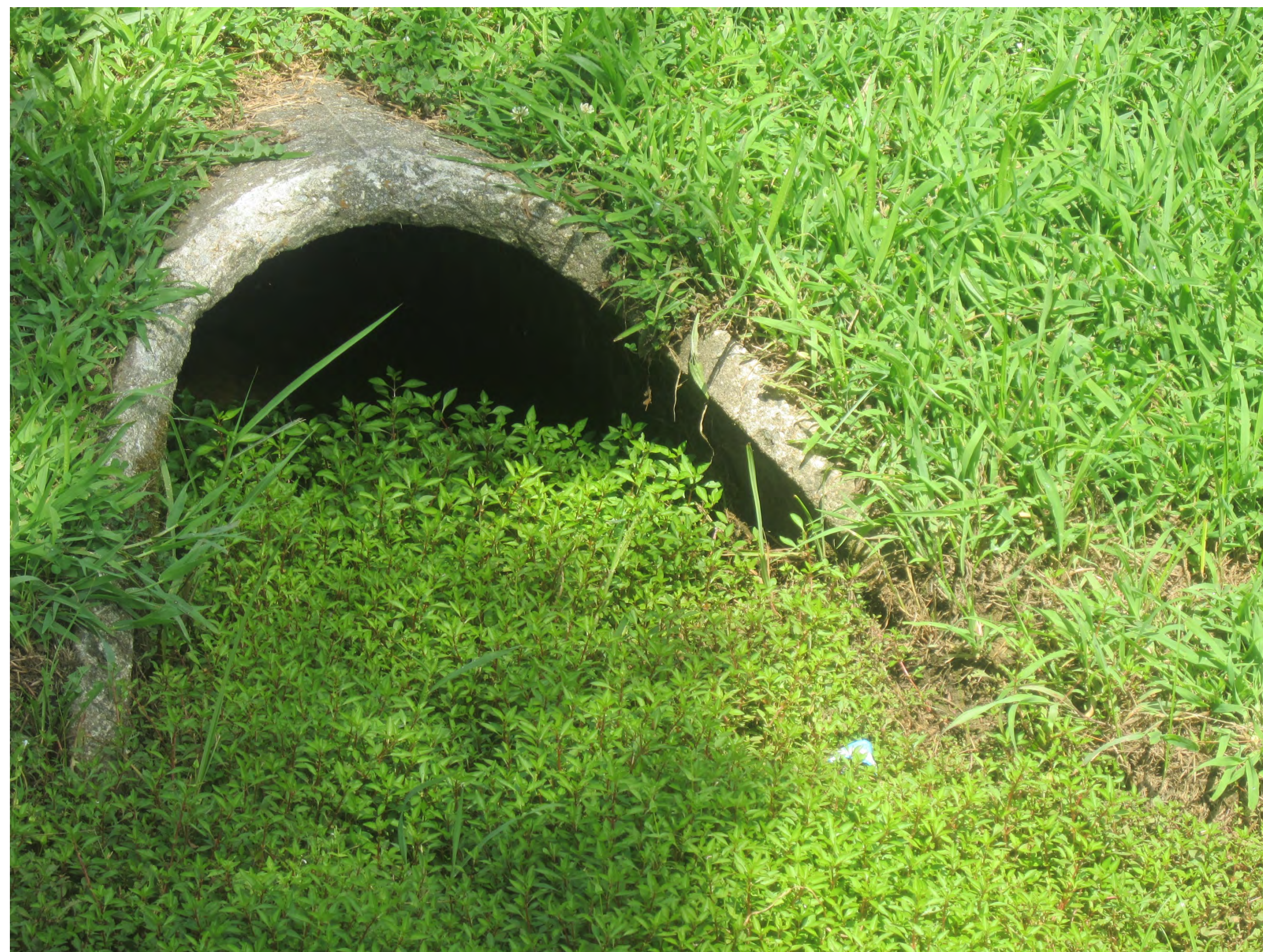
Basin #160 outlet structure
