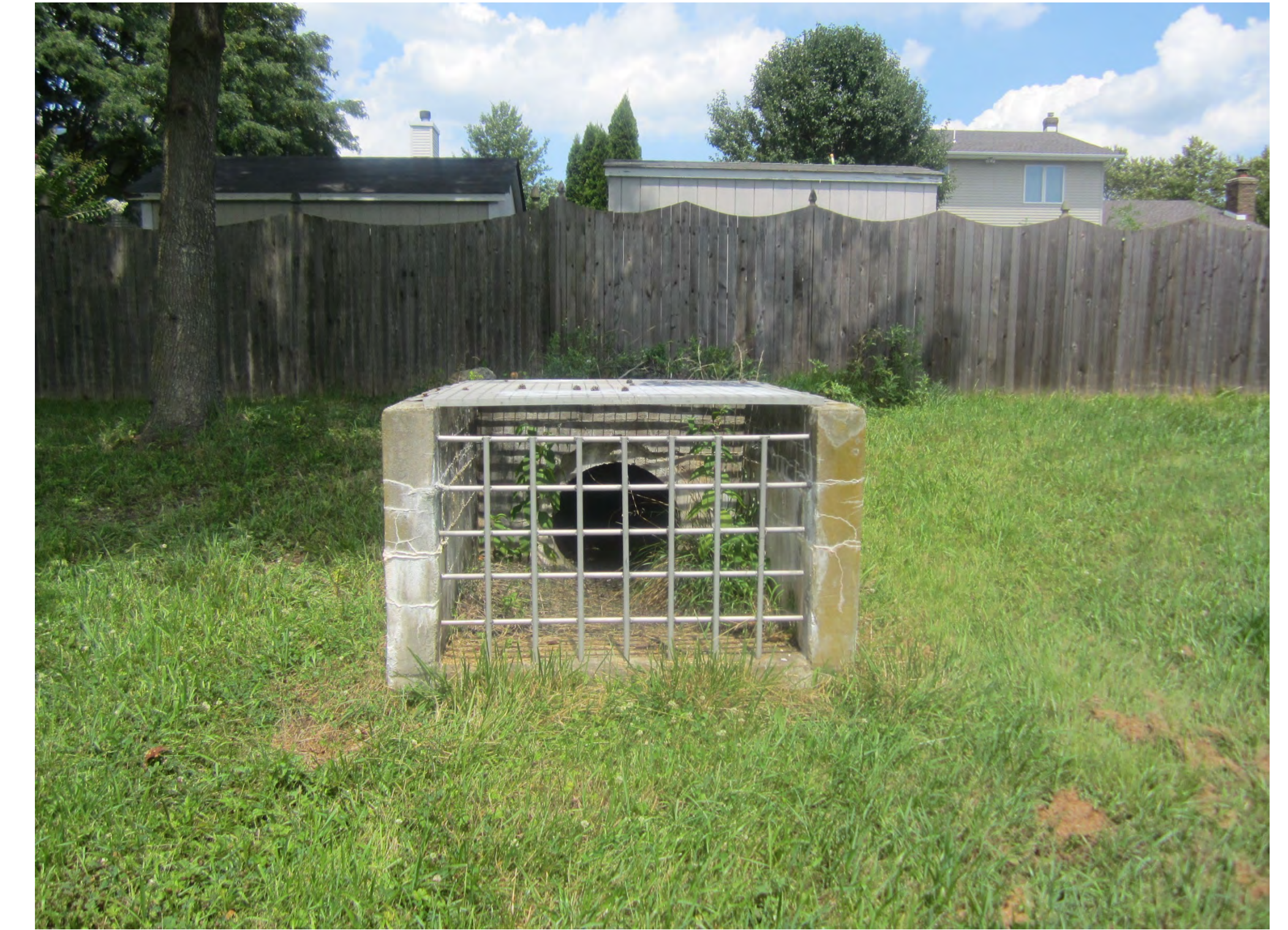
Secondary emergency overflow
