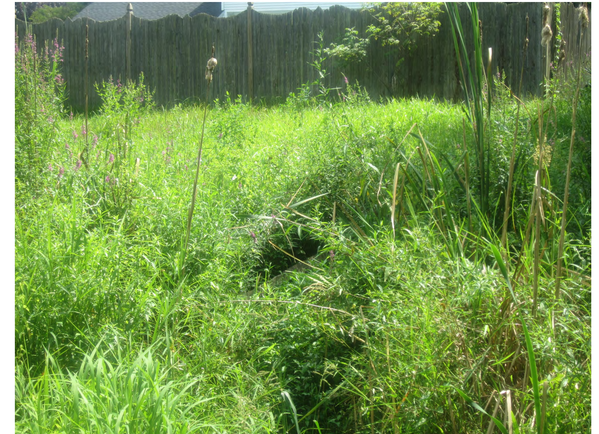
Overgrown western inlet
