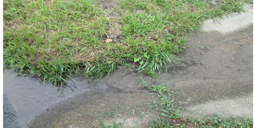
Low flow channel
