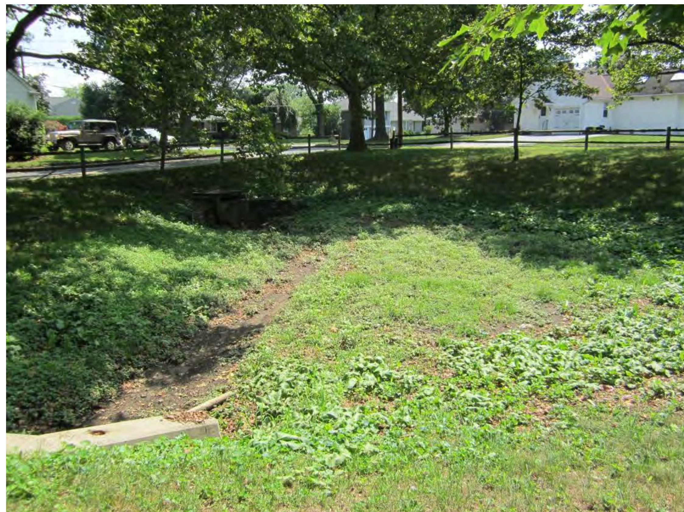
Basin bottom looking southeast
