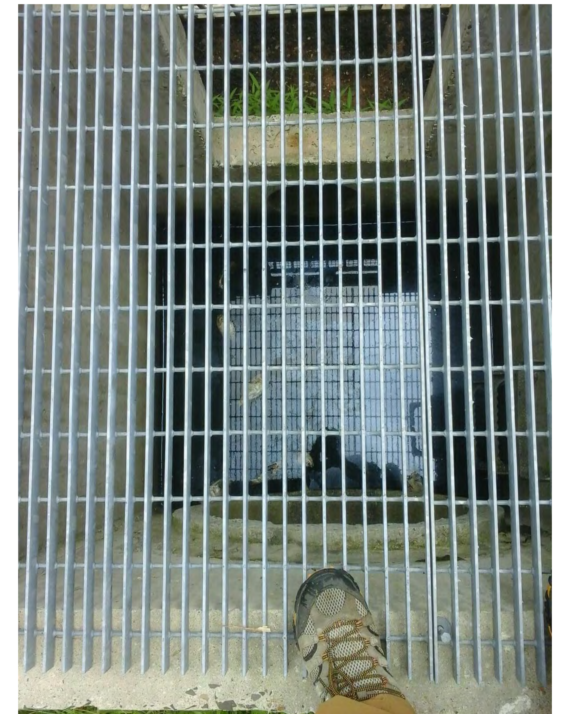
Fish in outlet structure
