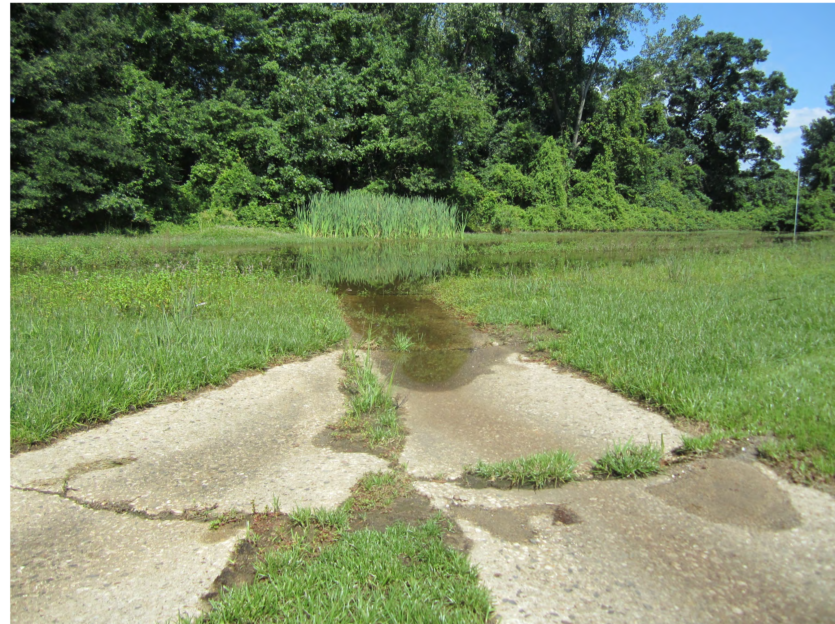
Basin bottom looking west
