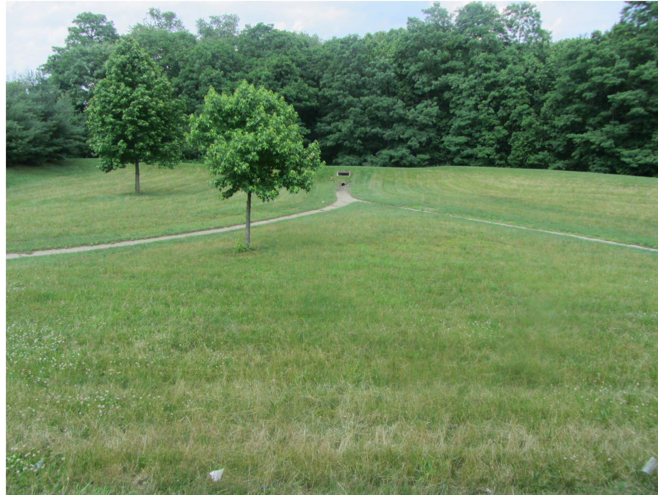
Basin bottom looking northeast
