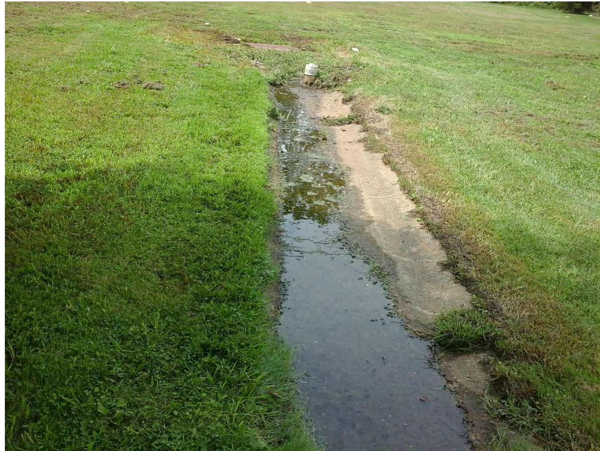
Low flow channel leading to catch basin
