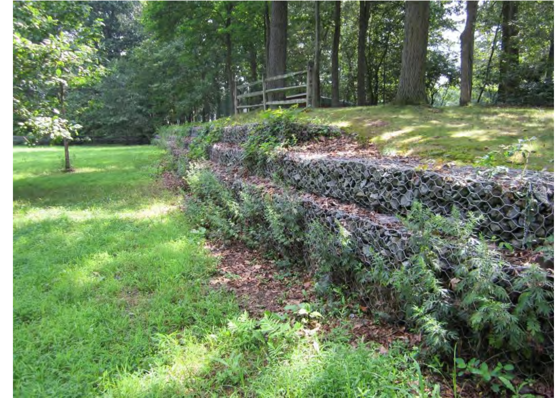
Gabion wall perimeter
