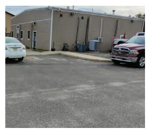
A bioretention system can be installed in the T-shaped green space that separates the two parking lots at the north end of the property to capture, treat, and infiltrate the stormwater runoff from the building by reconfiguring the downspout structure. A second bioretention system can be installed at the north end of the larger building by redirecting the nearby downspouts. A preliminary soil assessment suggests that the soils have suitable drainage characteristics for green infrastructure.
