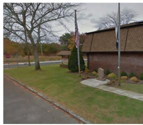
Two rain gardens can be installed at the west end of the building by redirecting downspouts into them to capture, treat, and infiltrate stormwater runoff from the rooftop. Parking spaces adjacent to the east face of the building can be retrofitted to pervious pavement to capture stormwater from the rooftop by redirecting downspouts into them. A preliminary soil assessment suggests that the soils have suitable drainage characteristics for green infrastructure.
