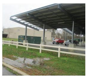
Two rain gardens can be installed near the entrance of Lot 4 to intercept stormwater from the roadways. An existing saturated area near the solar panels can be converted into a rain garden to capture, treat, and infiltrate stormwater runoff from the parking lot and improve drainage. A preliminary soil assessment suggests that the soils have suitable drainage characteristics for green infrastructure.
