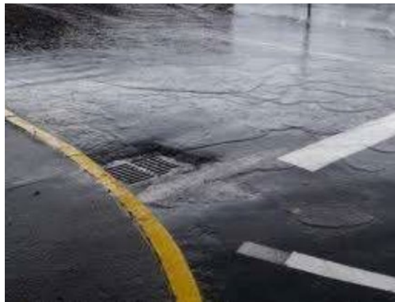
Figure 1: Stormwater draining from a parking lot
