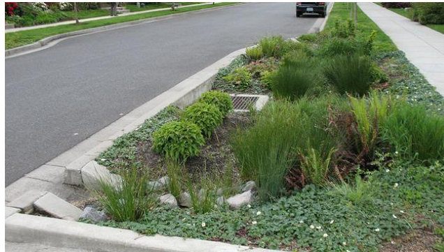
Figure 20: Example of a Green Street with incorporation of a Curb Extension and Rain Garden in Portland, OR 2
