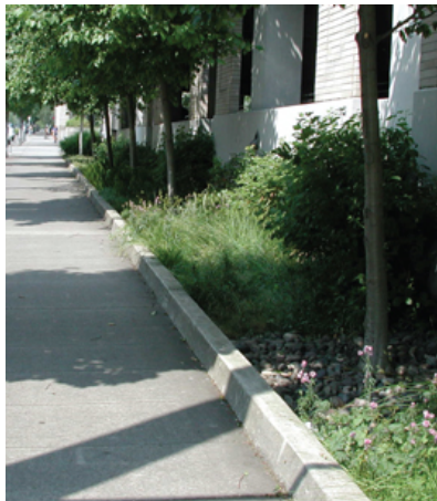
Figure 21: Example of a Green Street with incorporation of a flow-through planter in Portland, OR 2
