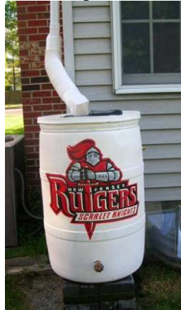
Figure 22: Example of an installed Rain Barrel in the Lower Delaware Watershed
