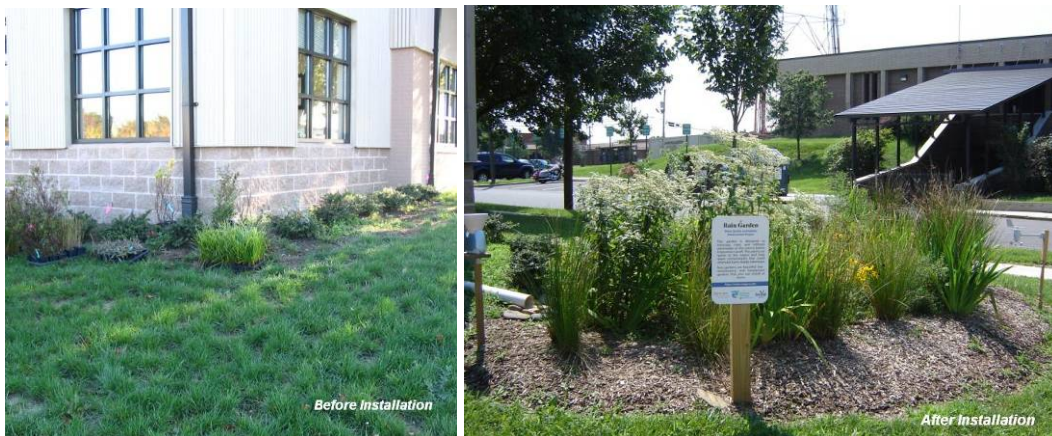
Figure 18: Example of a Rain Garden installed at the Rutgers Cooperative Extension of Burlington County, NJ in the Lower Delaware Watershed
