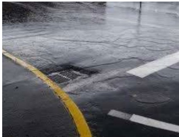
Figure 1: Stormwater draining from a parking lot
