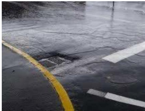
Figure 1: Stormwater draining from a parking lot
