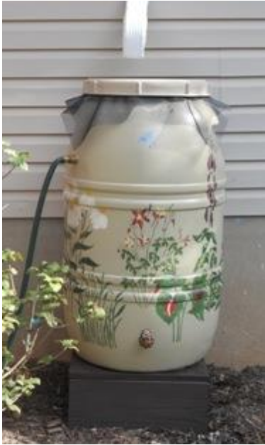
Figure 8a: Rain barrel used to disconnect a downspout with the overflow going to a flower bed
