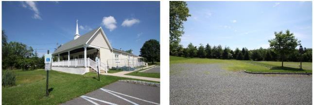
There is an existing detention basin. Rainwater also drains into the road from the parking lot. The parking spots east of the building can be replaced with porous asphalt capture and infiltrate runoff. The existing swale on the site can be retrofitted with vegetation to treat stormwater. A preliminary soil assessment suggests that more soil testing would be required before determining the soil's suitability for green infrastructure.
