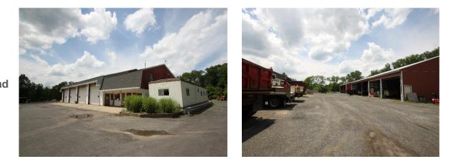
Rainwater from the roof drains onto the pavement. Downspouts from the building can be redirected into a cistern to harvest rainwater to wash department vehicles. A preliminary soil assessment suggests that more soil testing would be required before determining the soil's suitability for green infrastructure.
