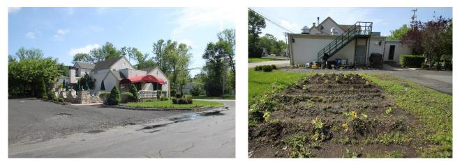
Rainwater on the site drains onto the road and pools at the entrance. Parking spaces can be replaced with porous asphalt to infiltrate stormwater. A cistern can be installed north of the building to harvest rainwater to be used by the existing garden. A bioswale and rain gardens can also be installed to capture, treat, and infiltrate runoff. A preliminary soil assessment suggests that more soil testing would be required before determining the soil's suitability for green infrastructure.
