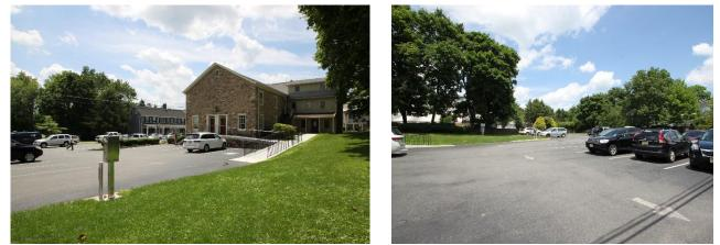
Rainwater on the site drains onto the road. The parking spots east of the building can be replaced with porous asphalt to capture runoff. There is also an opportunity for a rain garden to be installed north of the building to capture roof runoff. A preliminary soil assessment suggests that soils have suitable drainage characteristics for green infrastructure.
