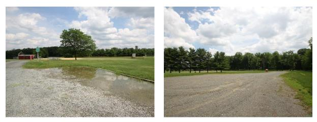
Heavy pooling occurs in the parking lots south of the tennis courts. Rain gardens can be installed along the lots to capture, treat, and infiltrate runoff, which would help remediate this issue. Additional rain gardens can be installed to manage roof runoff. A preliminary soil assessment suggests that the soils have suitable drainage characteristics for green infrastructure.
