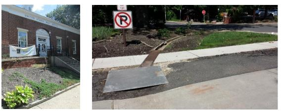
The Post Office parking lot is in poor condition and ponding occurs after rain events. Parking spaces can be replaced with pervious pavement to reduce impervious cover and promote infiltration. The concrete flow channel near the employee driveway can also be replaced with a bioswale to remove pollutants and allow stormwater to infiltrate. A preliminary soil assessment suggests that the soils have suitable drainage characteristics for green infrastructure.
