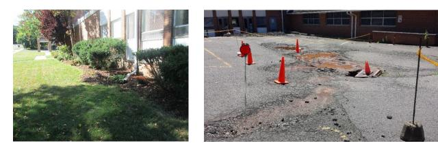
This church has severe damage to it's northern parking lot near the building. This area can be replaced with pervious pavement to infiltrate parking lot runoff. Bioretention systems can also be installed to capture, treat, and infiltrate additional parking lot runoff as well as roof runoff. A preliminary soil assessment suggests that more soil testing would be required before determining the soil's suitability for green infrastructure.
