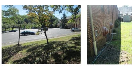
The church sits on a hill and runoff from the pathway and the downspouts is causing erosion and gullying. A bioretention system can be installed to help manage stormwater in this area. Rows of parking spaces can also be converted into pervious pavement to infiltrate parking lot runoff. A preliminary soil assessment suggests that the soils have suitable drainage characteristics for green infrastructure.
