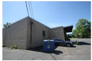
Water from the parking lot currently drains into catch basins behind the building. Parking spots can be replaced with porous asphalt to infiltrate this runoff. Downspouts can also be disconnected into a rainwater harvesting system as well. A preliminary soil assessment suggests that more soil testing would be required before determining soil suitability for green infrastructure.
