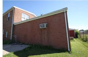
Downspouts currently direct water onto the lot beside the building. The downspouts can be connected to a rainwater harvesting feature. A preliminary soil assessment suggests that soils have suitable drainage characteristics for green infrastructure.
