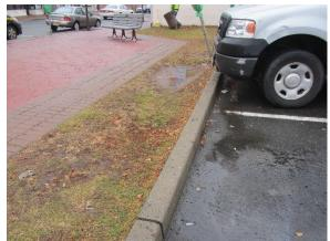
Parking spaces can be converted into pervious pavements to store stormwater runoff and allow it to slowly seep into the ground. A preliminary soil assessment suggests that more soil testing would be required before determining the soil's suitability for green infrastructure.
