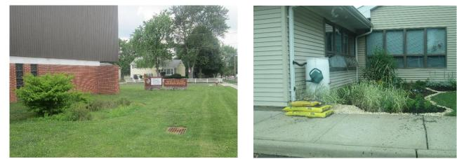
This church has two existing rain gardens and a rain barrel that captures roof runoff. Two additional rain gardens can be installed to infiltrate additional roof runoff. Parking spaces can be replaced with porous asphalt to reduce impervious cover and manage stormwater. A preliminary soil assessment suggests that the soils have suitable drainage characteristics for green infrastructure.
