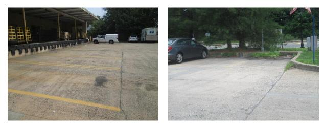
Parking spaces along the southern section of the parking lot can be converted into pervious pavement to infiltrate stormwater runoff. A preliminary soil assessment suggests that the soils have suitable drainage characteristics for green infrastructure.
