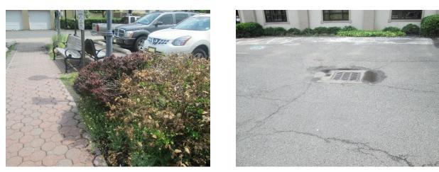
Parking lots were in poor condition at the time of assessment. Parking spaces can be converted into pervious pavement when the parking lot is repaved. A preliminary soil assessment suggests that the soils have suitable drainage characteristics for green infrastructure.
