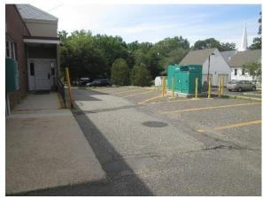
The fire department's runoff drains into directly connected downspouts. Parking lot runoff flows into the grass area to the southeast. Parking spaces can be replaced with pervious pavement to capture and infiltrate stormwater. A preliminary soil assessment suggests that more soil testing would be required before determining the soil's suitability for green infrastructure.
