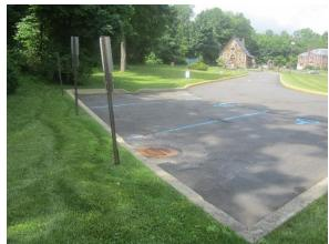
Multiple rows of parking spots can be replaced with pervious pavement to provide stormwater an opportunity to infiltrate. Building a rain garden adjacent to the northwest corner of the church can capture, treat, and infiltrate roof runoff. A preliminary soil assessment suggests that the soils have suitable drainage characteristics for green infrastructure.
