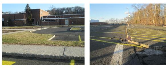
Rows of parking spots north and west of the school can be replaced with pervious pavement to provide stormwater being generated by the parking lots an opportunity to infiltrate. A preliminary soil assessment suggests that the soils have suitable drainage characteristics for green infrastructure.
