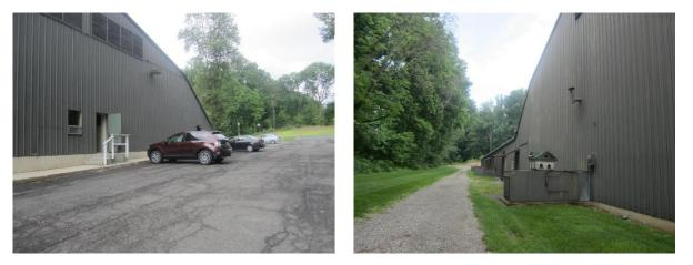
Parking spots north and west of the building can be replaced with porous asphalt to capture and infiltrate stormwater. A preliminary soil assessment suggests that the soils have suitable drainage characteristics for green infrastructure.
