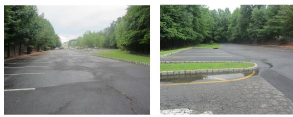
Two rows of parking spots south of the school can be replaced with porous asphalt to capture and infiltrate stormwater. A preliminary soil assessment suggests that more soil testing would be required before determining the soil's suitability for green infrastructure.
