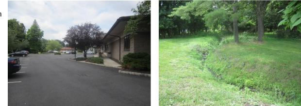
Stormwater is currently directed to an existing trench. Parking spots west and south of the building can be replaced with porous asphalt to capture and infiltrate stormwater. A preliminary soil assessment suggests that more soil testing would be required before determining the soil's suitability for green infrastructure.
