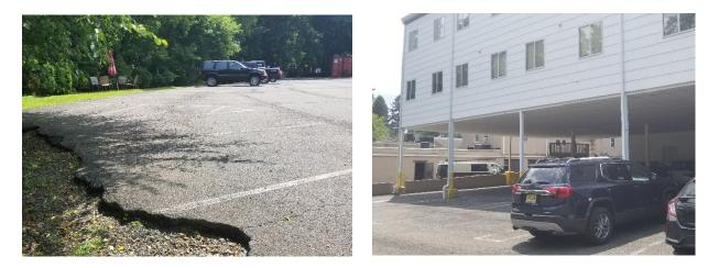
Pervious pavement can be installed in the back parking lot to capture, treat, and infiltrate parking lot runoff. Downspout planter boxes can be installed at the bases of the downspouts connected to the support beams at the southeast corner of the building to capture and filter stormwater. A preliminary soil assessment suggests that more soil testing would be required before determining the soil's suitability for green infrastructure.
