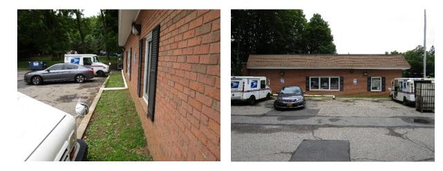
Parking spaces in the parking lot to the east of the building can be converted to porous pavement to capture and infiltrate stormwater runoff from the parking lot and the downspout. A septic system in the turfgrass area north of the building limits rain garden opportunities. A preliminary soil assessment suggests that the soils have suitable drainage characteristics for green infrastructure.
