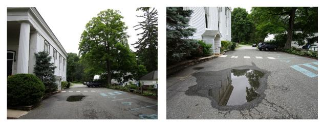
Parking spaces in the parking lot to the south/front of the building can be converted to porous pavement to capture and infiltrate stormwater runoff from the parking lot. A preliminary soil assessment suggests that the soils have suitable drainage characteristics for green infrastructure.
