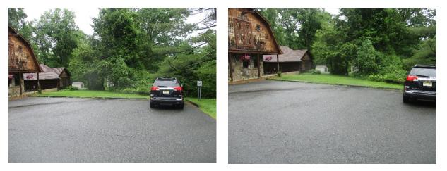
A rain garden can be installed south of the building to capture stormwater runoff from both the rooftop of the building as well as the parking lot. Downspout planter boxes can be installed in front of the building to capture the stormwater runoff from the western rooftop. A preliminary soil assessment suggests that the soils have suitable drainage characteristics for green infrastructure.
