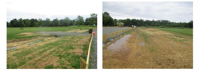
A rain garden can be installed along the northern edge of the parking lot area to help infiltrate the pooling stormwater in that area. A preliminary soil assessment suggests that the soils have suitable drainage characteristics for green infrastructure.
