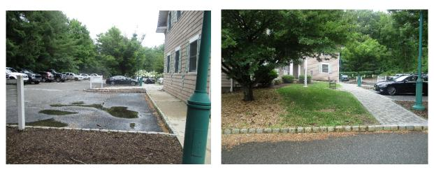
Pervious pavement can be installed in the parking spaces west of the building to capture and infiltrate stormwater. A rain garden can be installed to the northwest of the building to capture, treat, and infiltrate stormwater runoff from the roof. A preliminary soil assessment suggests that the soils have suitable drainage characteristics for green infrastructure.
