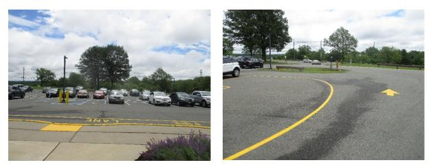
Pervious pavement can be installed in the southernmost row of the parking lot to capture, treat, and infiltrate stormwater runoff from the parking lot. A preliminary soil assessment suggests that the soils have suitable drainage characteristics for green infrastructure
