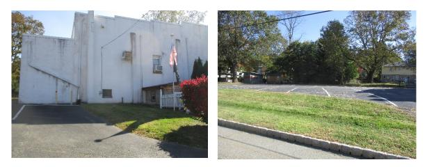
Half of the building's rooftop runoff and part of the parking lot runoff, can be treated with pervious pavement in the east strip of the parking lot. A preliminary soil assessment suggests that more soil testing would be required before determining the soil's suitability for green infrastructure.
