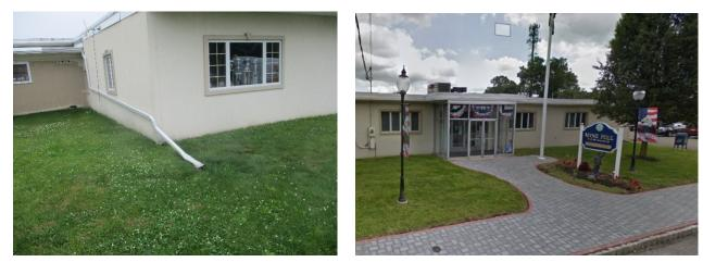
A rain garden can be installed in the turfgrass area near the building to capture, treat, and infiltrate rooftop runoff. A preliminary soil assessment suggests that more soil testing would be required before determining the soil's suitability for green infrastructure.
