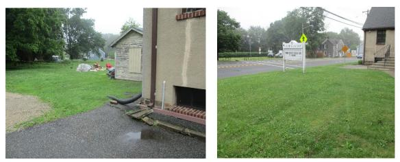
Rain gardens can be installed on the north, southeast, and south sides of the building near disconnected downspouts to capture, treat, and infiltrate rooftop runoff. A preliminary soil assessment suggests that the soils have suitable drainage characteristics for green infrastructure.
