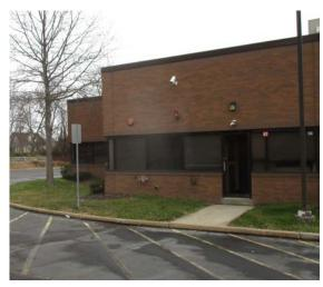
Sections of parking spaces can be converted to porous pavement to capture and infiltrate stormwater runoff from the parking lot. A preliminary soil assessment suggests that the soils have suitable drainage characteristics for green infrastructure.
