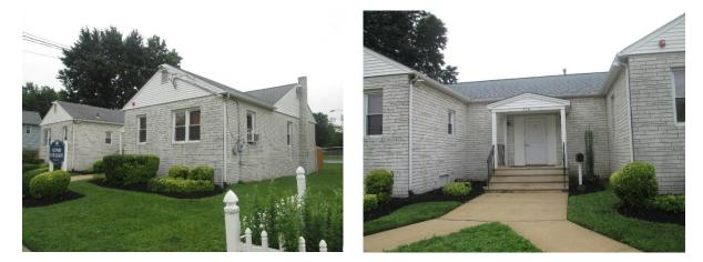
West of the building a rain garden can be installed to capture, treat, and infiltrate roof runoff by disconnecting and redirecting nearby downspouts into it. A preliminary soil assessment suggests that the soils have suitable drainage characteristics for green infrastructure.
