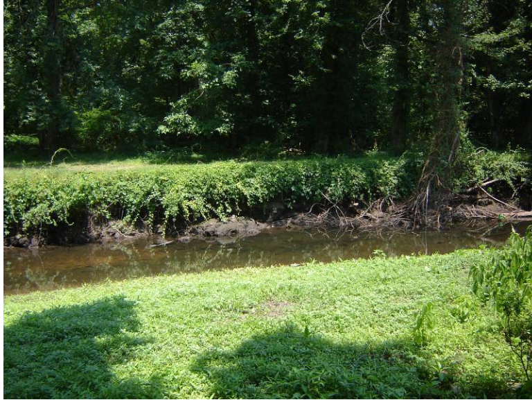
Figure 2: Photograph of unstable streambanks along Tenakill Brook at Memorial Park.
