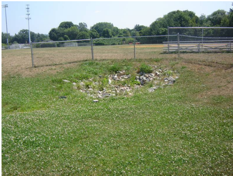
Figure 3: Photograph of swale inlet to undergo a retrofit.
