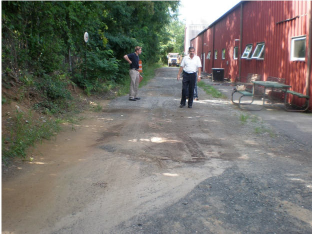
The emergency access road behind the DPW facility building was a dirt road that sloped towards the Troy Brook.
