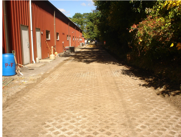
Long view of the pavers immediately after installation.
