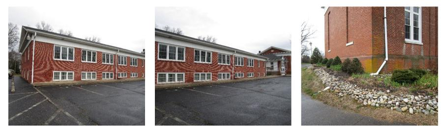
The parking spaces southwest of the building can be converted to pervious pavement to allow runoff from the roof and pavement to infiltrate through the surface. A rain garden can be installed in the front turfgrass area to capture, treat, and infiltrate runoff from the roof and driveway. A preliminary soil assessment suggests that the soils have suitable drainage characteristics for green infrastructure.
