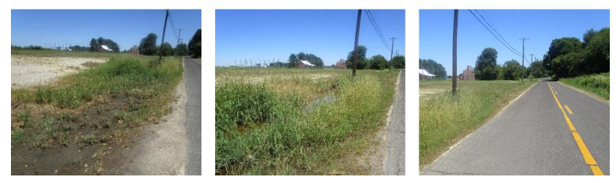
The turfgrass area alongside the road west of the building can be converted into a bioswale. Currently, the soil along the roadside is eroding and puddles with stormwater runoff. This problem can be solved with the creation of a bioswale. A preliminary soil assessment suggests that more soil testing would be required before determining the soil's suitability for green infrastructure.
