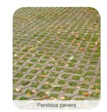
To protect and repair our waterways, reduce flooding, and stop erosion, stormwater runoff has to be better managed. Impervious surfaces need to be disconnected with green infrastructure to prevent stormwater runoff from flowing directly into New Jersey's waterways. Disconnection redirects runoff from paving and rooftops to pervious areas in the landscape.
