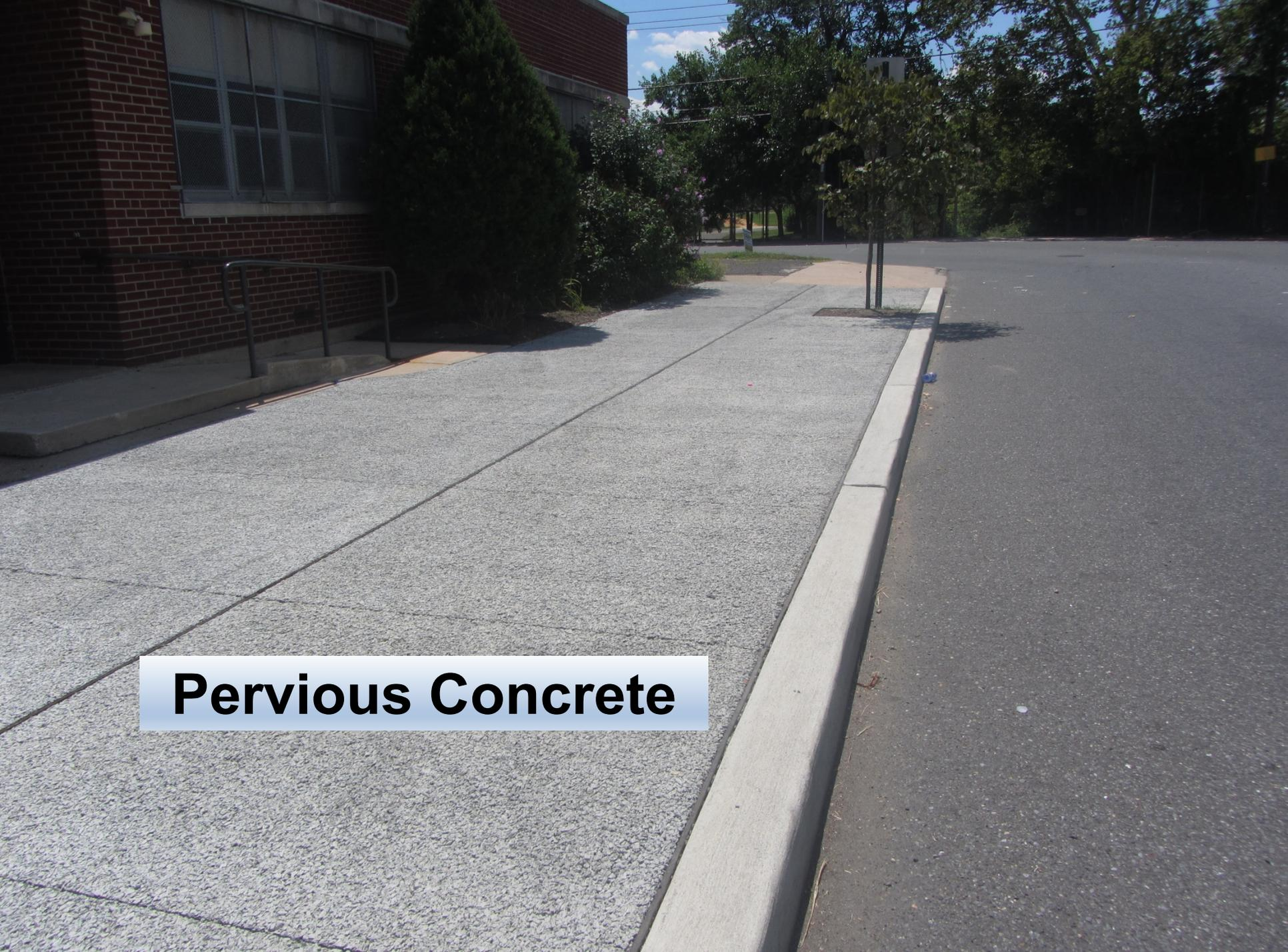
A photograph showing a sidewalk made of pervious concrete. The sidewalk is light gray and has a porous, aggregate-like texture. It runs alongside a brick building on the left, which has a metal handrail. To the right of the sidewalk is a concrete curb and an asphalt road. The background features green trees and a clear blue sky.
