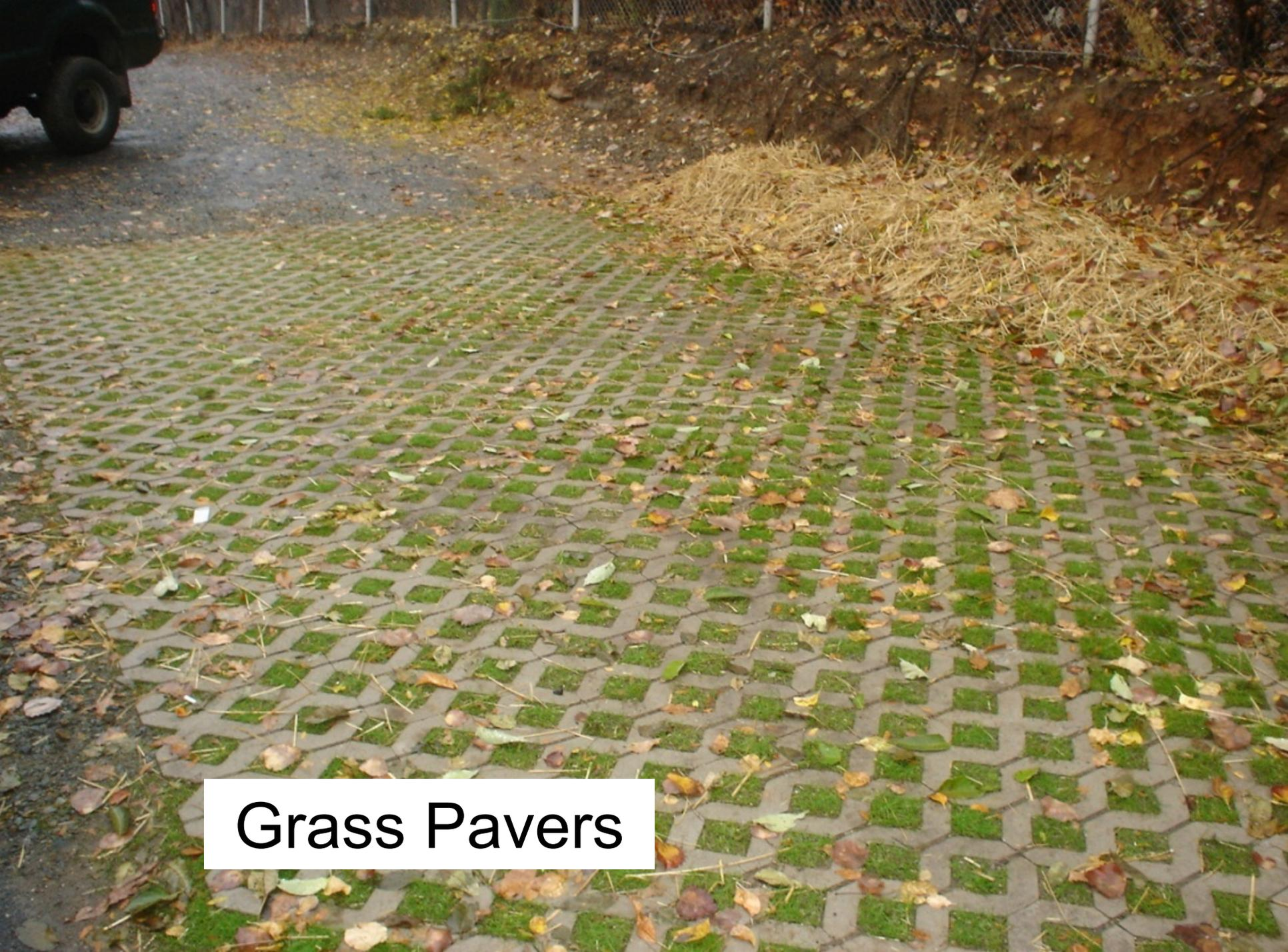
A photograph showing a driveway paved with interlocking concrete grass pavers. The pavers are arranged in a grid pattern, with green grass growing through the openings. The driveway is covered with fallen autumn leaves and some dry grass. In the background, there is a chain-link fence and a dark vehicle parked on the left. The overall scene is outdoors during autumn.
