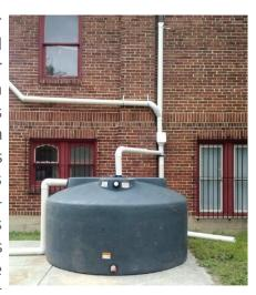
power by designing and installing rainwater harvesting systems that allow the collection, storage, and reuse of the rainwater.
