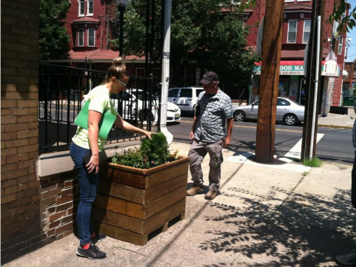
Downspout planter box in North Camden
