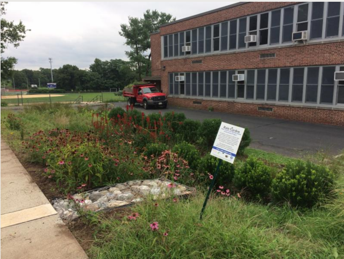
Governor Livingston High School, Berkeley Heights, New Jersey AFTER maintenance, August 2018
