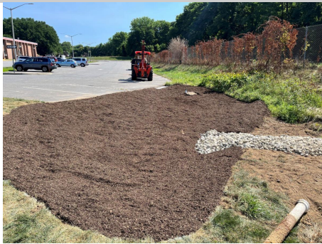
Phillipsburg Elementary School rain garden construction, August 2022
