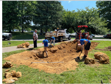
Phillipsburg Middle School rain garden construction, August 2022
