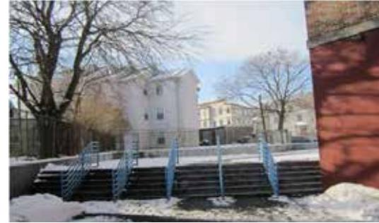
The site is Paterson School #8 located at 45 Chadwick Street. There is little to no identifiable slope to the site. There are no external downspouts on the building. The pavement appears to be in good condition, and the site is almost entirely impervious. Depaving and stormwater planters could be used to reduce runoff.
