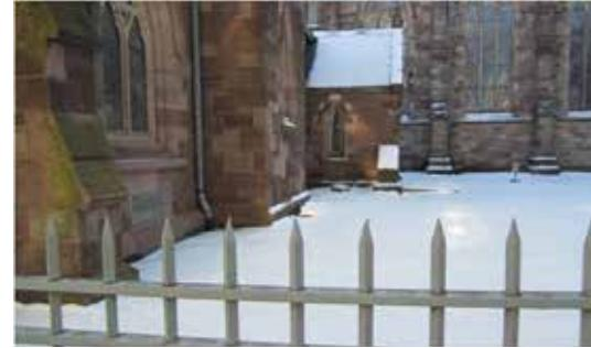
The site is the Cathedral of St. John the Baptist located at 381 Main Street. The site seems to slope from north to south. All of the existing pavement appears to be in good condition. The north side of the site has a grassed area with downspouts that could be disconnected into a rain garden.
