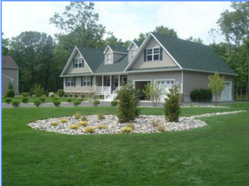
Doebley & Dad Construction Company built this home in Egg Harbor Township using EPA WaterSense® new home specifications
