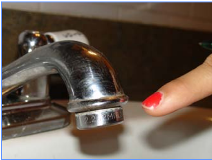
A Rahway High School Student notices that one of the school's faucets uses 2.22 gallons of water per minute.
