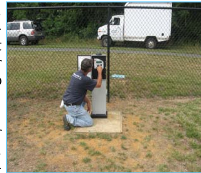
Installation of a Smart Controller at Thompson Park Soccer Field in East Greenwich Twp., NJ
