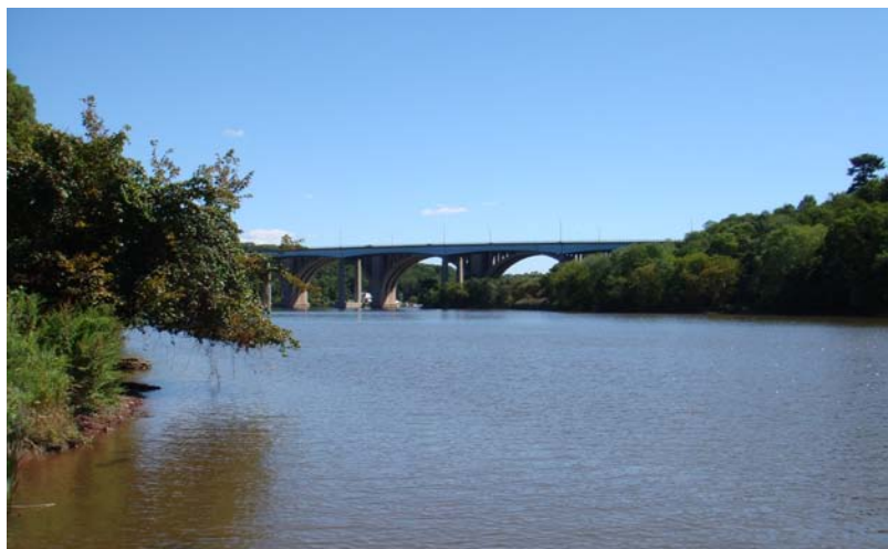
Route 1 Bridges over Raritan from Donaldson Park
