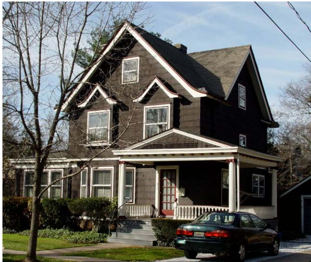
235 Lincoln Avenue, Livingston Manor District (Table 9.3, Item 7)
