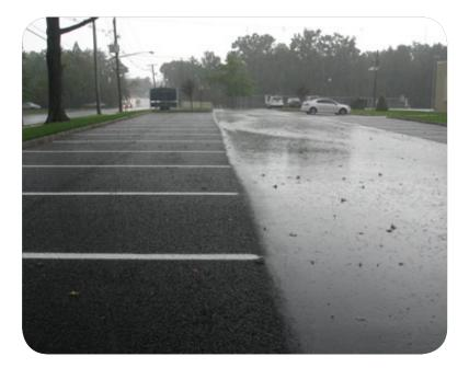
**POROUS ASPHALT** It is common to design porous asphalt in the parking stalls of a parking lot. This saves money and reduces wear. **DRAINAGE AREA** The drainage area of the porous asphalt system is the conventional asphalt cartway and the porous asphalt in the parking spaces. Runoff from the conventional asphalt flows into the porous asphalt parking spaces.
