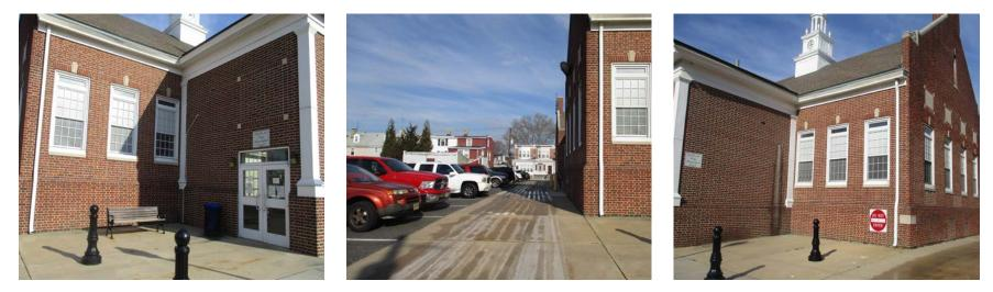
Stormwater is currently draining from south to north across the site. Paved areas to the east and west and of the south entrance can be converted to porous asphalt to capture and treat roof runoff. A preliminary soil assessment suggests that more soil testing would be required before determining the soil's suitability for green infrastructure.
