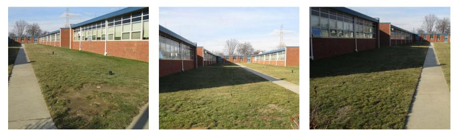
Stormwater is currently draining across the site to nearby catch basins. Building downspouts can be disconnected and directed into rain gardens. Installing rain gardens adjacent to the building can capture, treat, and infiltrate roof runoff. A preliminary soil assessment suggests that more soil testing would be required before determining the soil's suitability for green infrastructure.
