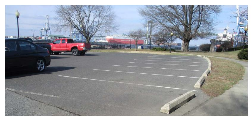
This site is located at Proprietors Park, directly adjacent to the Gloucester City Marina. Stormwater is currently draining from east to west across the site. Parking spaces in the Proprietors Park parking lot can be converted to porous asphalt to capture and treat stormwater runoff. This will help decrease the amount of polluted water that drains to the Delaware River.
