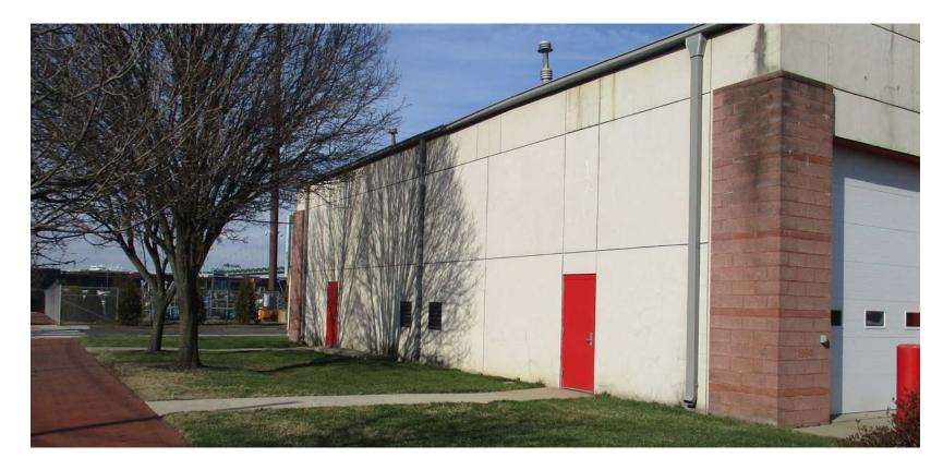
This site is located at the Gloucester City Fire Department. Stormwater is currently draining to nearby catch basins. Downspouts along the building can be directed into rain gardens to capture, treat, and infiltrate runoff. A cistern connected to building downspouts can capture water, allowing it to be used for washing vehicles and equipment.
