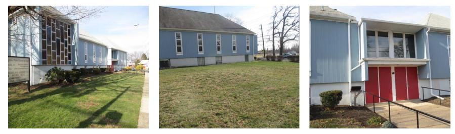
Stormwater is currently draining across the site to nearby catch basins. Building downspouts can be disconnected and directed into a rain garden. Installing a rain garden adjacent to the building can capture, treat, and infiltrate roof runoff. A preliminary soil assessment suggests that more soil testing would be required before determining the soil's suitability for green infrastructure.
