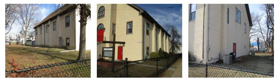
Stormwater is currently draining across the site to nearby catch basins. Building downspouts can be directed into a rain garden. Installing a rain garden adjacent to the building can capture, treat, and infiltrate roof runoff. A preliminary soil assessment suggests that more soil testing would be required before determining the soil's suitability for green infrastructure.
