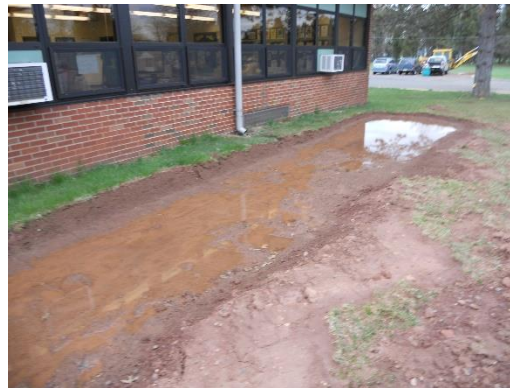
Post excavation April 2011
