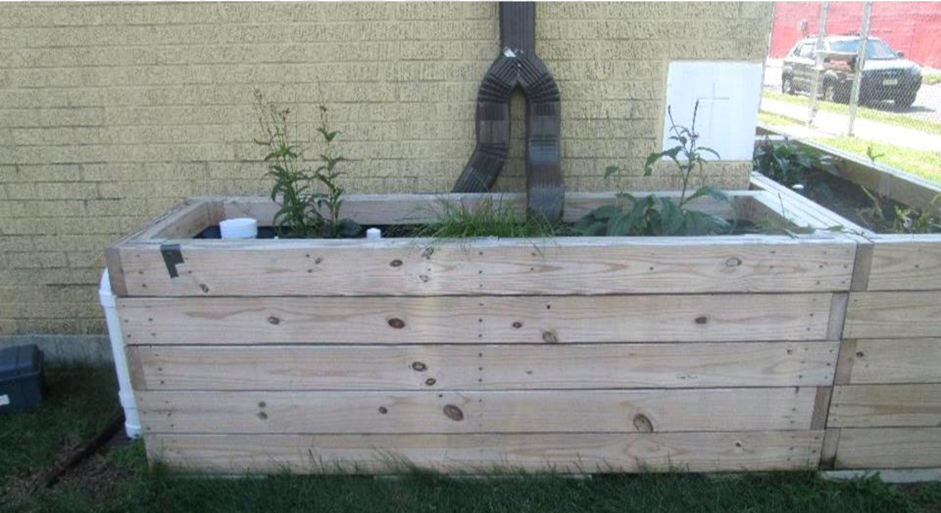
Downspout Planter Boxes at Acelero Harvesting System
