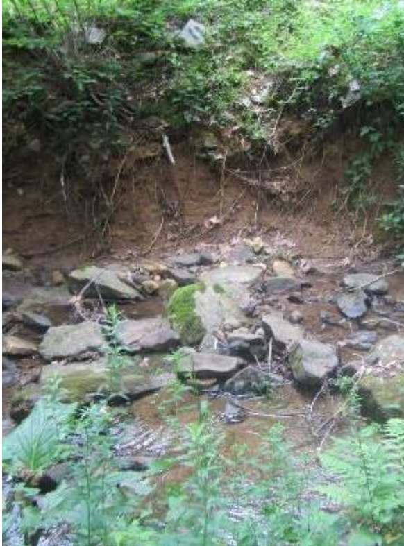
Embankment Destabilization
