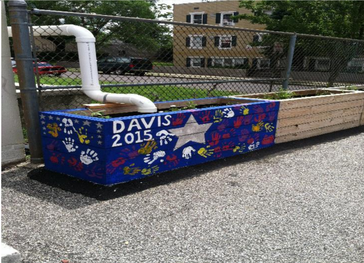
Downspout Planter Boxes at Davis School Harvesting System
