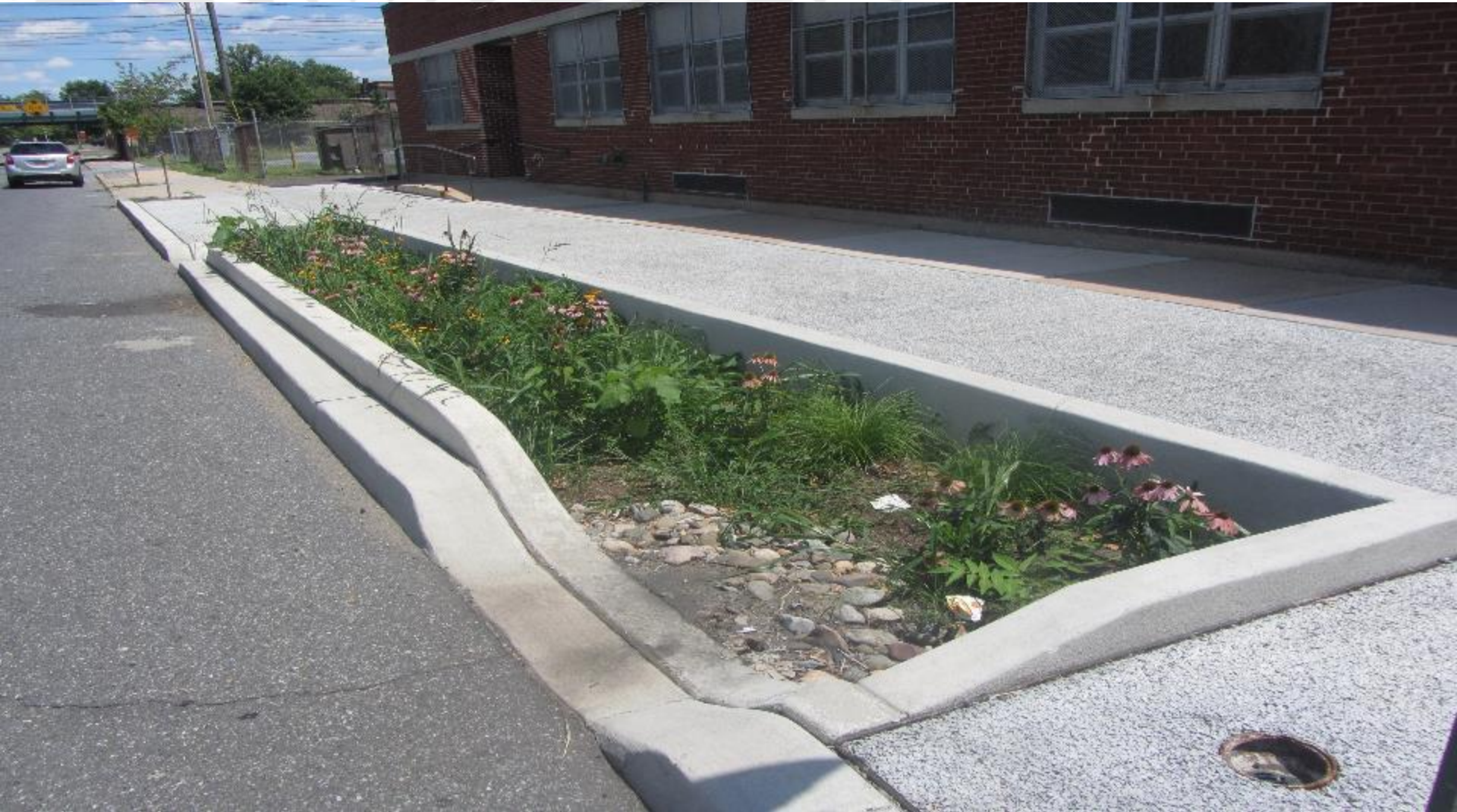
Stormwater Planter at the Brimm School
