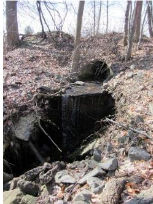
Outlet Destabilization
