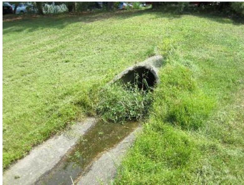
Clogged low-flow channel
