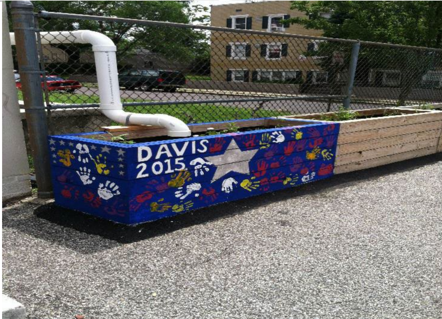
Downspout Planter Boxes at Davis School
