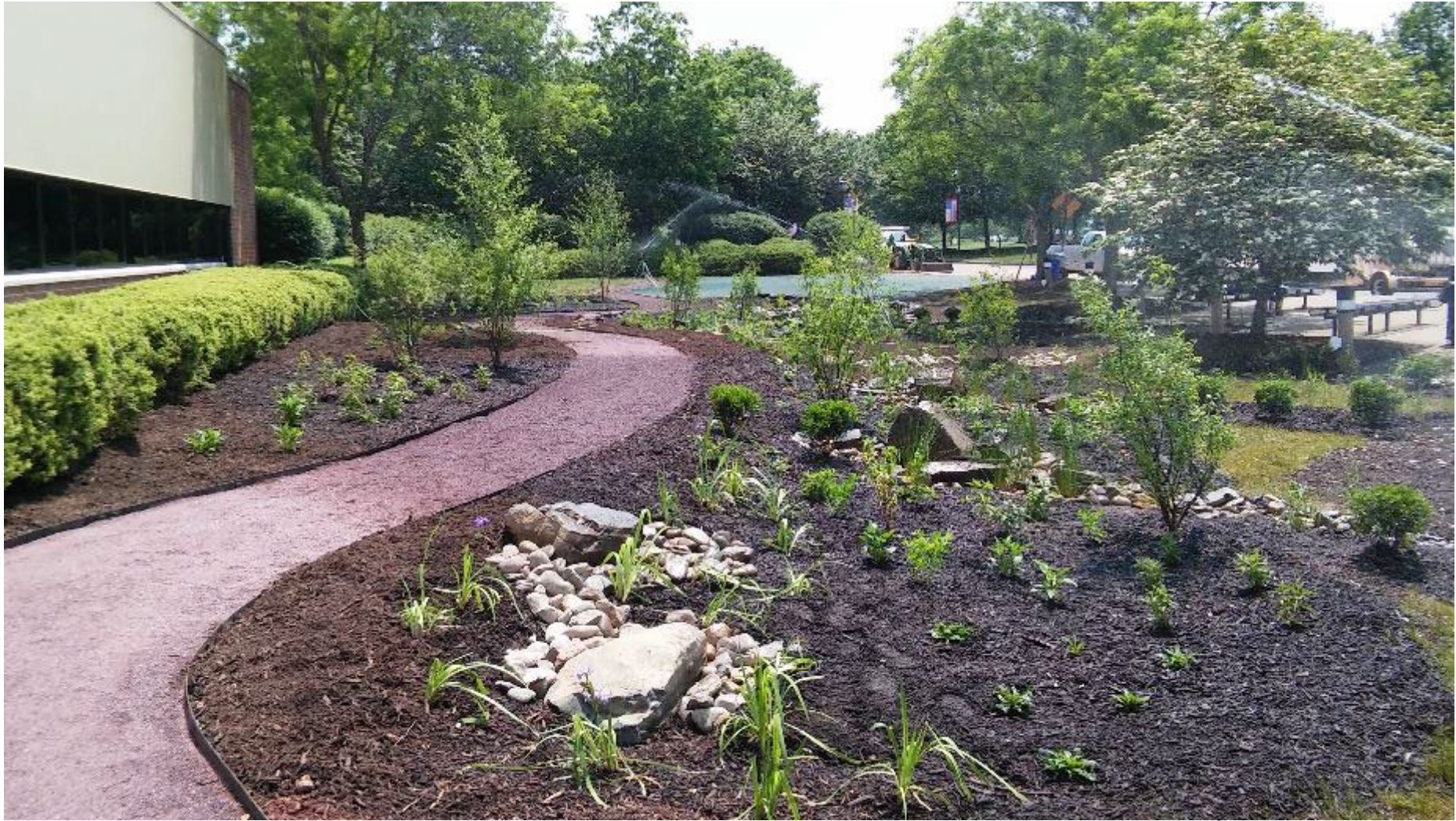
Rain garden at Hillsborough Municipal Building
