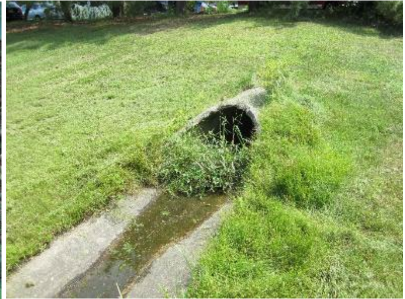
Clogged low-flow channel
