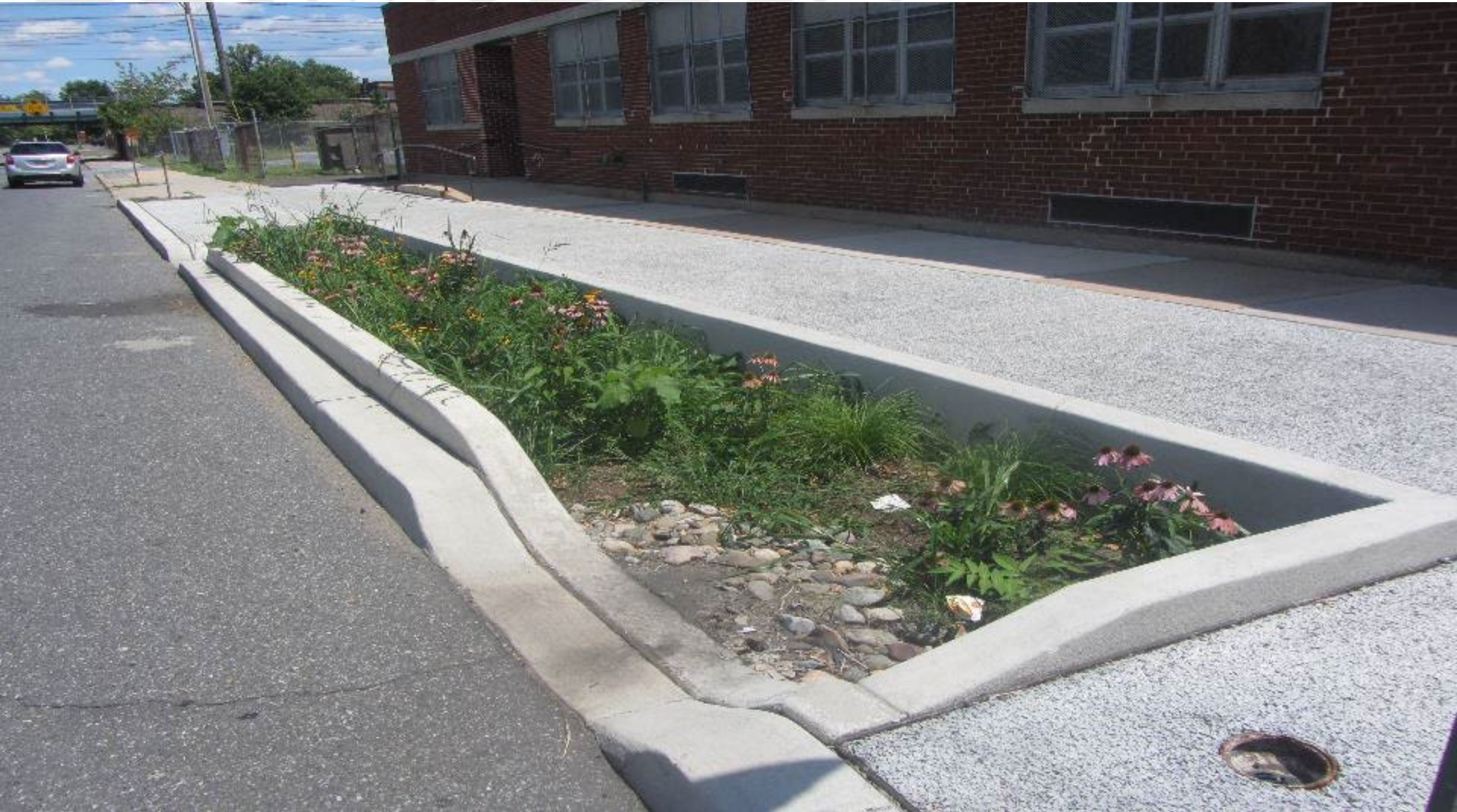
Stormwater Planter at the Brimm School
