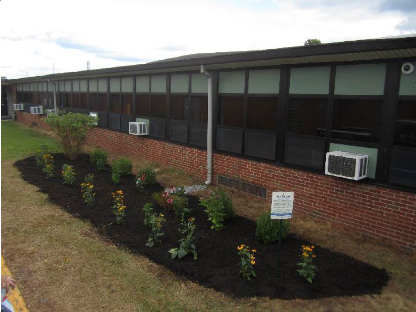
Rain garden at Woods Road School in Hillsborough
