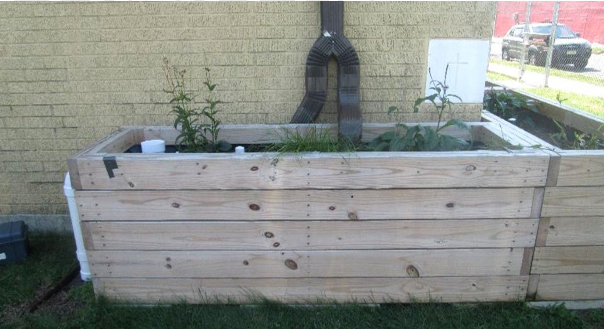
Downspout Planter Boxes at Acelero
