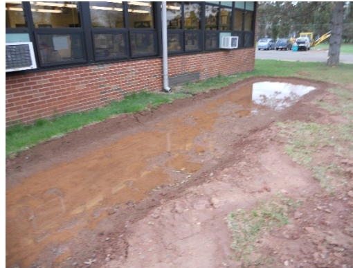
Post excavation April 2011
