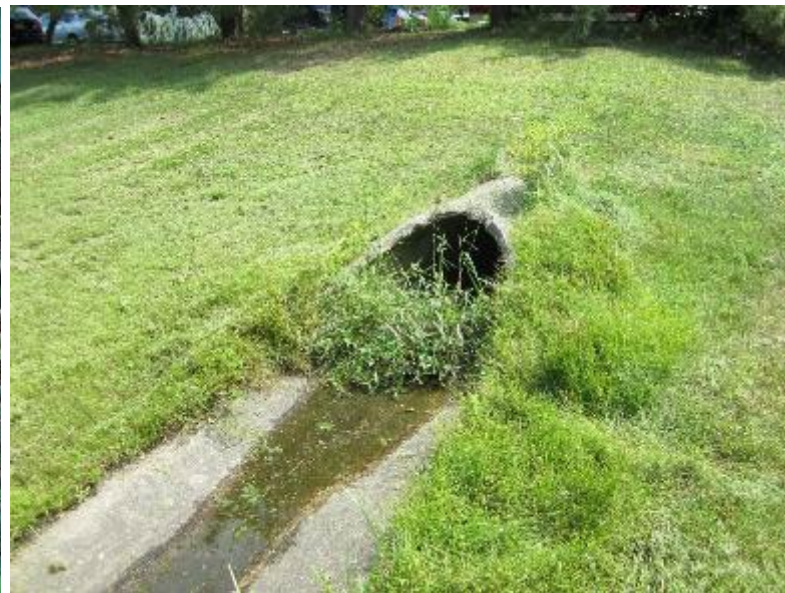
Clogged low-flow channel
