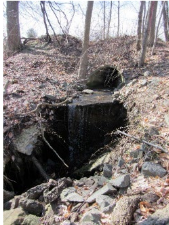
Outlet Destabilization
