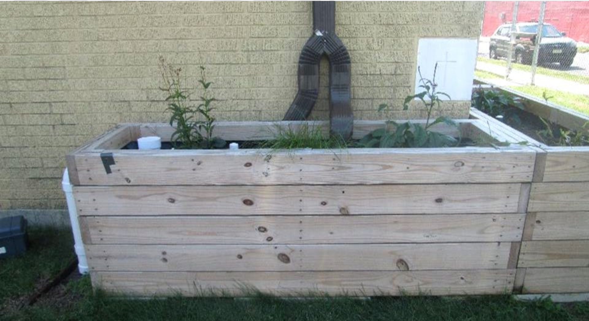
Downspout Planter Boxes at Acelero
