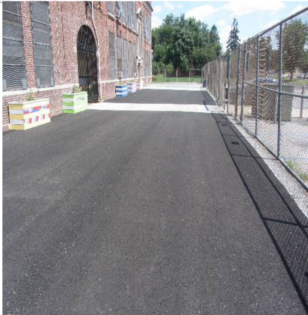
Porous Pavement at Yorkship School (Asphalt)
