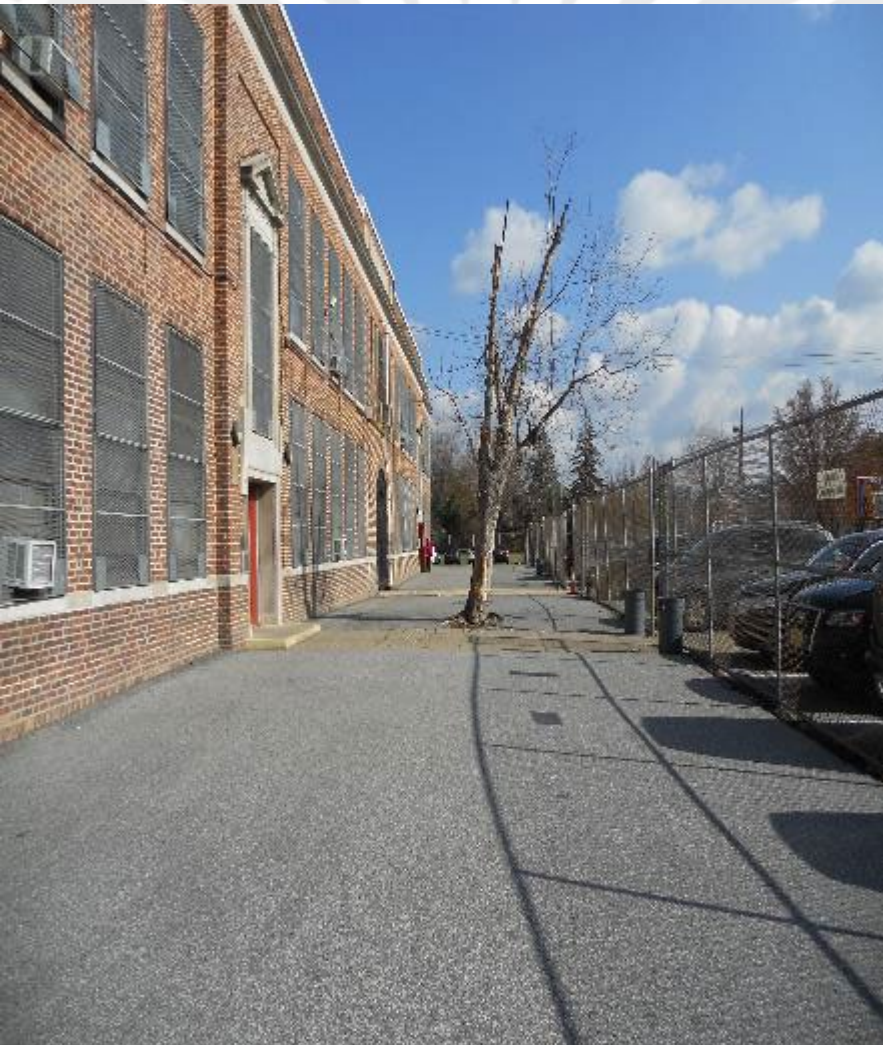
Porous Pavement at Yorkship School (Asphalt)
