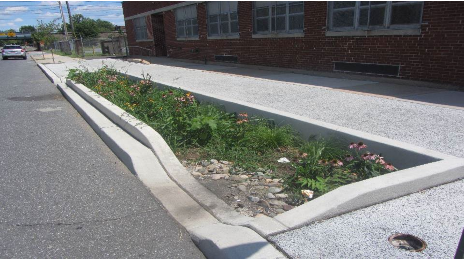
Stormwater Planter at the Brimm School in Camden, NJ
