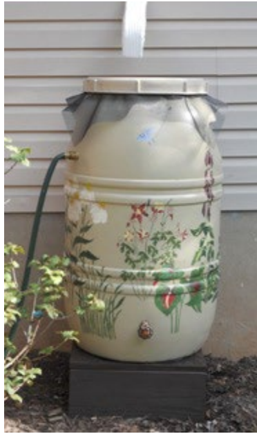
Figure 8a: Rain barrel used to disconnect a downspout with the overflow going to a flower bed
