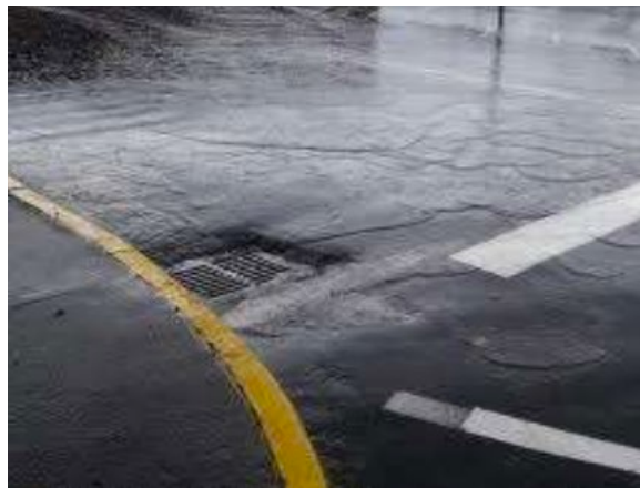
Figure 1: Stormwater draining from a parking lot
