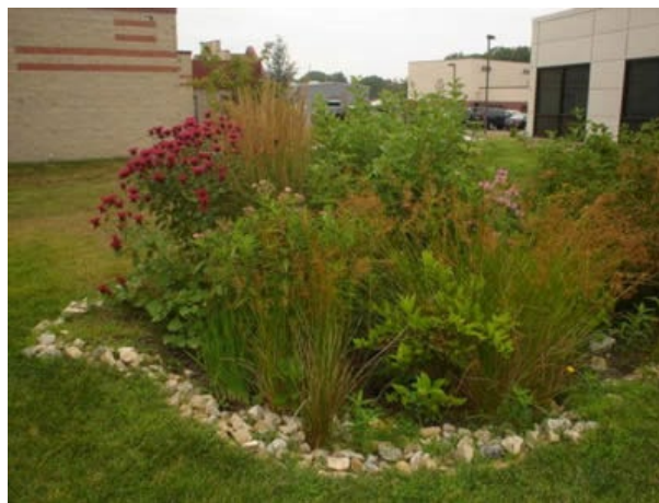
Figure 7: Rain garden outside the RCE of Gloucester County office which was designed to disconnect rooftop runoff from the local storm sewer system
