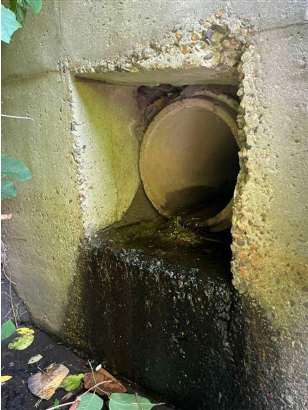
Outfall ID: SB006 (6/14/2024)
