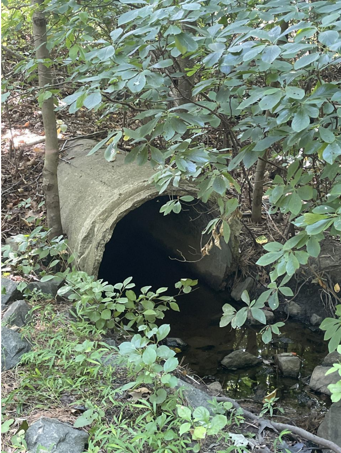
Outfall ID: AC02 (8/4/2022)
