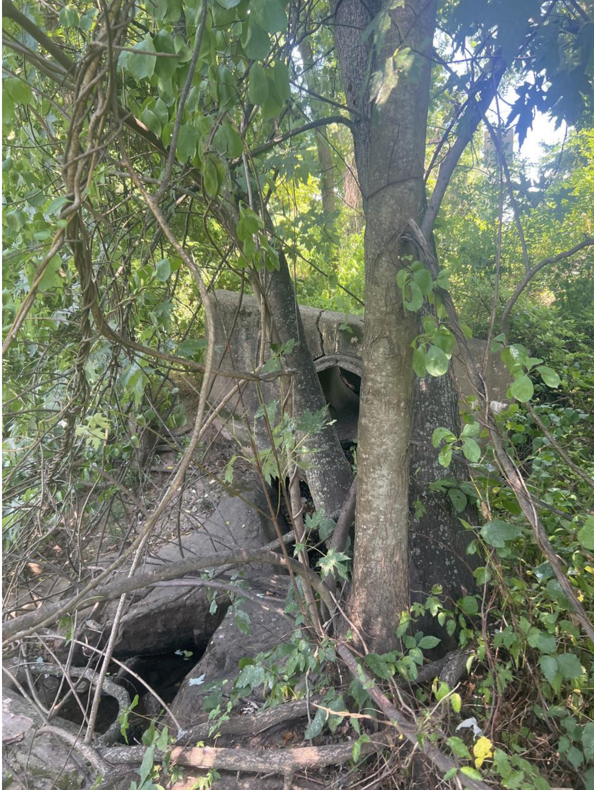
Outfall ID: AC09 (7/22/2022)
