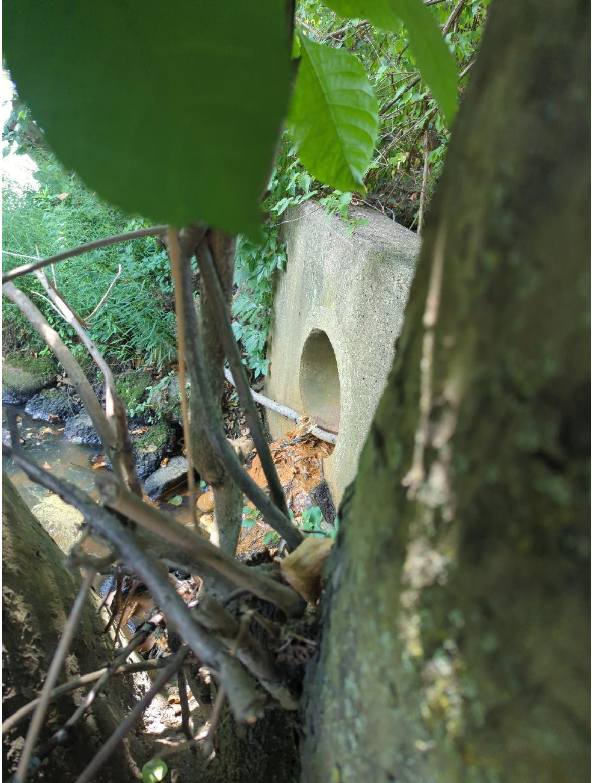
Outfall ID: AC14 (7/22/2022)
